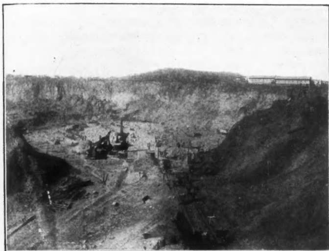
FACE OF NO. 1 WORKINGS
