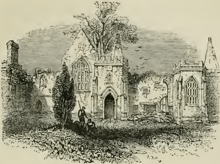
Remains of Winfield Manor House.
