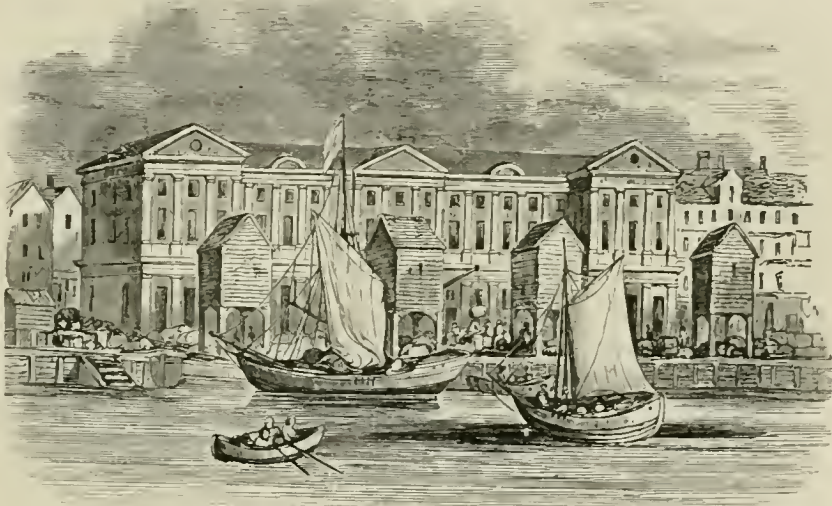
The Custom-House, London, as it appeared before the Great Fire. (From a Print by Hollar.)
