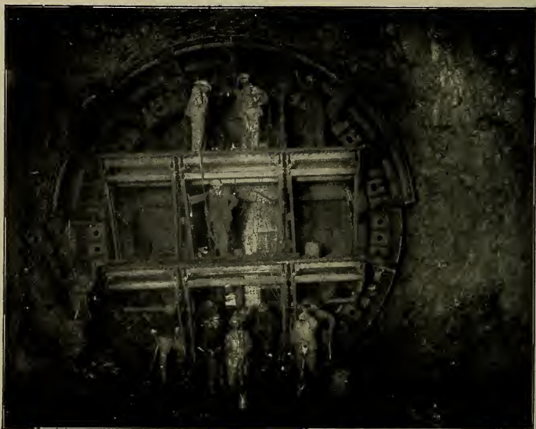
Shield Fitted with Fixed Hoods and Fixed Extensions to the Floors.
