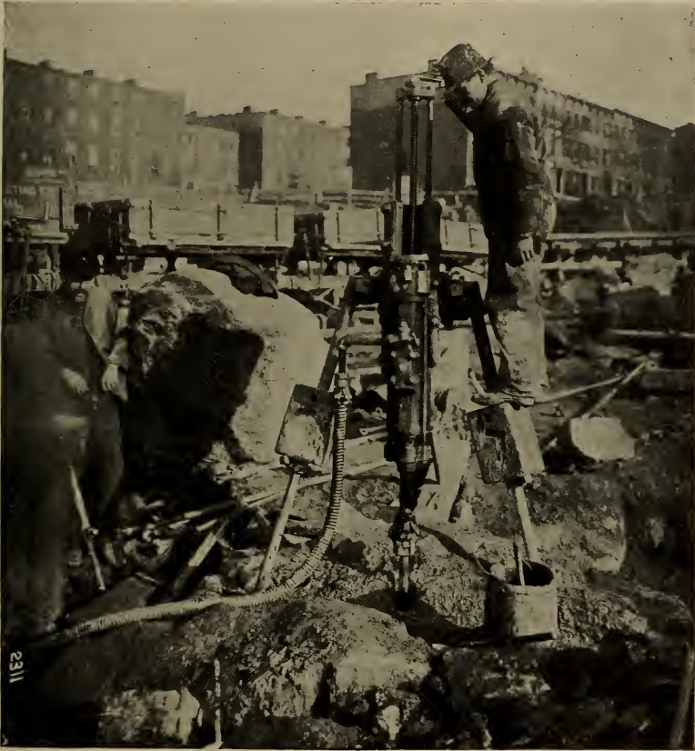
Drilling for P. R. R. Terminal Excavation.
