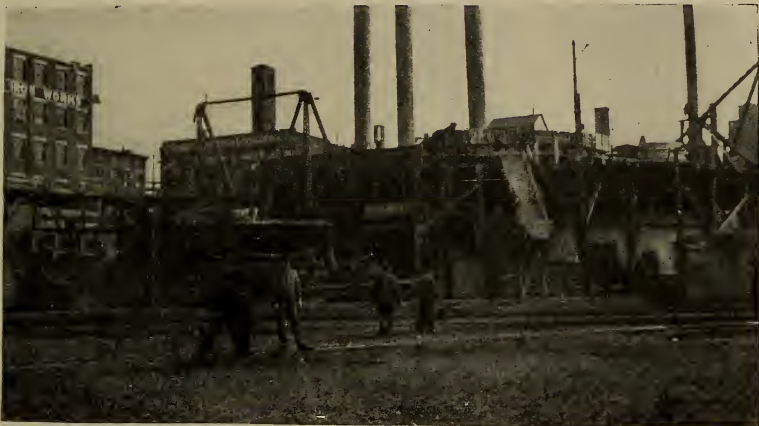
FIG. 7.—Manhattan Power House for P.R.R. North River Tunnels.
