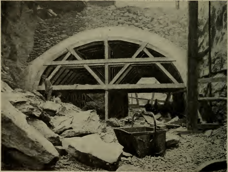
Concrete Arch Subway Construction in Open Cut.
