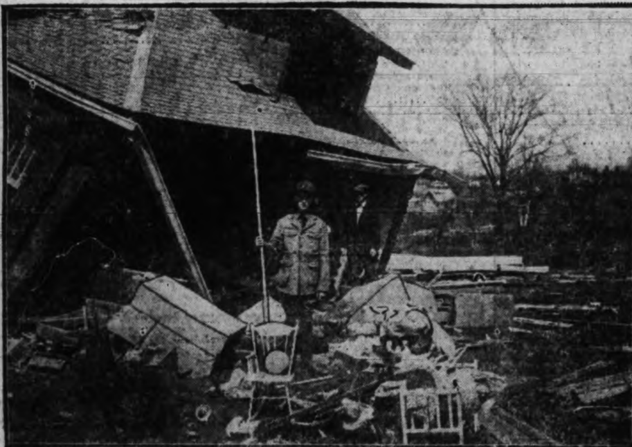
TWELVE BUILDINGS WERE COMPLETELY DESTROYED and a number injured in a tornado which recently swept the little town of Silver Springs, Md.
