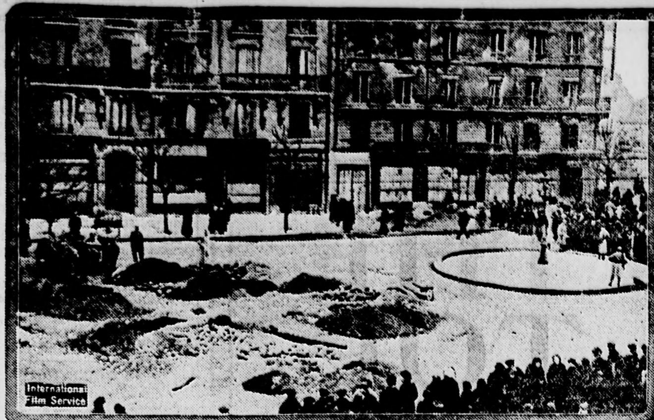
One of the streets in Paris showing the damage caused by a 200-pound torpedo dropped from a raiding Gotha on the night of January 30. Great holes many feet deep were made by the torpedoes, and the buildings in the background were badly injured.
