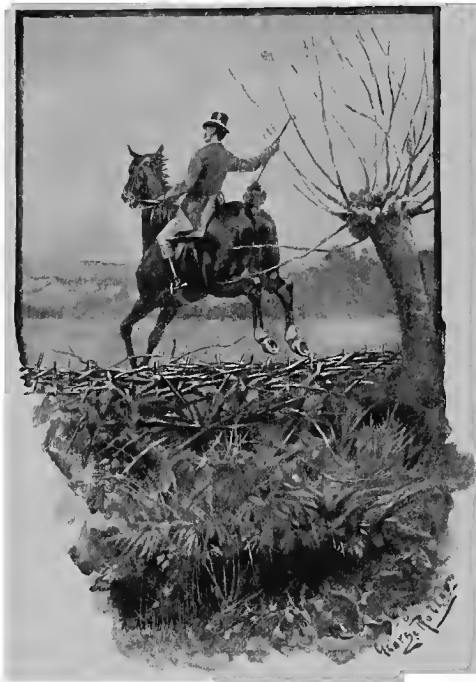
DITCH AND "STAKED-AND-BOUND" FENCE
