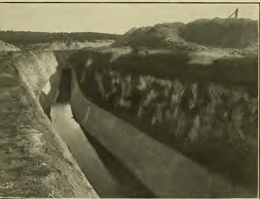
2. CONCRETE-LINED CANAL AND TUNNEL TAKING WATER FROM UPPER KLAMATH LAKE, OREGON.
