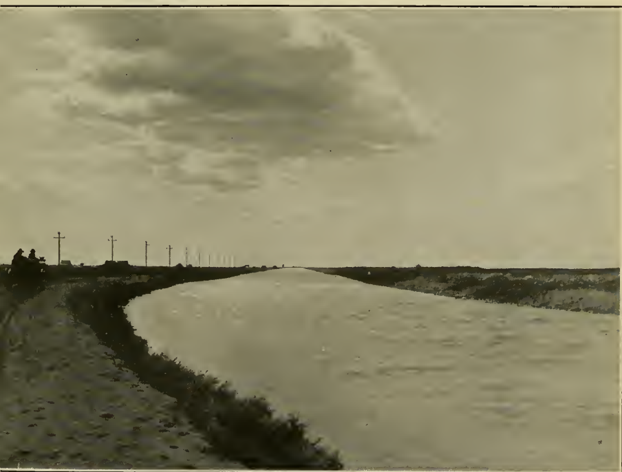
2. MAIN NORTHSIDE CANAL, MINIDOKA PROJECT, IDAHO, TYPICAL OF THE LARGER IRRIGATION CANALS, WITH POWER TRANSMISSION LINES LOCATED ON THE BANK.
