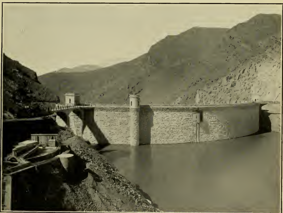
2. ROOSEVELT DAM, LOOKING DOWNSTREAM.
