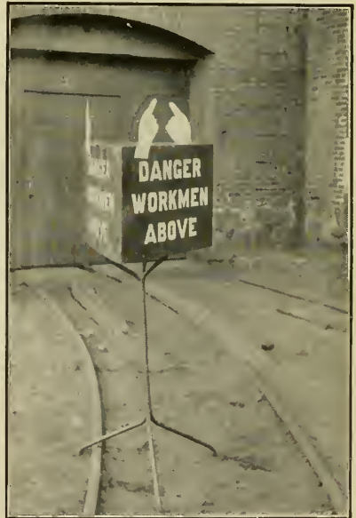
3. WARNING SIGN TO ATTRACT ATTENTION TO WORKMEN OVERHEAD.
