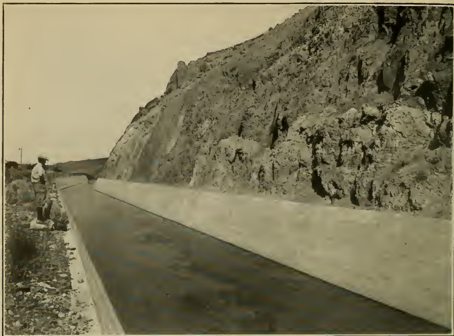
1. CEMENT-LINED CANAL CARRYING WATER OF TRUCKEE RIVER TO CARSON RIVER, NEVADA.
