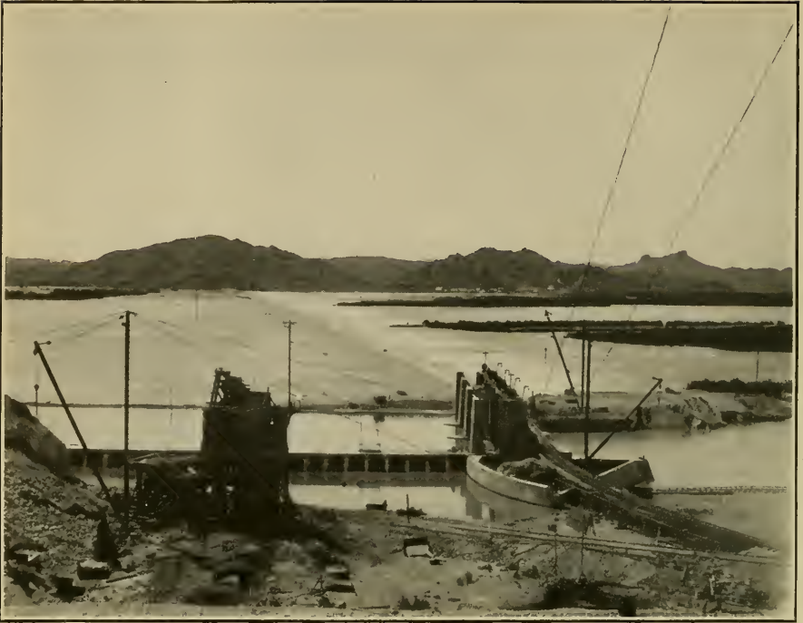
1. LAGUNA DAM ON COLORADO RIVER, LOOKING FROM NEAR THE HEADGATES ON THE CALIFORNIA SIDE ALONG THE AXIS OF THE DAM TO ARIZONA.
