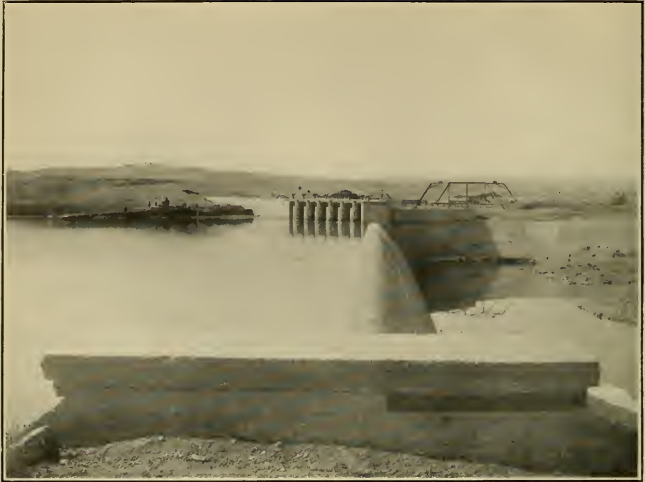
1. DAM IN BELLE FOURCHE RIVER, DIVERTING THE STREAM INTO FEED CANAL FOR OWL CREEK RESERVOIR, SOUTH DAKOTA.
