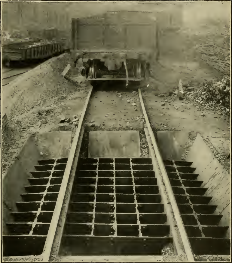
GRILL WORK PROTECTION FOR BINS AND HOPPERS.
