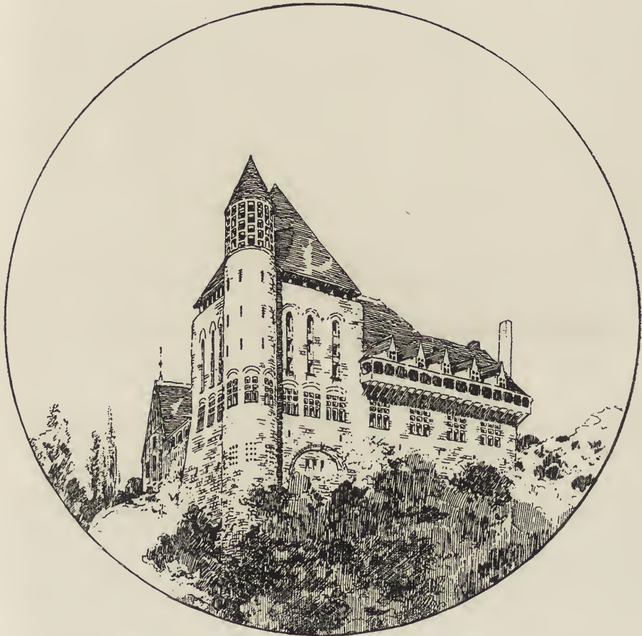
134. Design for Soldiers' Home, Minneapolis, Minn. L. S. Eufington, Architect. Grouping of windows. Triplet windows in mass. Four windows in appendage.
