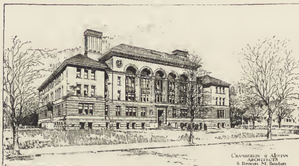
116. English High School, Cambridge, Mass. Mass with two appendages all roofed alike.
