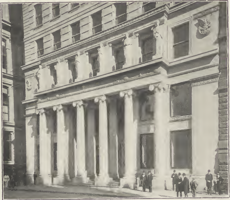
PORTICO OF THE AMERICAN SURETY BUILDING.
