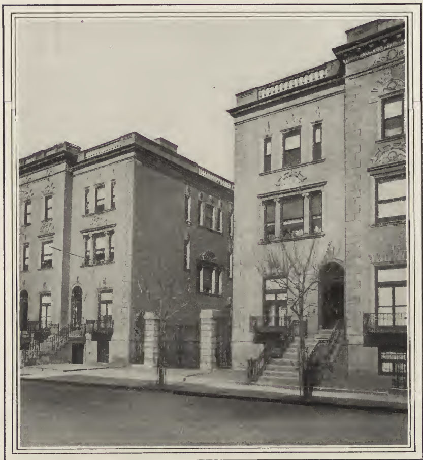
NOS. 219 AND 221 WEST 138TH STREET.
