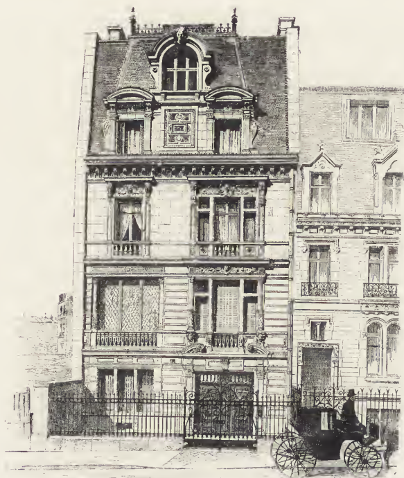
301. Example for critical analysis. Faulty composition of details.
