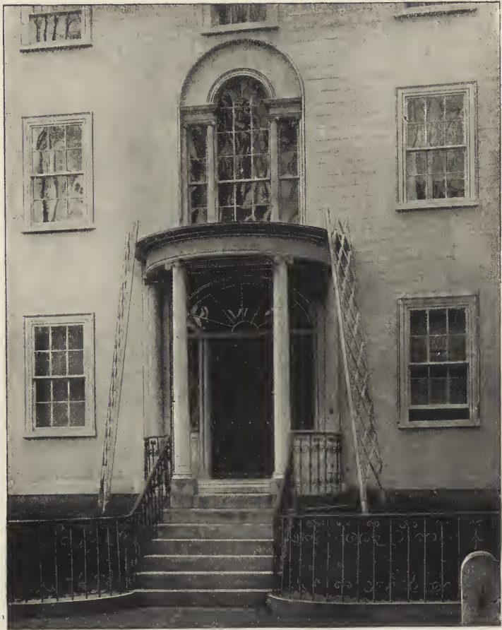
14 Middle Street, OLD COLONIAL DOORWAY, Portsmouth, N. H.
