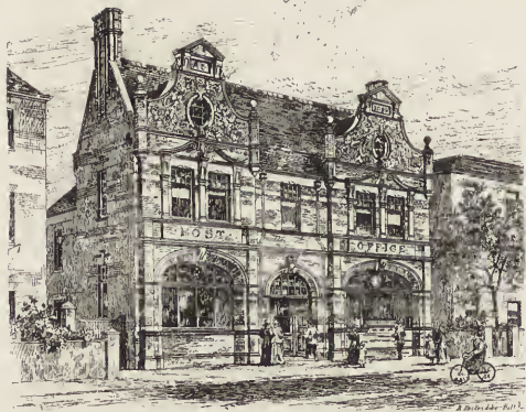
276. Postoffice, Surbiton, England. The central doorway serves to unite the double treatment.
