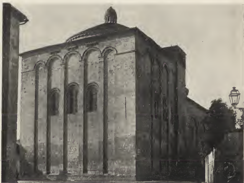
S. ÉTIENNE, PÉRIGUEUX. (From the northeast.)
