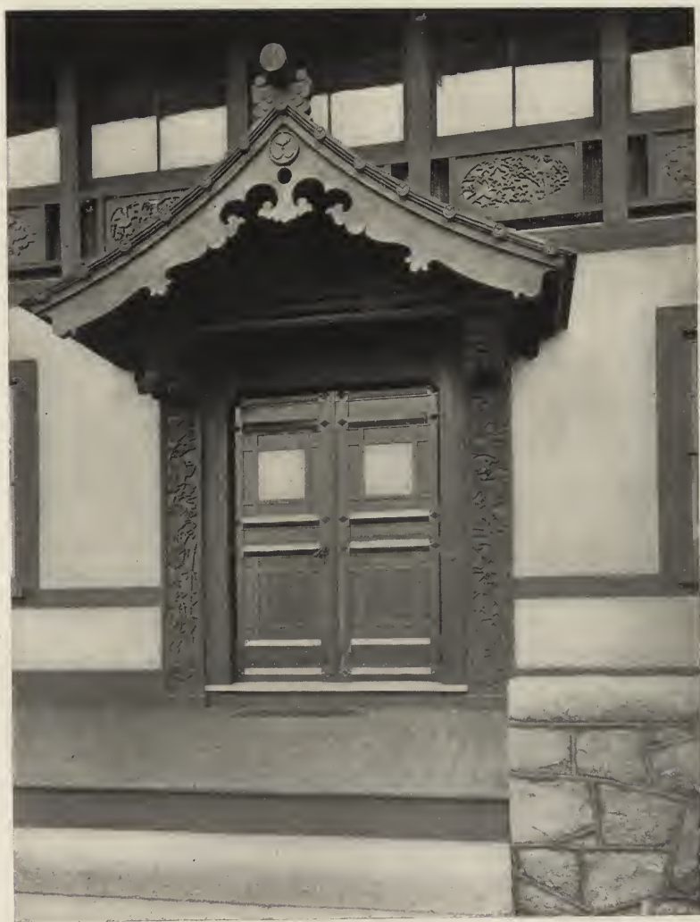
DETAIL OF THE FRONT DOOR.
