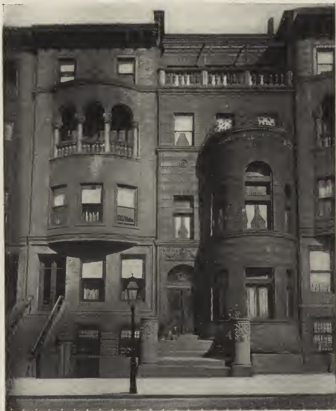
NOS. 327 AND 329 WEST 76TH STREET.
