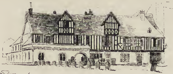
47. Old building at Lisieux. A single mass with two subordinate masses, so classed because one or both may be removed, yet leave a complete design.
