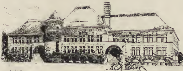
94. Pillsbury Science Hall, Minneapolis. L. S. Buffington, Architect. The high central part is the main mass. The tower is an unsymmetrical subordinate mass. The wings are two appendages.
