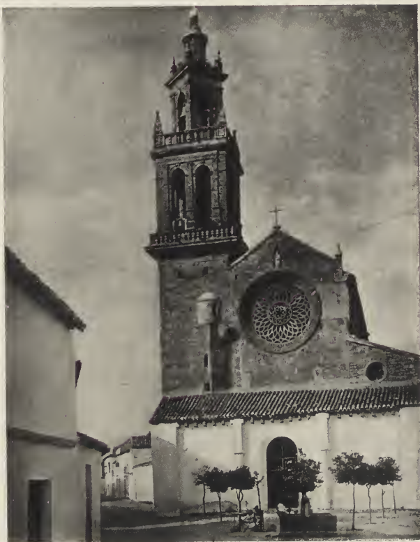
63. A single tower placed unsymmetrically.
