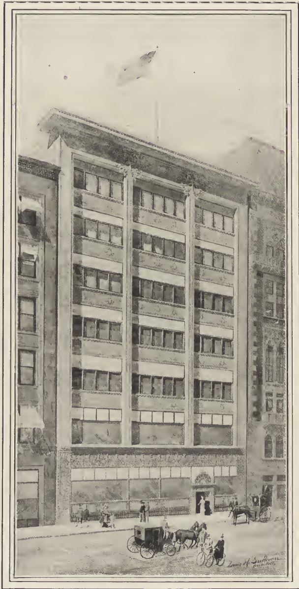
McCORMICK BUILDING. 130 Michigan Avenue, Chicago, Ill. Louis H. Sullivan, Architect.
