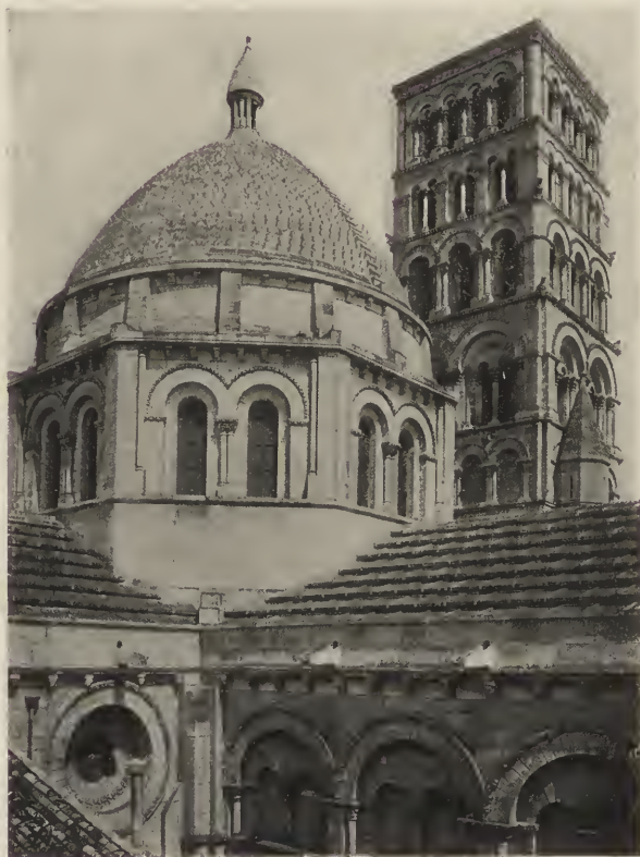
ANGOULÊME CATHEDRAL.—VIEW OF DOME AND TOWER.
