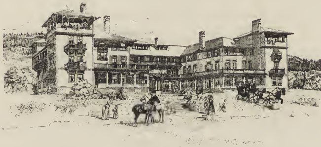
258. Another complex double group. Each member has a tower attached as a subordinate mass.
