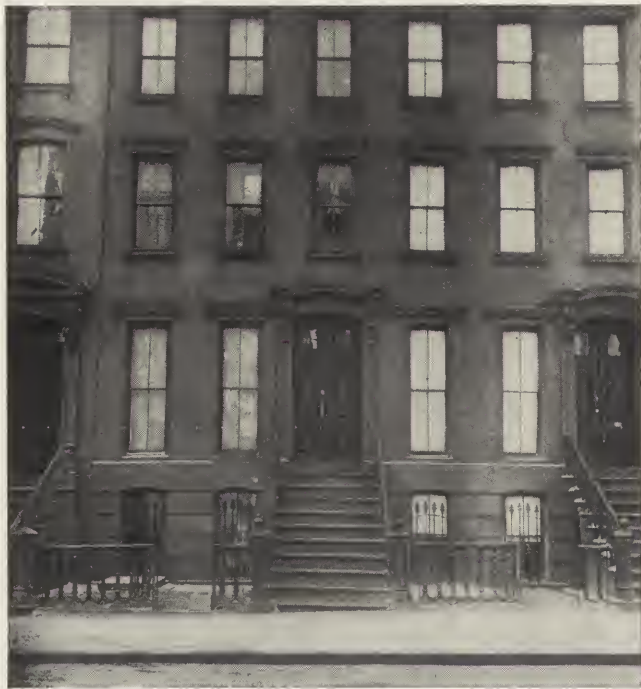
NO. 238 EAST 51ST STREET.
