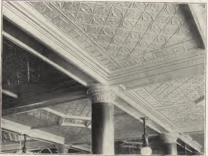
CEILING IN E. S. SMITH BUILDING, WASHINGTON, D. C.
