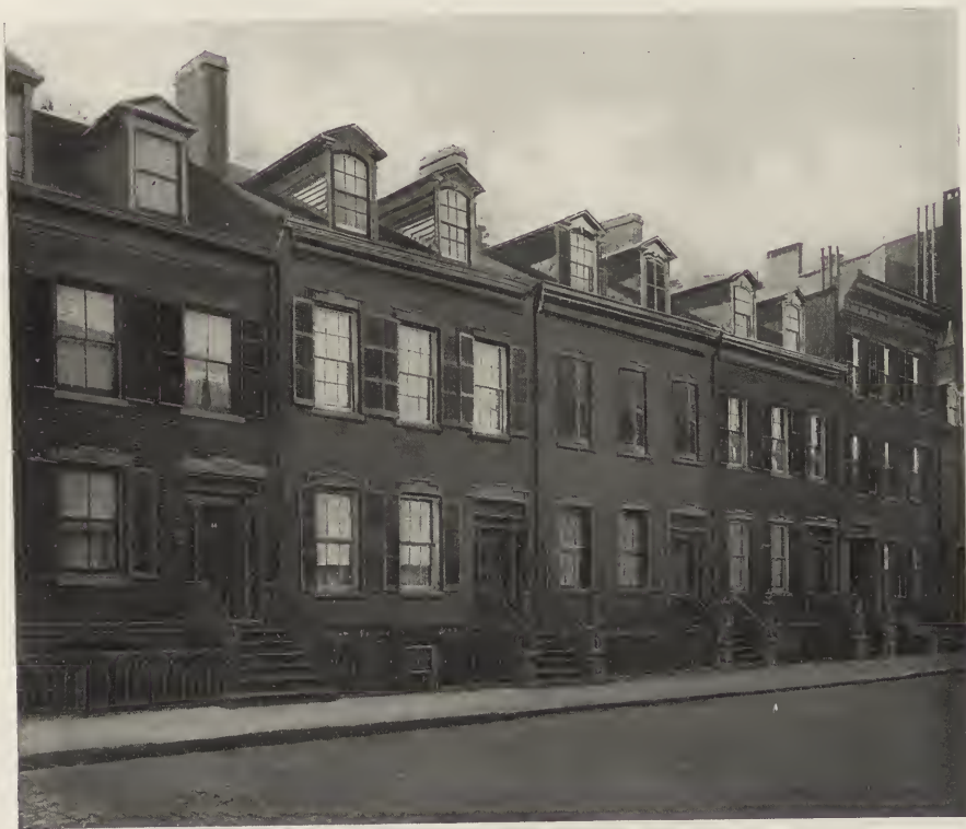
NOS. 16 TO 20 VANDAM STREET.
