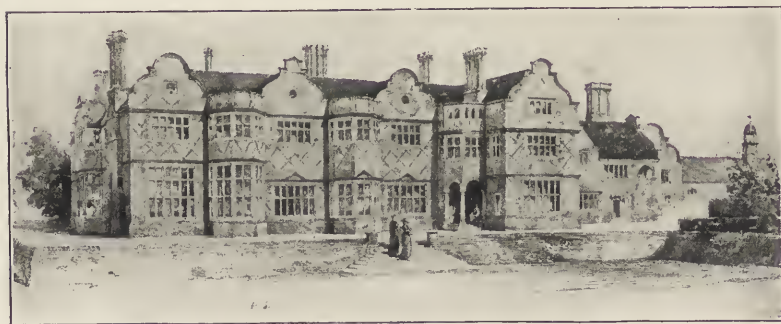
81. The same. The projection of one gable does not prevent its grouping with the others. There is also a group of three bays between the gables.
