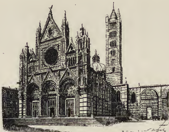
77. Cathedral, Sienna. The façade is an example of three unequal gables.
