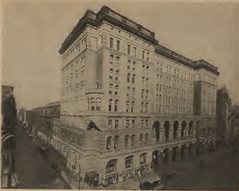
The Philadelphia & Reading Terminal Railroad Station, Philadelphia. Painted with Dixon's Silica Graphite Paint.
