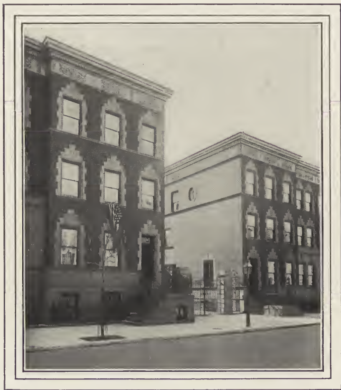
NOS. 214 AND 216 WEST 138TH STREET.
