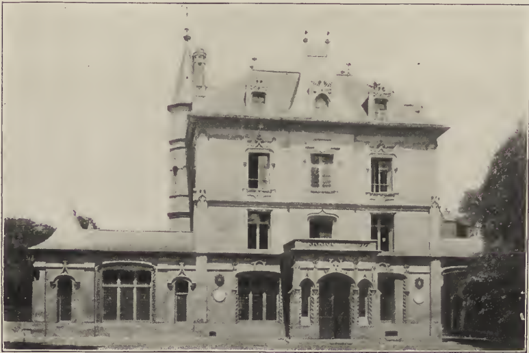
90. Mass, with a single appendage. The one-story portion on the left side is the appendage.
