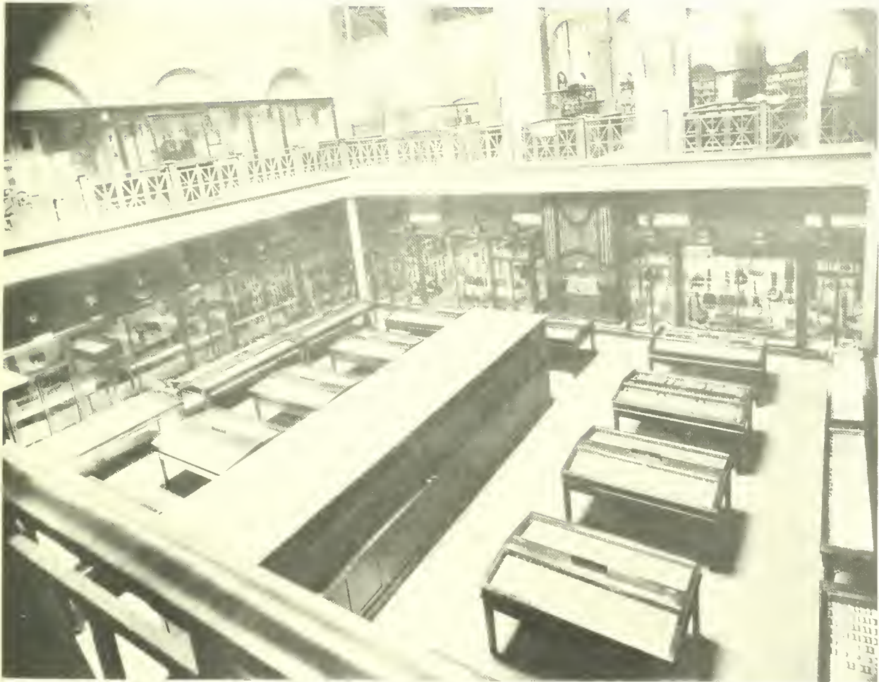
Fig. 128.—GENERAL VIEW of the northwest court in the Arts and Industries Building, about 1915.
