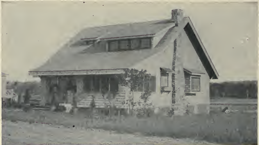
Brick piers are used here, with stone for the chimney. Whatever piers are used, latticework should close the openings between them
