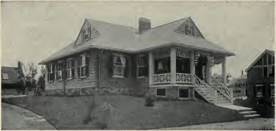
A continuous wall of stone has been used, with a raised line of pointing on the outside. The latter would be out of place with a less finished style of summer home
