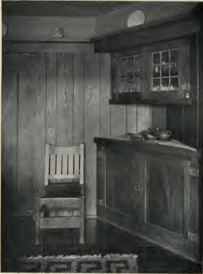
A high wainscoting of cypress in which six-inch and ten-inch boards are used alternately. The V-joint, as here, is always preferable to the beaded joint
