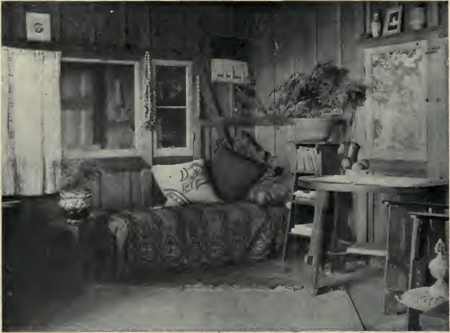
An inside finish of battened boards is used here, giving the effect of being set back so as to leave the studding frame slightly projecting
