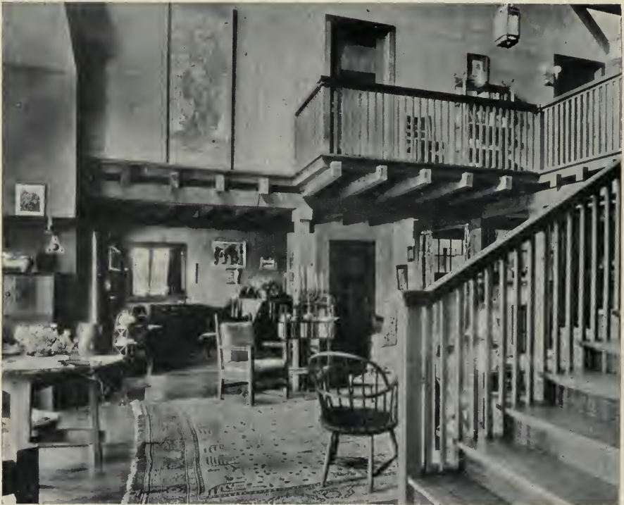
An interesting effect has been secured by leaving the floor joists uncovered to form the ceiling of the first story. The balcony is supported on these floor joists as cantilevers
