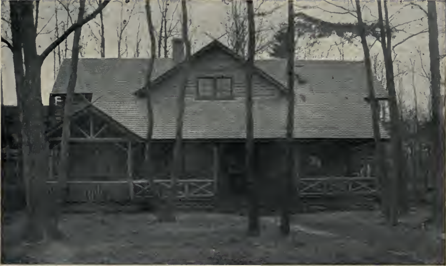
In this log structure the logs project one over another at the right-hand end to form a support for a balcony
