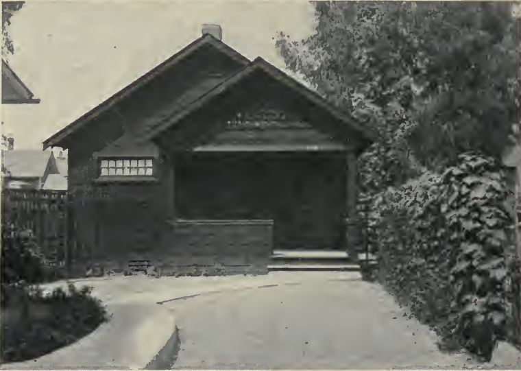
The side walls of shakes are carried directly down to the ground—a rather unusual form of foundation excepting in cheap construction. This whole bungalow cost but $1200. It consists of five rooms and a bath
