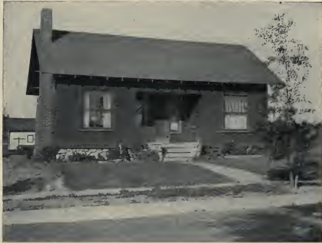
One of the very simple bungalows used as temporary homes in California—probably little more than a living-room and two bedrooms
