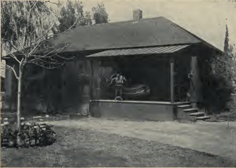
The foundation here is of rough redwood boards, set an inch or two apart with battens on the inside
