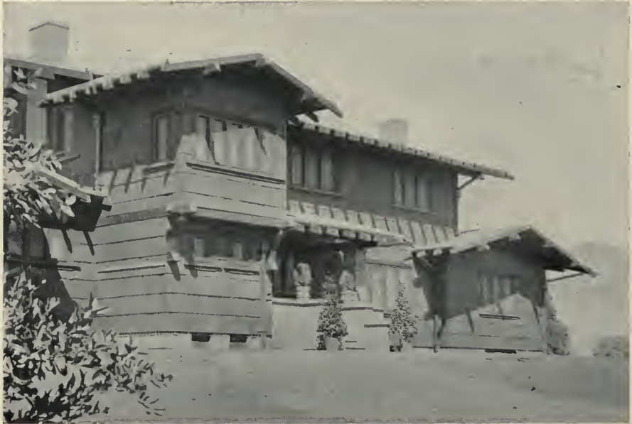
Other exteriors on pages 57, 115; interiors on pages 145, 151 Geo. A. Clark & L. du P. Millar, architects The roof of the Childs California home is covered with one of the prepared roofings that comes in a dull lead color
