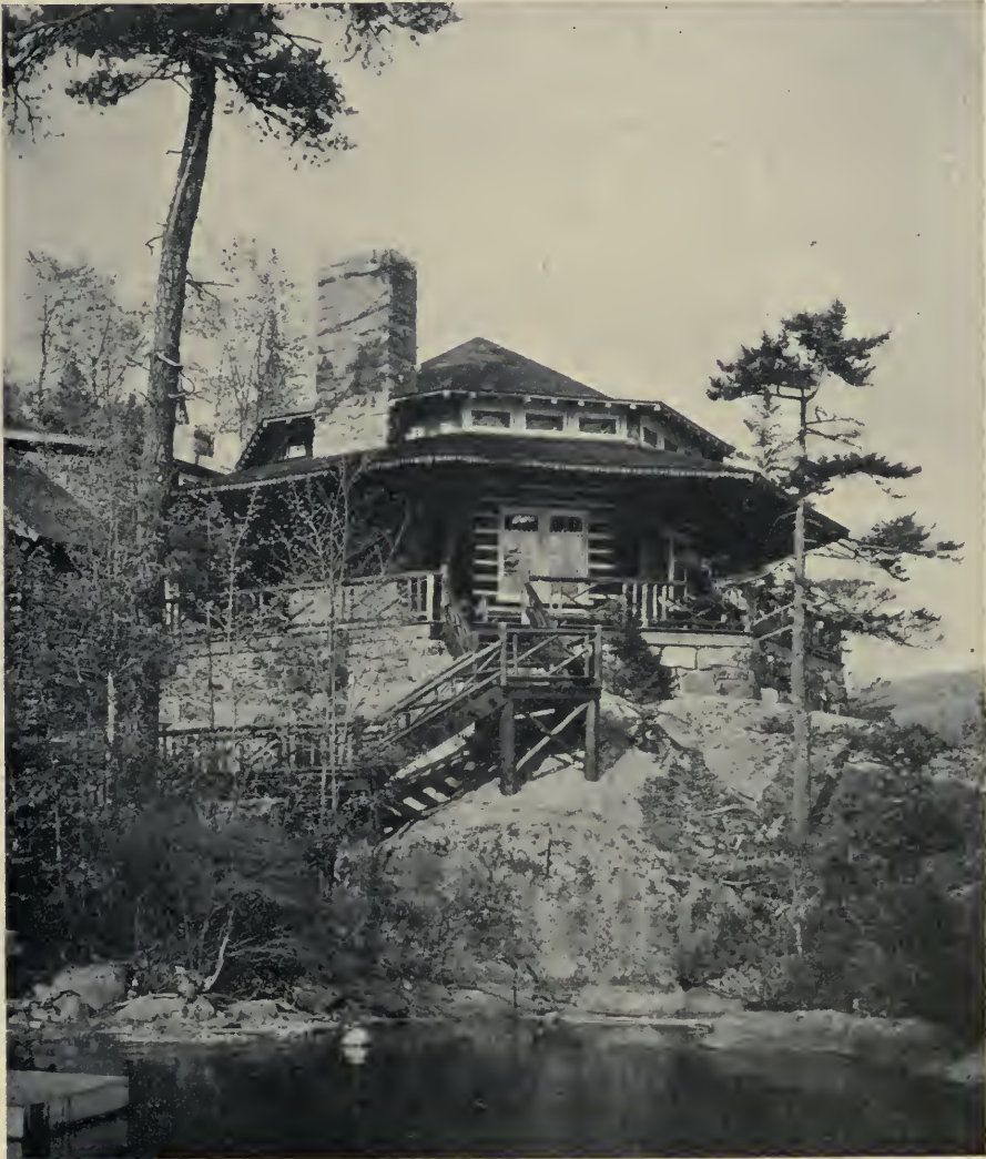
Exteriors pp. 39, 94, 100, 111, 153; interiors pp. 118, 148, 150, 152. Davis, McGrath & Shepard, architects The typical Adirondack lodge, this particular example being on Lake Wilbert, Franklin County, N. Y. The structure is of smooth logs with plastered chinks
