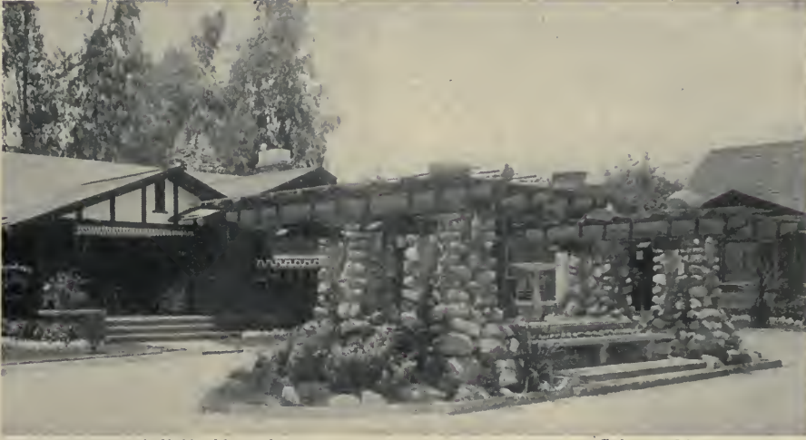
Plan on page 77; individual bungalows on pages 14, 21-25, 130, 142 Sylvanus Marston, architect At the near end of the Court the driveway turns around a fountain which is a very popular gathering place in the late afternoons
