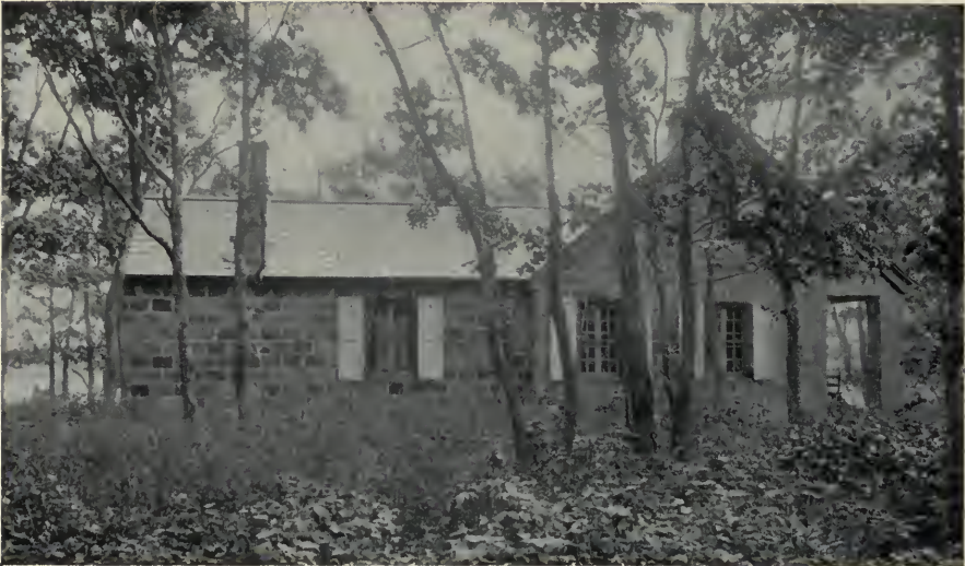
Other exterior on page 107; interiors on pages 131, 143, 167 Cummings & Howard, architects Terra cotta tile was used for the walls of this bungalow, being left uncovered both outside and in. The building is, of course, fireproof
