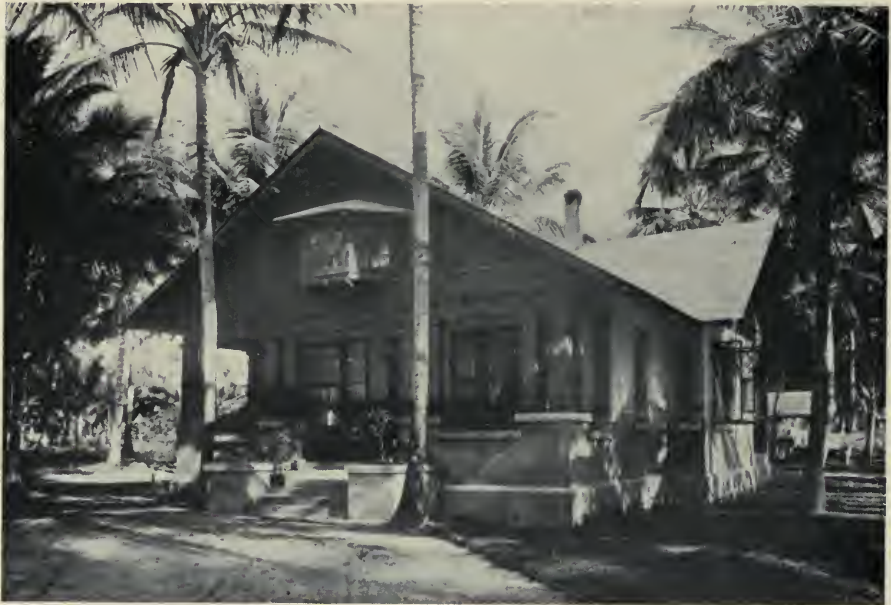
Antonin Nechodoma, architect The bungalow has found its way into the tropics, where the coolness of cement walls has naturally been found more agreeable than wood construction. Cement bungalows in Santa Domingo
