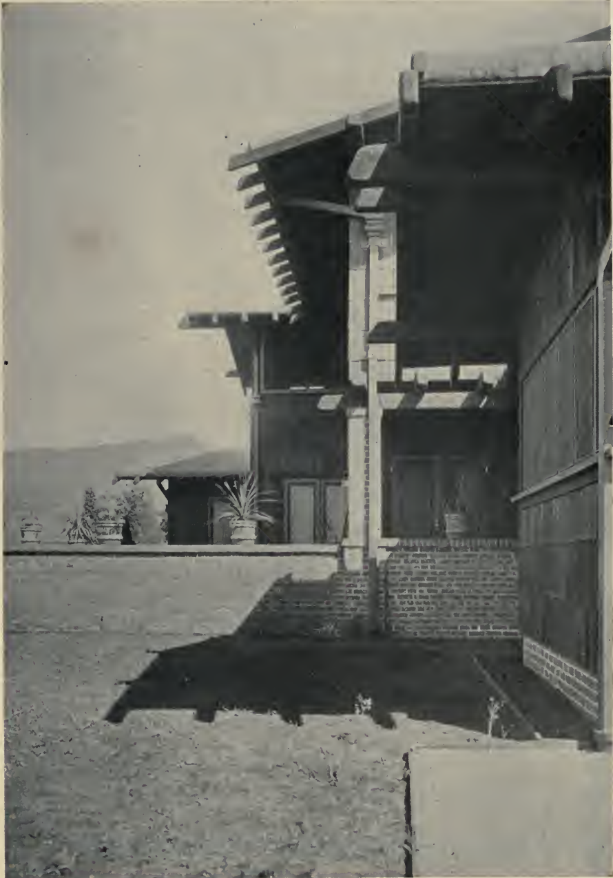
Other exteriors on pages 57, 114; interiors on pages 145, 151 Geo. A. Clark & L. du P. Millar, architects The roofing is turned over a rounded edge at the eaves in a way that gives it the appearance of a solid lead roof. The roof rafters inside are sheathed, the spaces between them being filled with sawdust to keep out the heat
