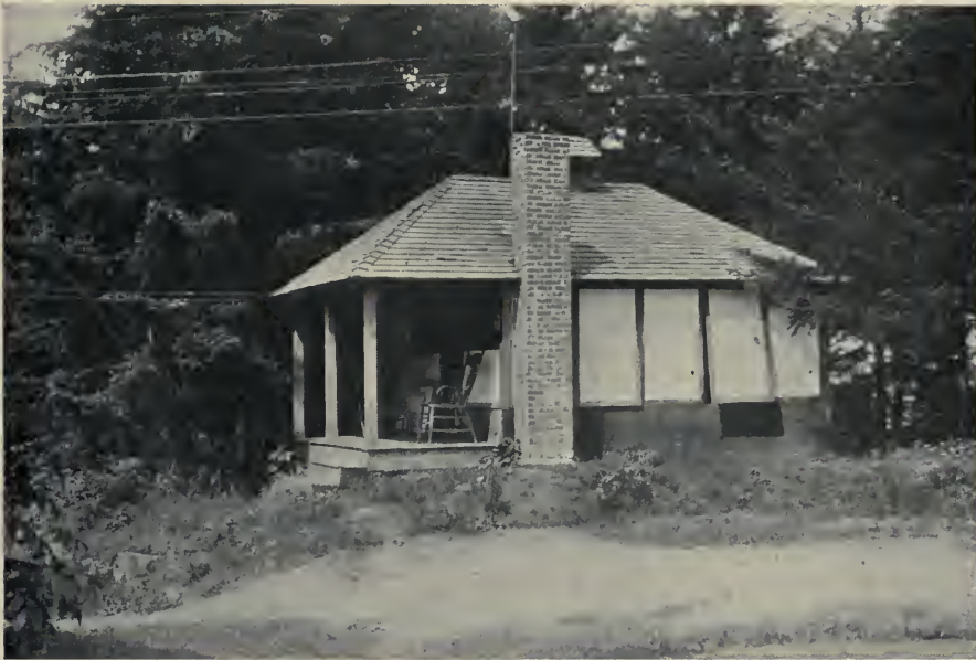
The tent-house of Southern California has the main portion of its side walls built of canvas stretched on frames. These may be propped open, giving shade and ventilation
