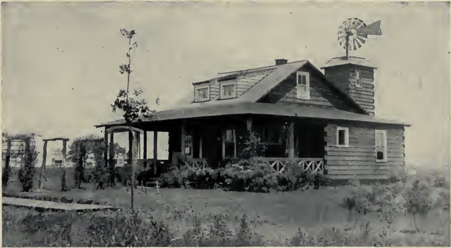
The windmill is usually passed over as a possibility for water supply on account of its unsightliness. In this example, however, the designer has incorporated it rather ingeniously with the design of the whole building
