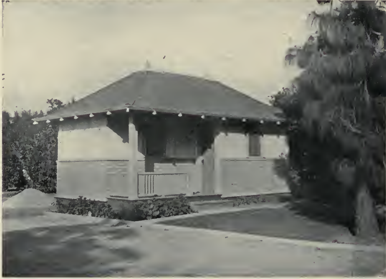
There are two rooms and a shower bath in this Southern California tent-house; the cost was about $300
