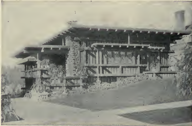
A Western Coast bungalow that displays a remarkably daring utilization of modified Japanese motives. The roof, it will be noticed, is almost flat. The walls are made up of whole timbers
