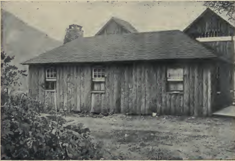
The best way to secure the effect of a log structure inexpensively is to nail slabs—the outside slices of a log—directly to a stud frame
