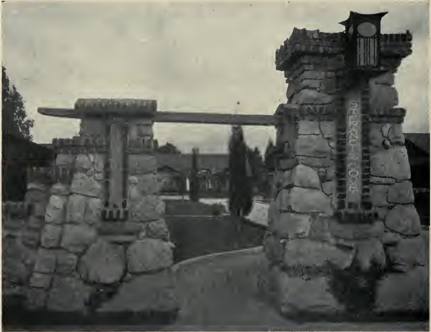
Plan on page 77; individual bungalows on pages 14, 21-25, 130, 142 Sylvanus Marston, architect The footpath entrance to St. Francis Court, Pasadena—a striking instance of the very common use throughout Southern California of rough clinker brick in conjunction with stone work
