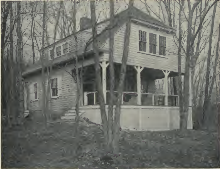
Plan on page 57; interiors on pages 80, 81, 136 William P. Hubon, architect Mr. Hubon's camp near Salem, is said to have been built at a cost of $1100, of shingles that have been allowed to weather
