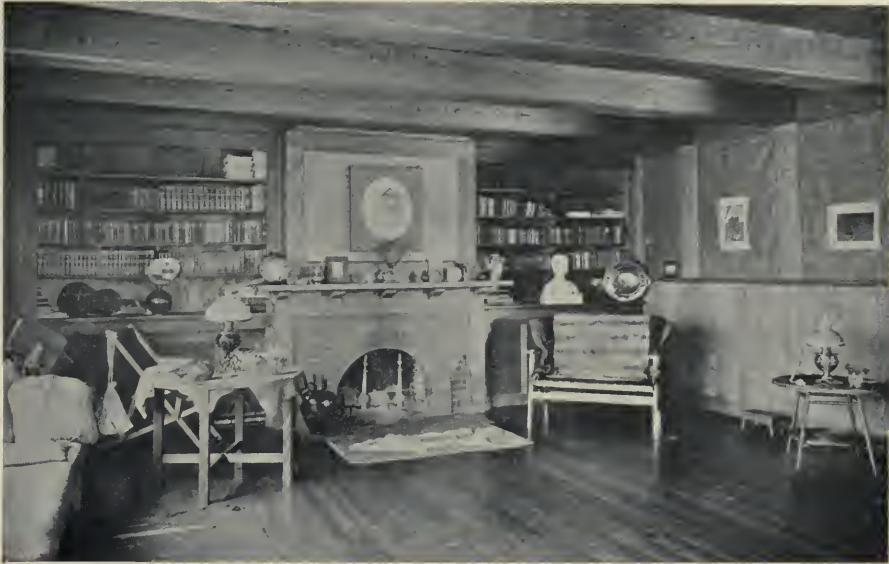
The walls are finished with a perfectly plain wainscoting of cypress, above which bur-lap is used between the upright strips under the boxed ceiling beams
