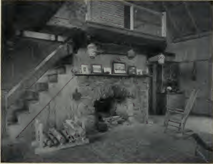
Plan on page 57; exterior on page 56; other interiors on pages 80, 81 William P. Hubon, architect Mr. Hubon has made a more effective feature of his stone fireplace by running the stairway to the attic up around its front
