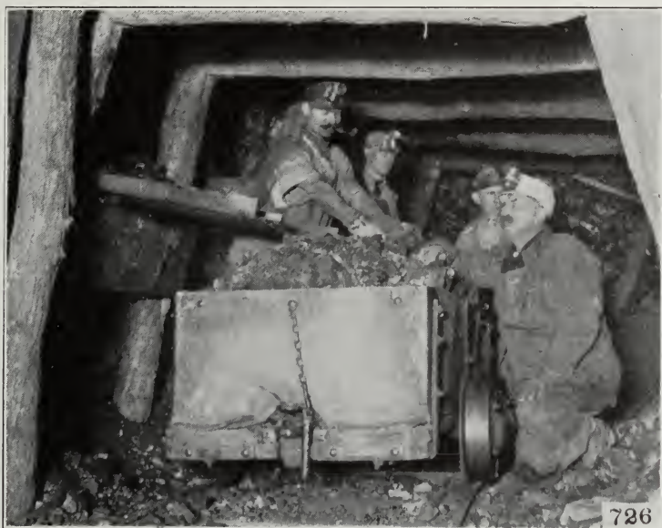
FIG. 26. Chute in panel longwall mine in dipping seam (photo by H. I. Smith, U. S. Bureau of Mines)
