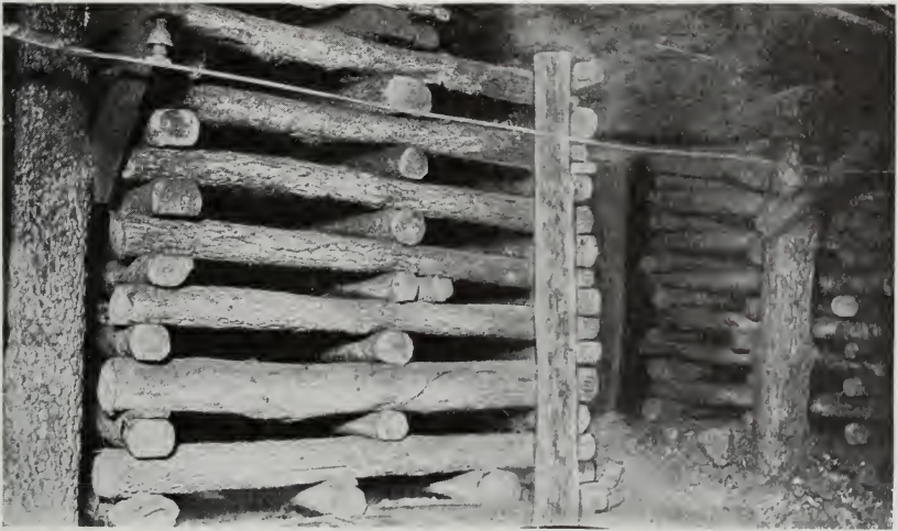
FIG. 41. Cog timbering at parting
