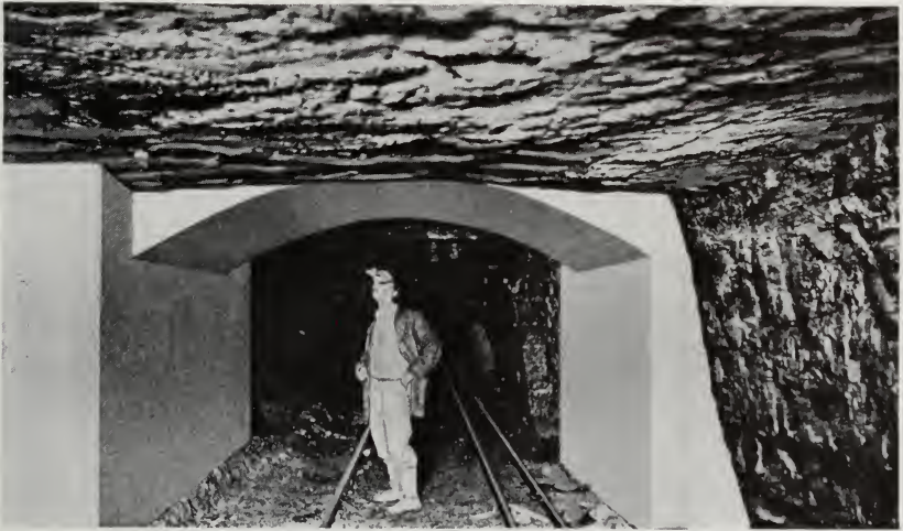
FIG. 53. Concrete overcast
