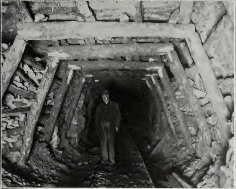
FIG. 36. Entry closely timbered in longwall mine
