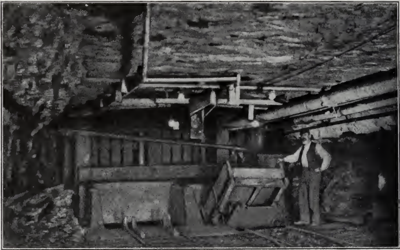
FIG. 60. Hopper for receiving coal at bottom of shaft
