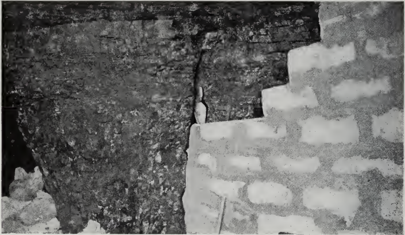
FIG. 50. Latch in rib dug to receive stopping
