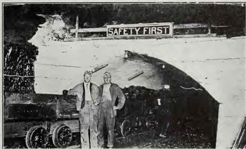
FIG. 39. Inby end of concrete-lined bottom
