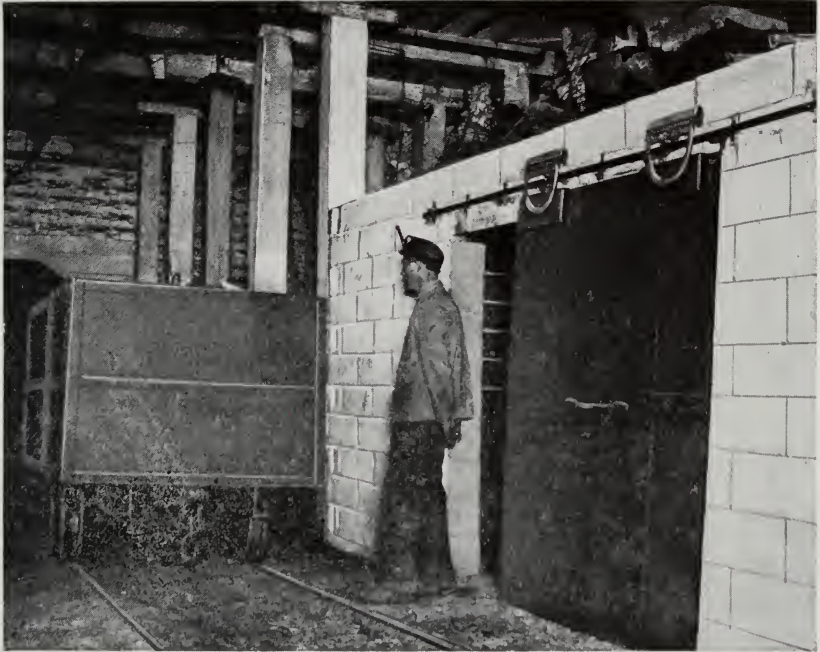
FIG. 54. Steel hay car and concrete hay room. (Photo by R. Y. Williams, U. S. Bureau of Mines.)
