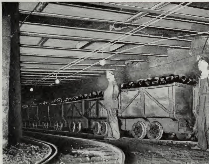
FIG. 38. Shaft bottom with roof supported by steel I-beams set on concrete walls (photo by R. Y. Williams, U. S. Bureau of Mines)
