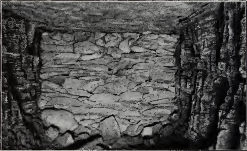
FIG. 48. Typical gob stopping
