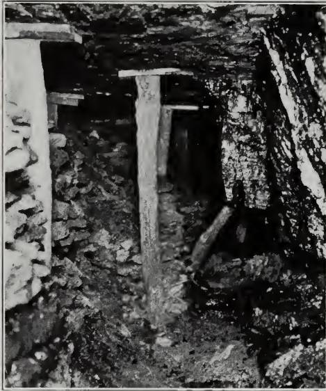
FIG. 27. Props and sprags at face of longwall mine (photo by H. I. Smith, U. S. Bureau of Mines)
