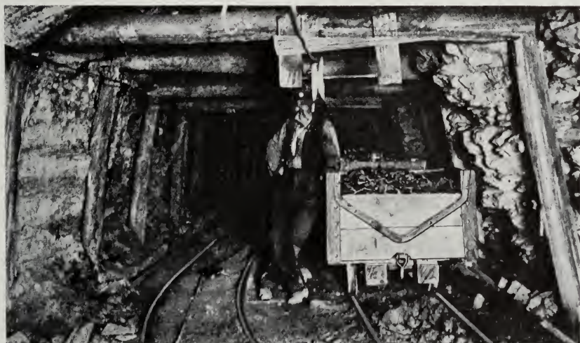
FIG. 37. A typical lye in a longwall mine
