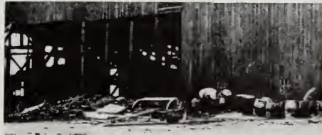
FIG. 65. Inflammable material piled against frame tipple
