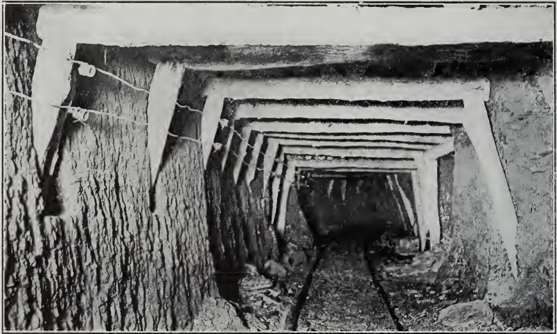
FIG. 42. Timbering in haulage entry
