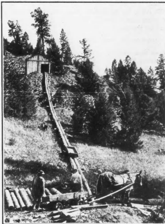
The higher adits are not conveniently reached by horse-drawn carts carrying the mine timbers, so this skidway has been built, up which the timbers are pulled by a compressed-air hoist
