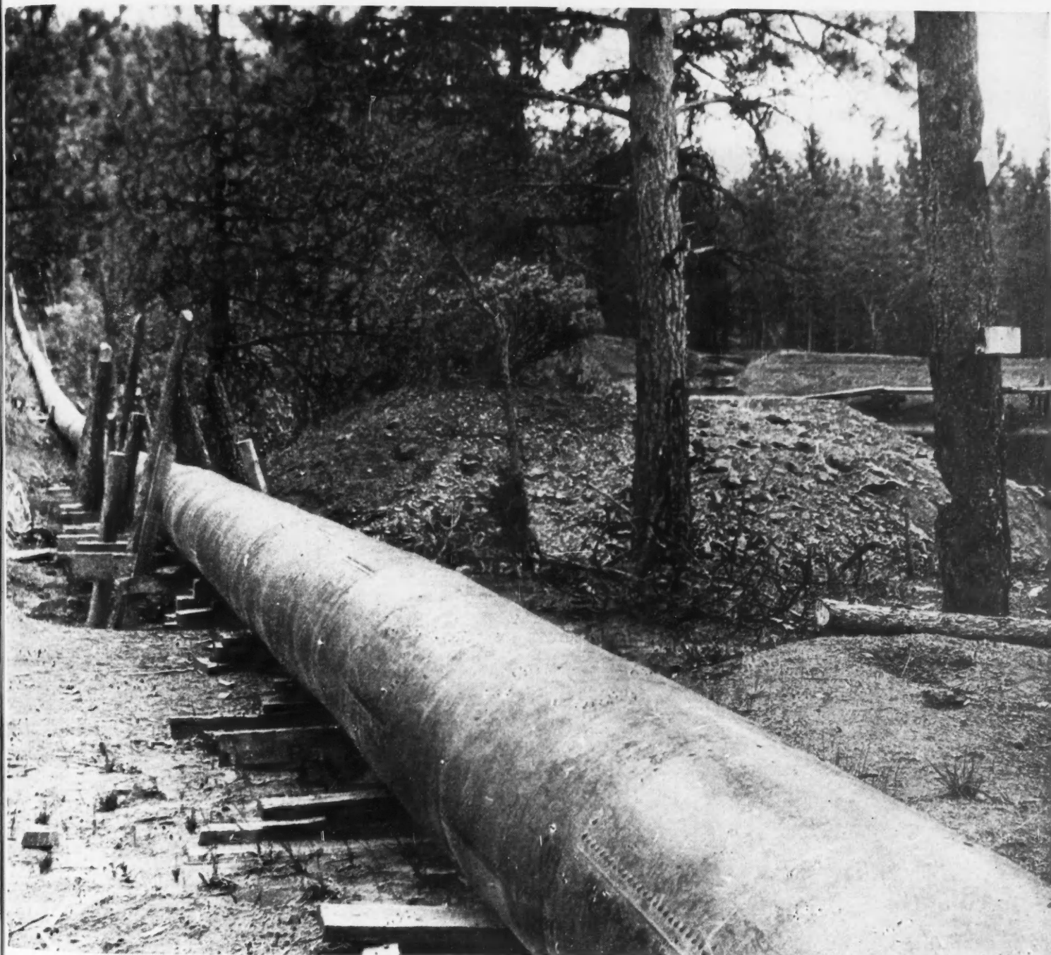
A pipe line in southern Oregon that supplies water for hydraulic mining gold-bearing gravels
