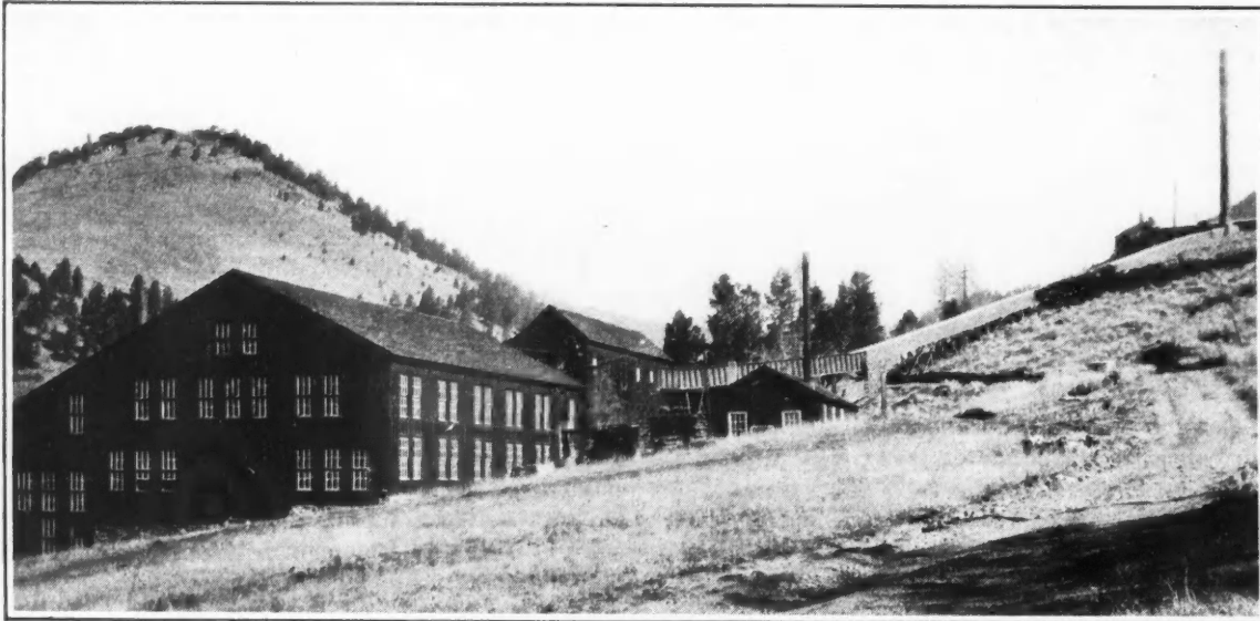
The concentrating mill and arsenic plant of the Jardine Mining Co. A wooden flue leads up the mountain side to the steel stack
