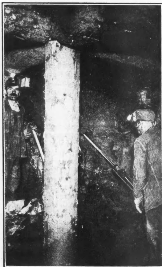
Meant to be a drilling scene underground, this flashlight is rather a photograph of one of the square sets so generally used in the mine
