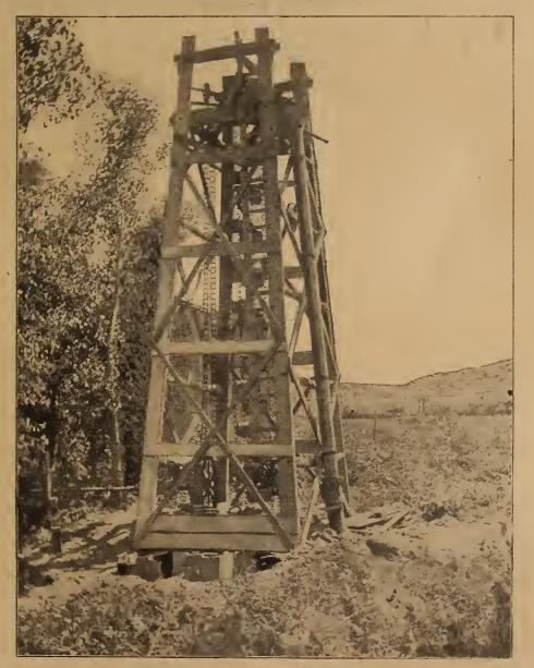
DERRICK WITH BUCKETS ON ENDLESS CHAIN ELEVATING WATER WHICH IS VALUED AT \$10 A DAY FOR IRRIGATING PURPOSES
