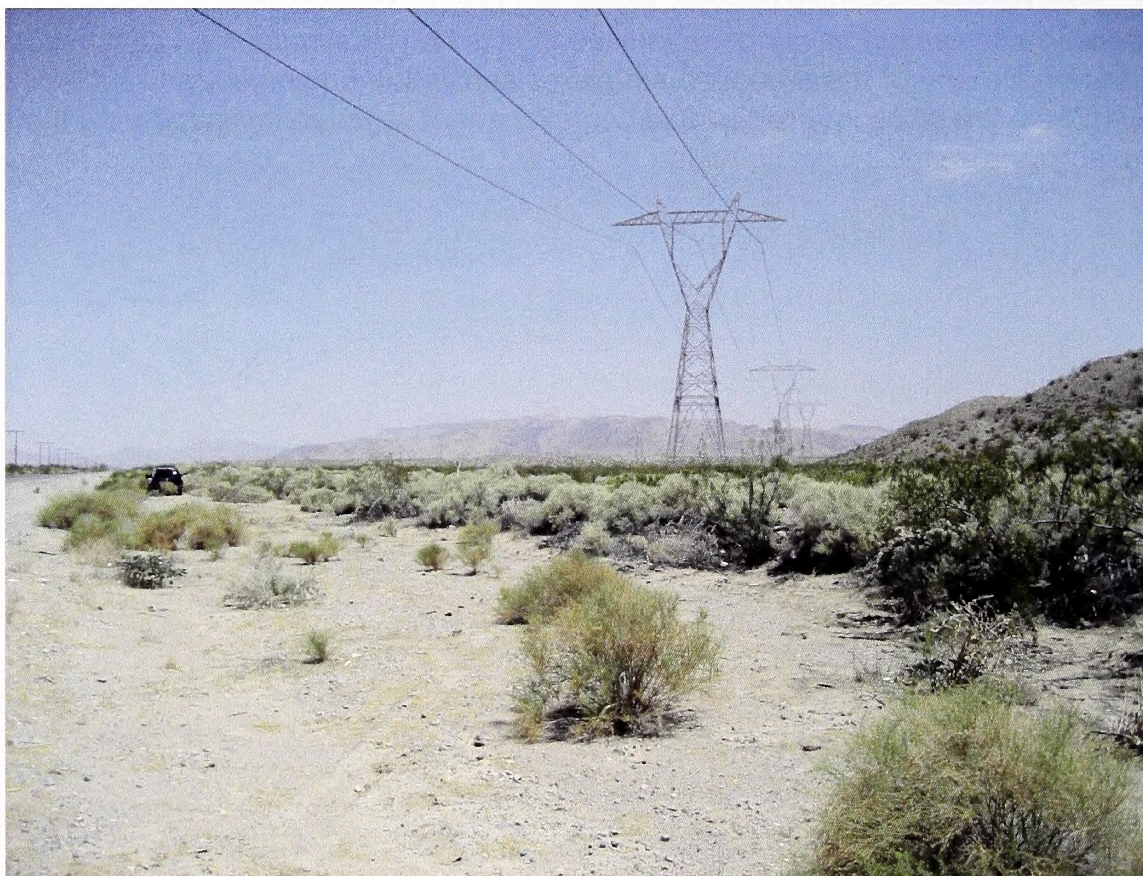
Figure 4.15-5 View to the North from KOP 4, Segment 10 Sub-Alternative
