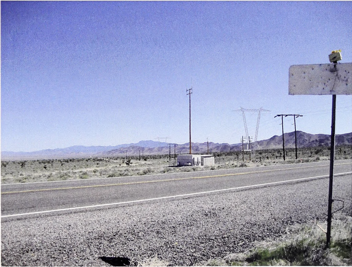
Figure 4.15-3 View to the Northeast from KOP 2, Segment 8, Guyed-V Structures
