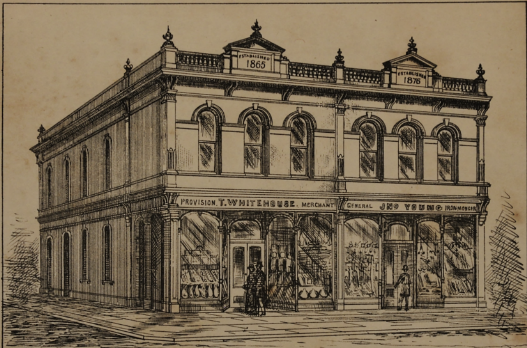
T. WHITEHOUSE - NEW BUILDING CUBA STREET
