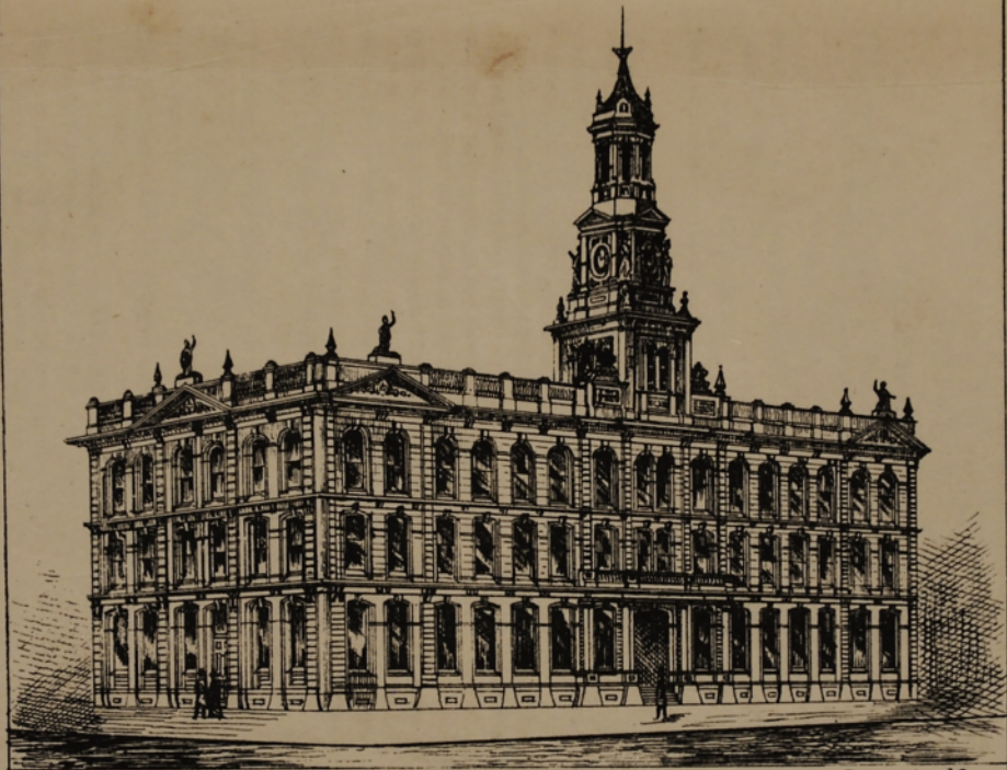
NEW POST AND TELEGRAPH OFFICES.
