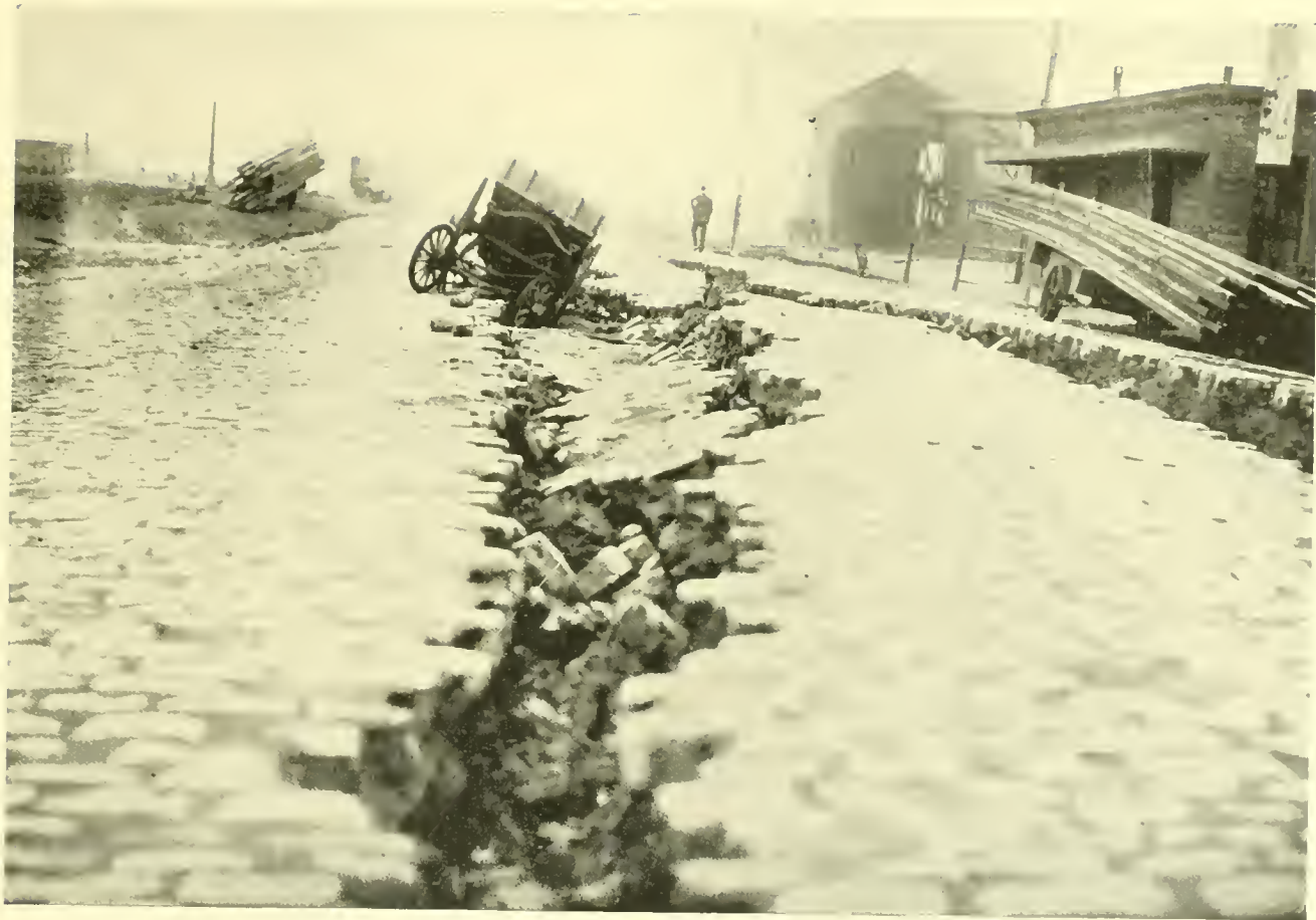
Break in the Street near Water Front, caused by Earthquake.
