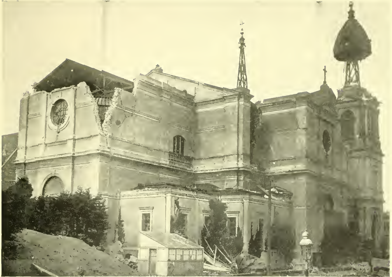
St. Dominic's Church, Bush and Steiner Streets—Wrecked by Earthquake.
