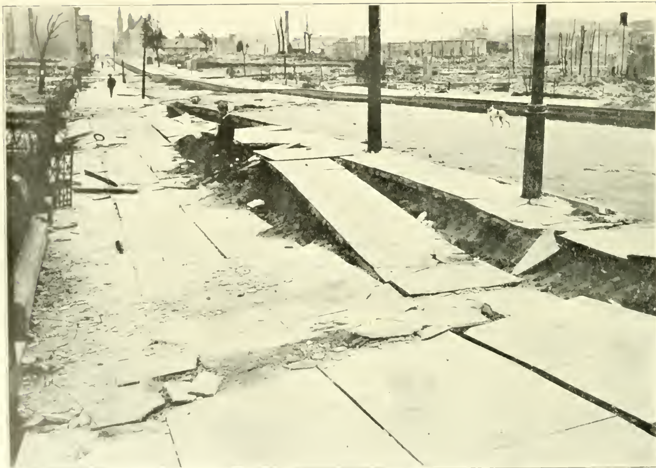
Capp Street, near Seventeenth, Damaged by Earthquake.
