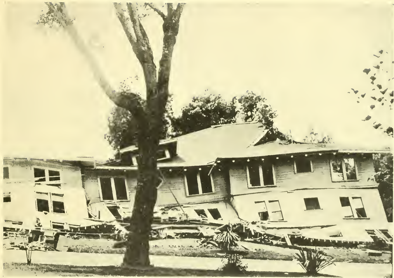
Hotel Vendome Annex, San Jose, Wrecked by Earthquake.
