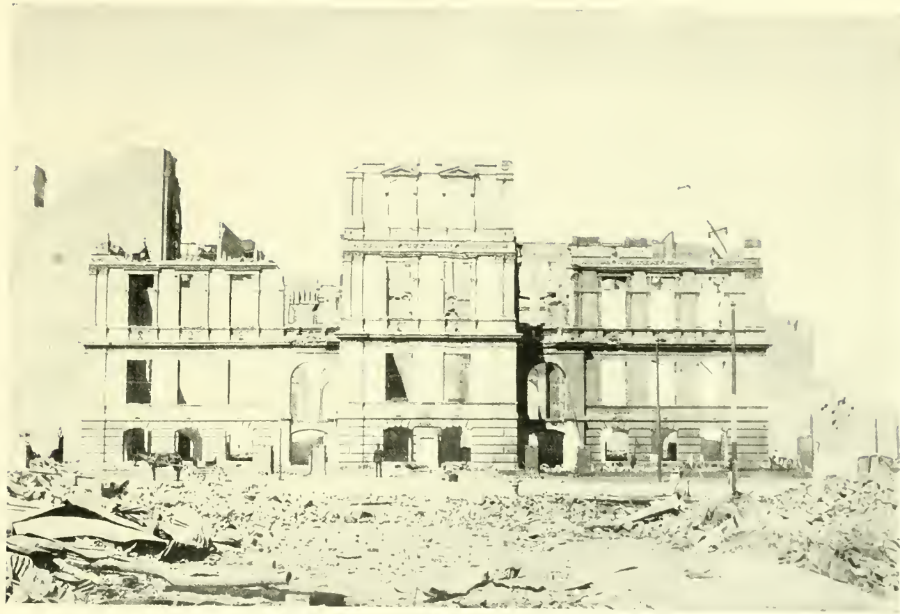
Lincoln School, Fifth Street. Damaged by Fire.
