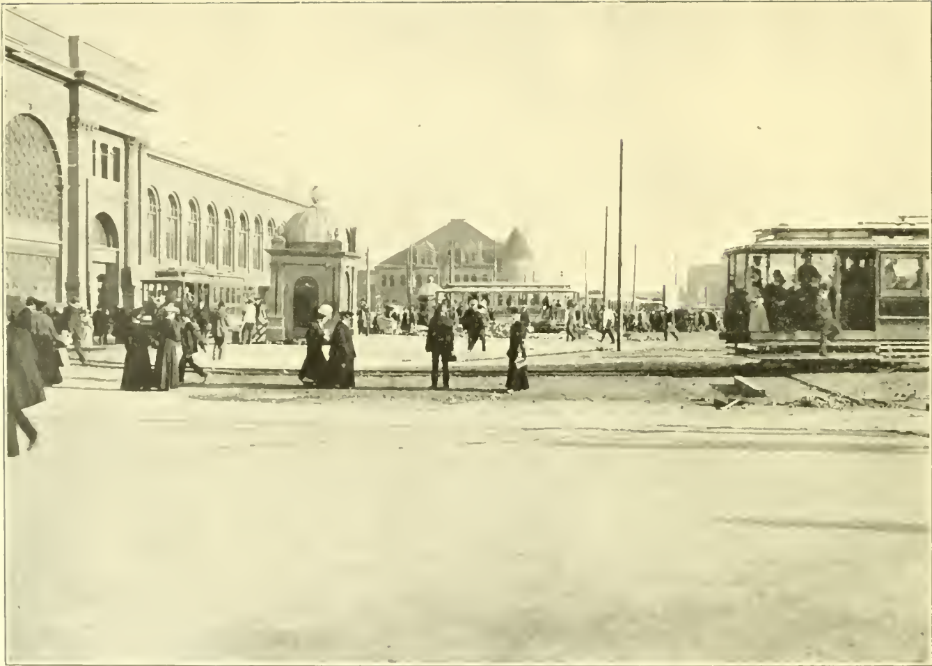
The New Loop at the Ferry for Car Service. Completed November, 1906.
