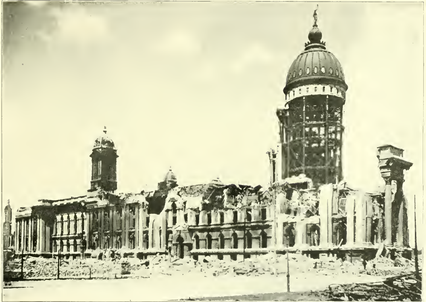
City Hall, San Francisco, Damaged by Earthquake.
