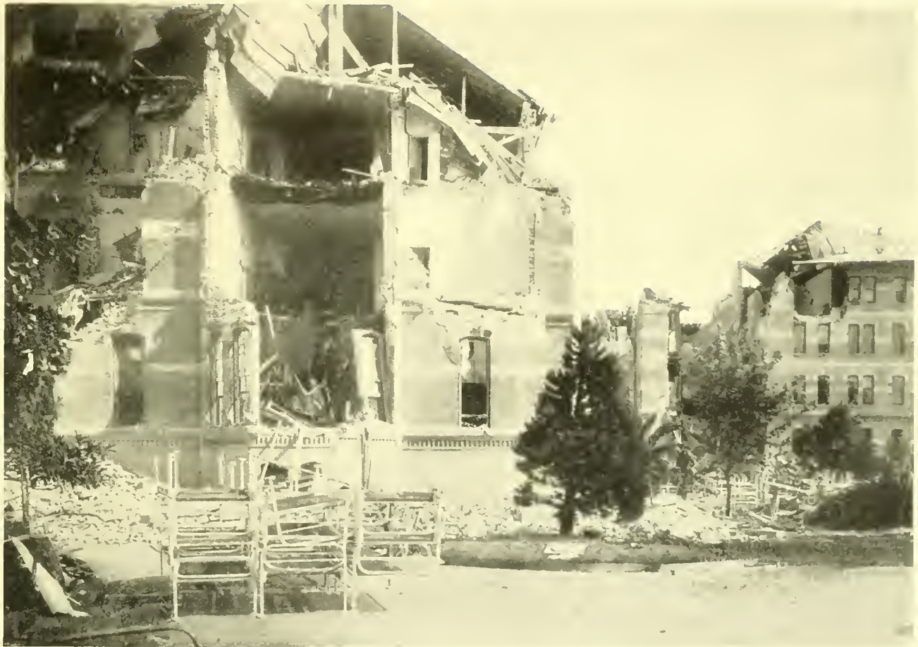
Another portion of the Wrecked Asylum at Agnews, showing Results of Earthquake.
