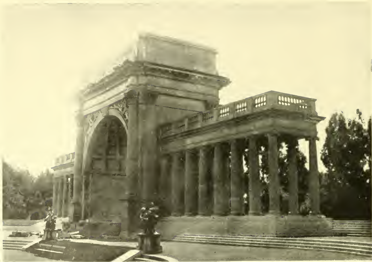
The Music Stand, Golden Gate Park, Damaged by Earthquake.
