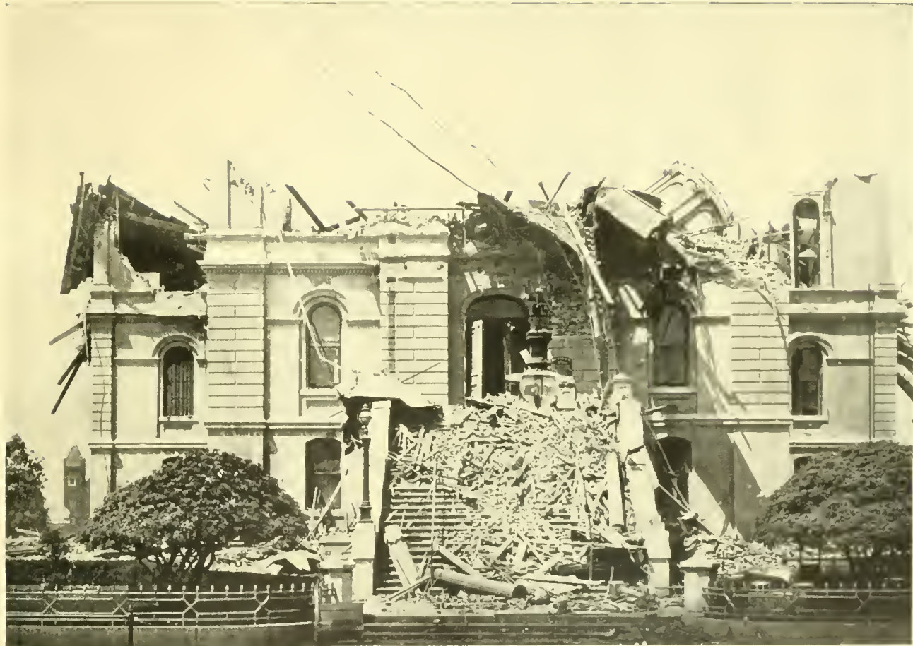
Sonoma County Courthouse, Santa Rosa, after the Earthquake.
