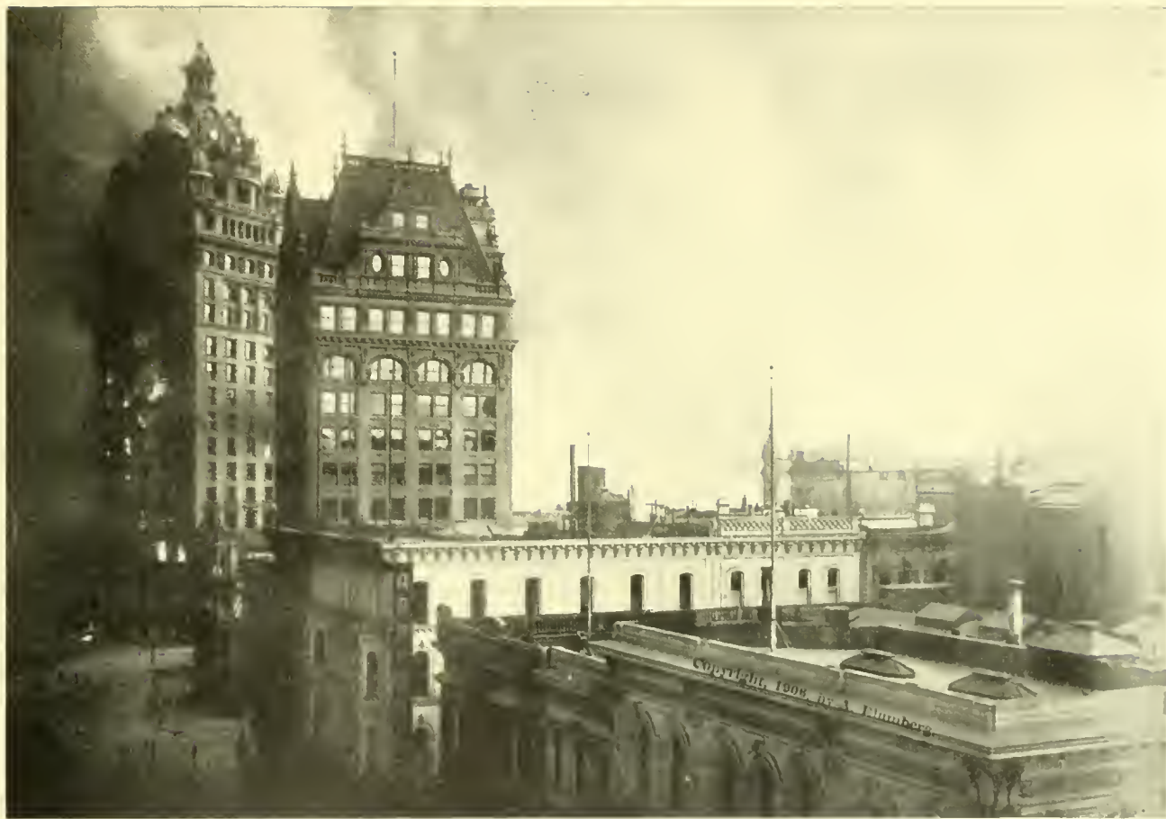
The Burning of the Call Building, as seen from Kearny Street. The Mutual Savings Bank Building in the foreground.
