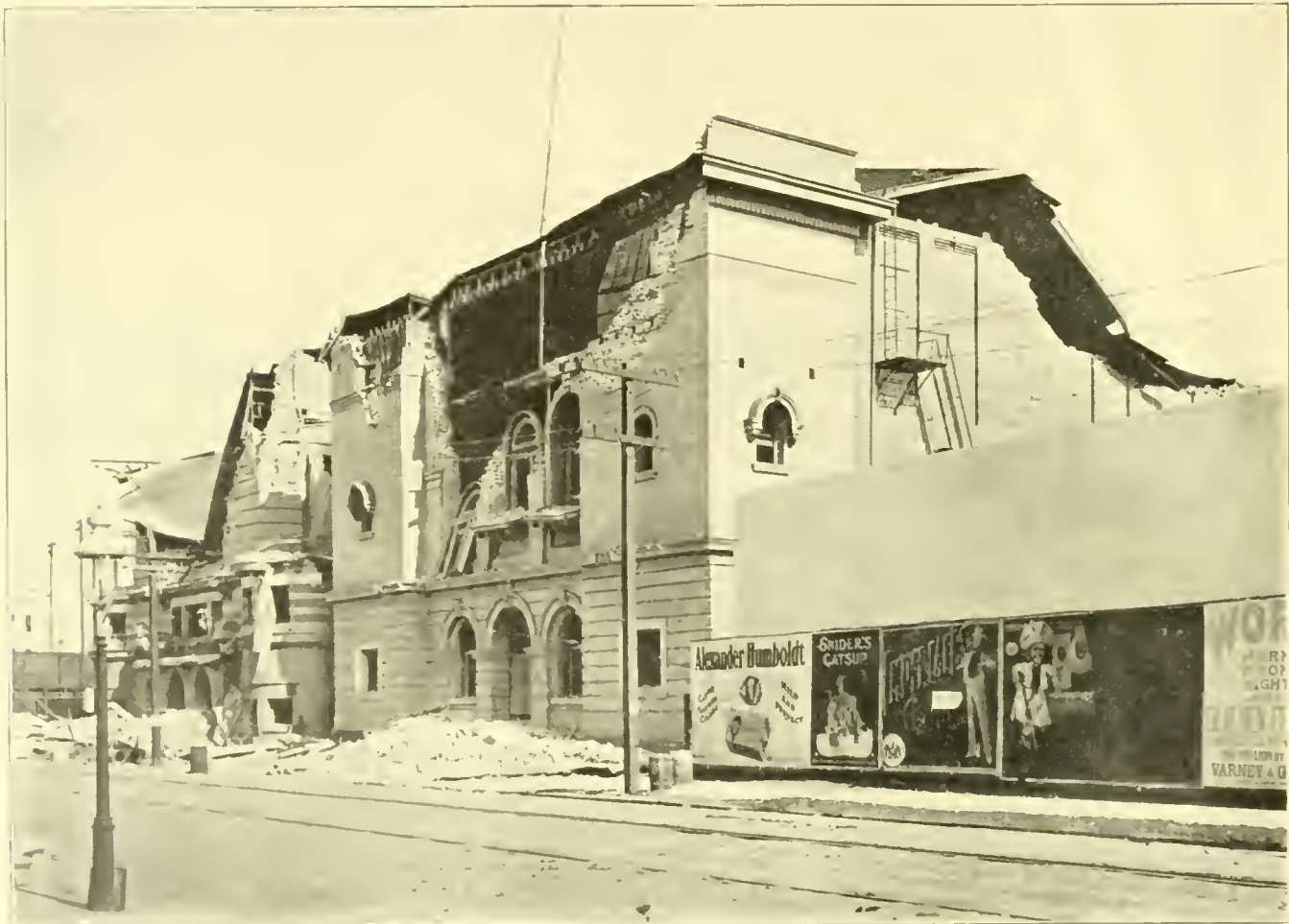
Scottish Rite, Masome Hall, with Jewish Synagogue on the left, Geary Street, near Fillmore, San Francisco, Damaged by Earthquake.
