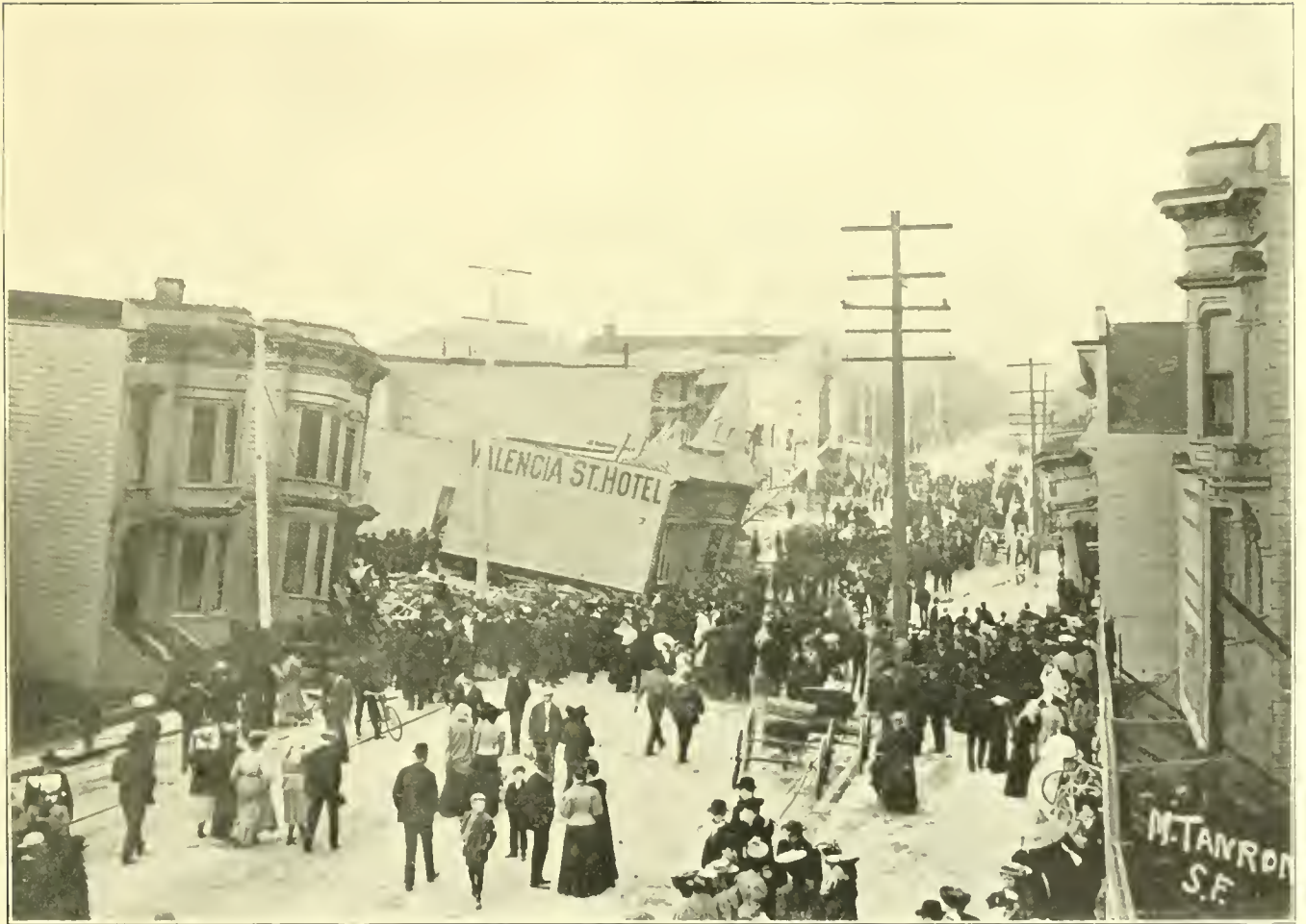
Valencia Street Four-Story Hotel Destroyed by Earthquake. Thirty People Killed.
