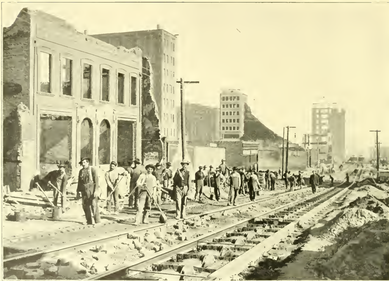
Repairing Tracks on Sutter Street after the Fire. Changing Line from Cable to Electric.
