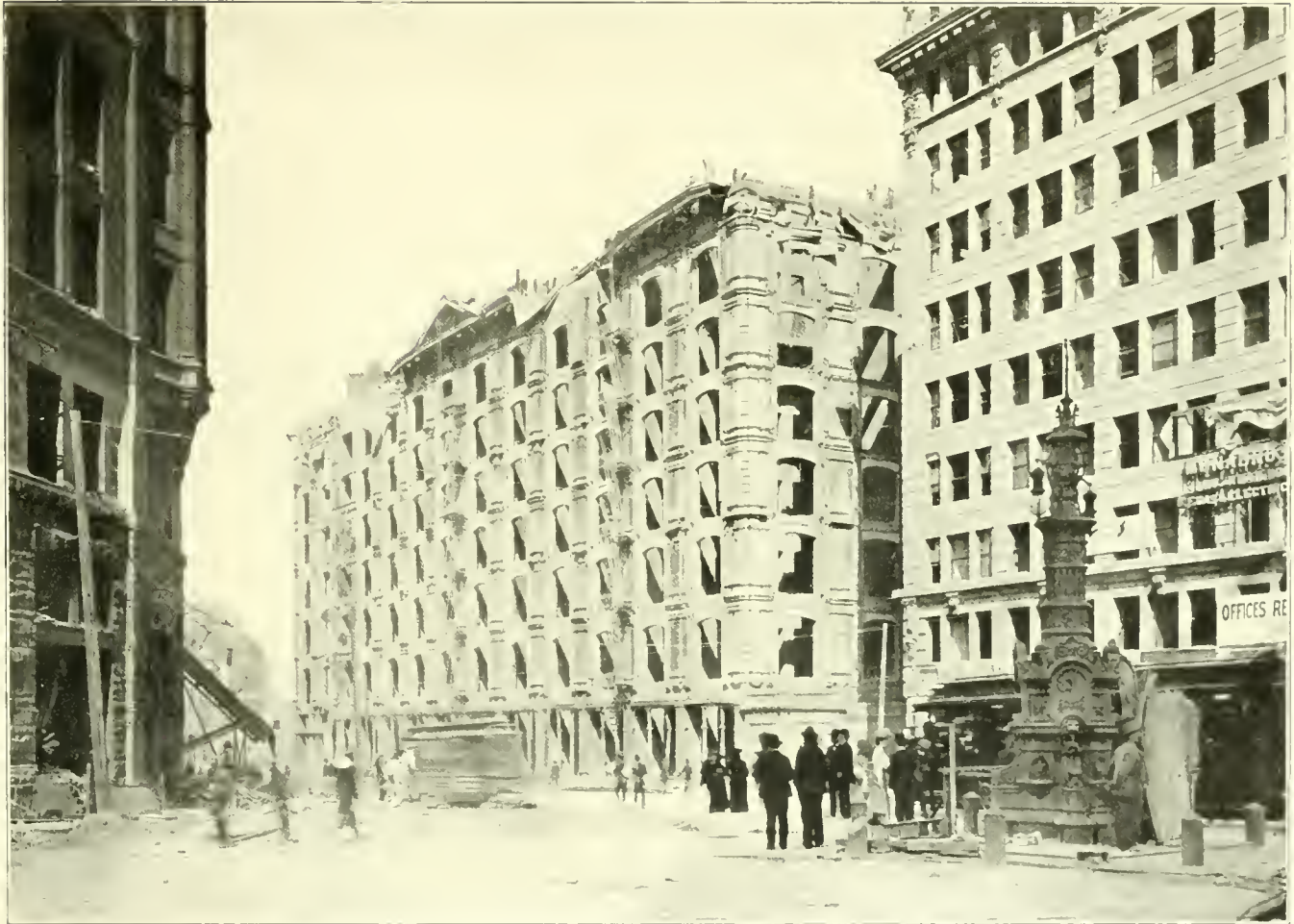
Palace Hotel, San Francisco, after the Fire, with Monadnock Block on right. Walls withstood both Fire and Earthquake.
