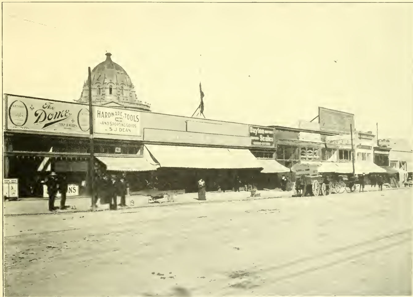
Market Street, between Eighth and Ninth, Rebuilt Since Fire. From photograph taken November, 1903.
