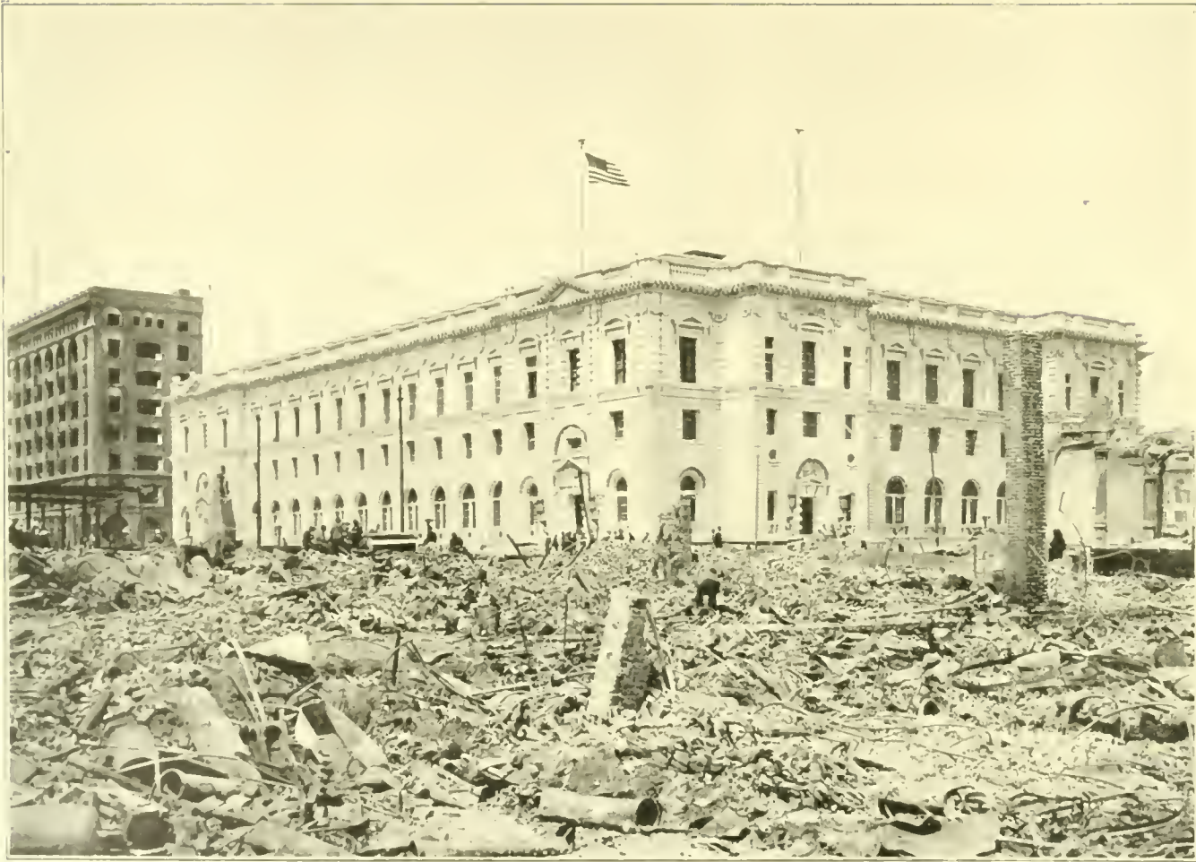
The New Postoffice, San Francisco—did not suspend business except for a few hours to fight fire. Grant Building at left.
