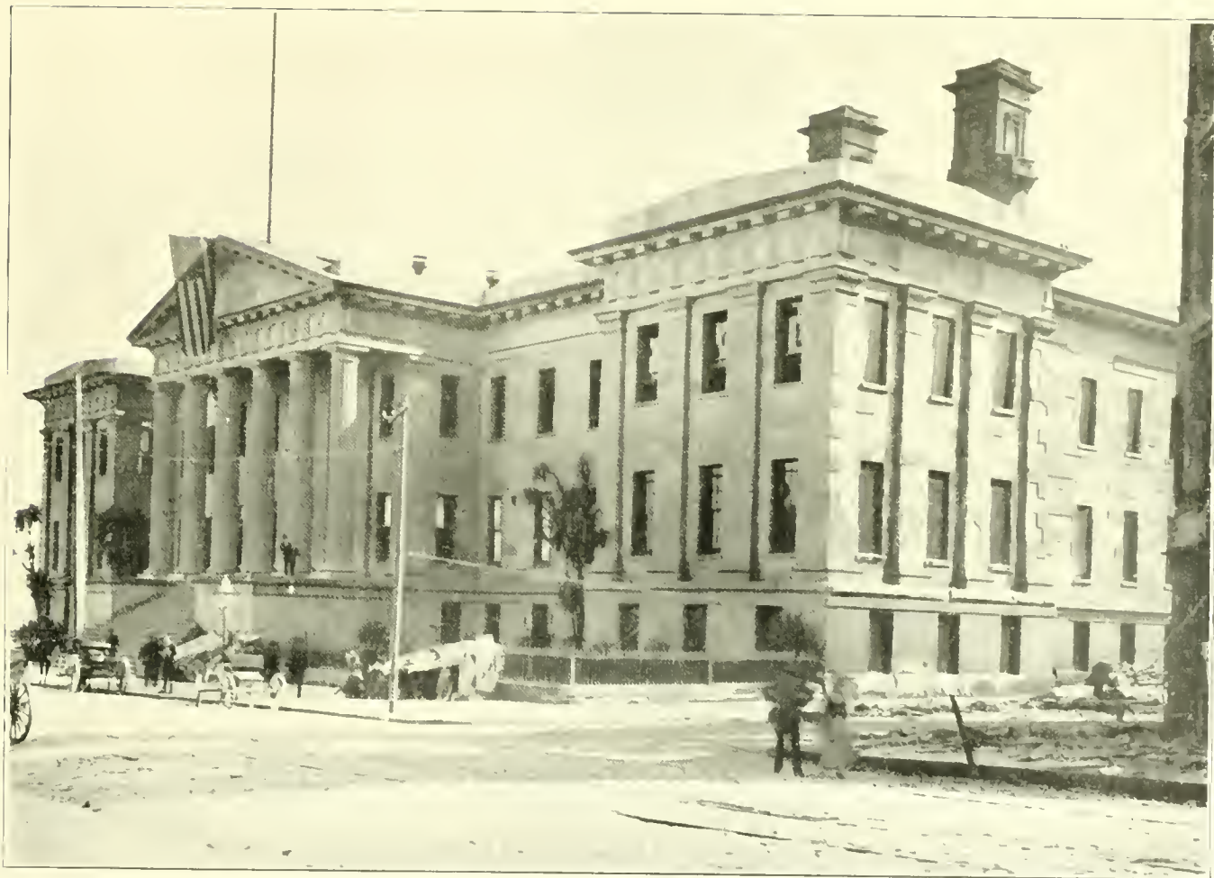
The Mint, San Francisco—Withstood both Earthquake and Fire with scarcely any Damage.
