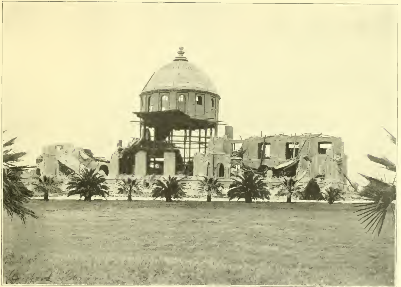
Stanford Library, Stanford University—Damaged by Earthquake.
