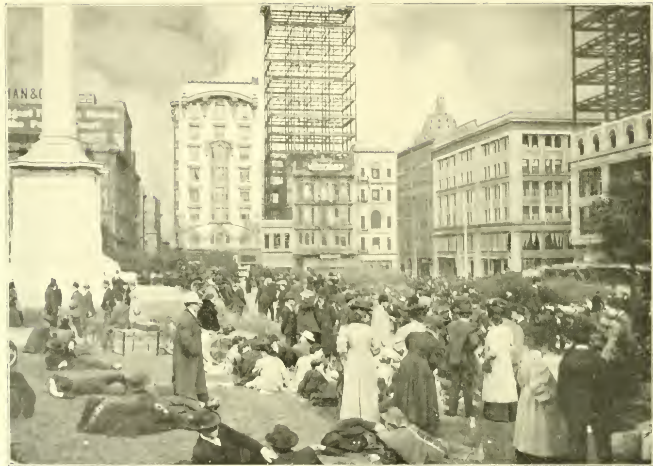
People fleeing from the flames resting in Union Square. All Buildings shown here afterwards burned.
