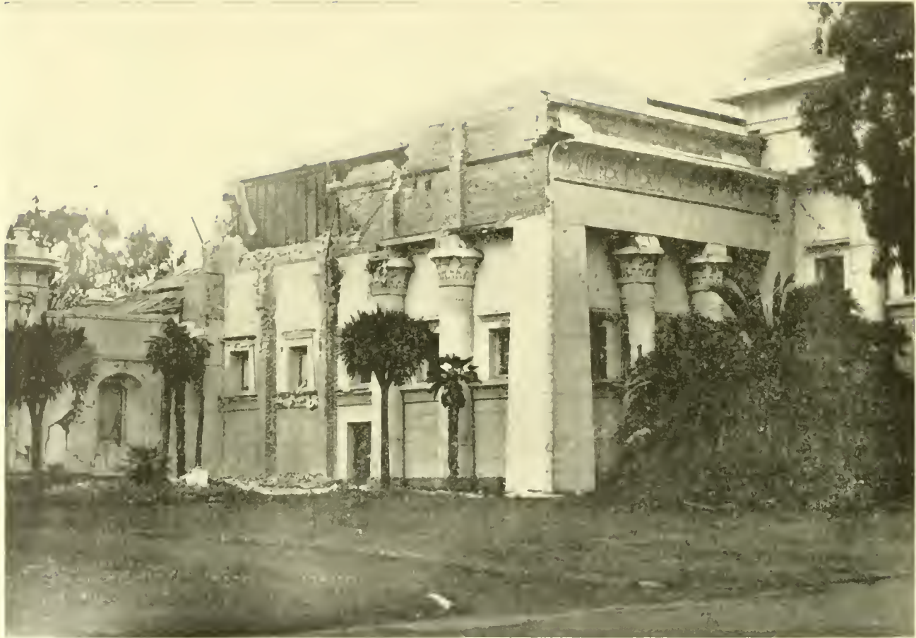
Museum, Golden Gate Park. Damaged by Earthquake.
