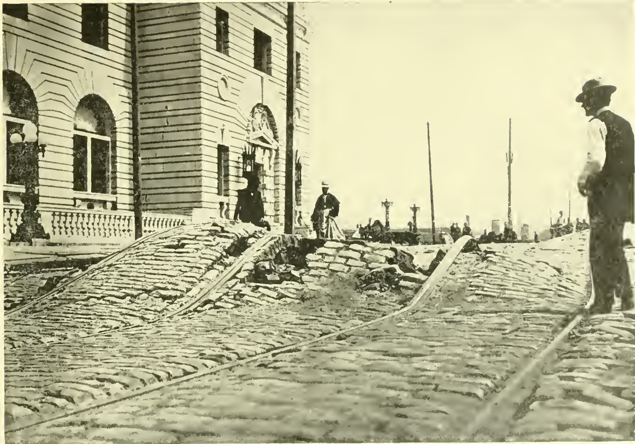
Result of Earthquake on Mission Street, opposite Postoffice.
