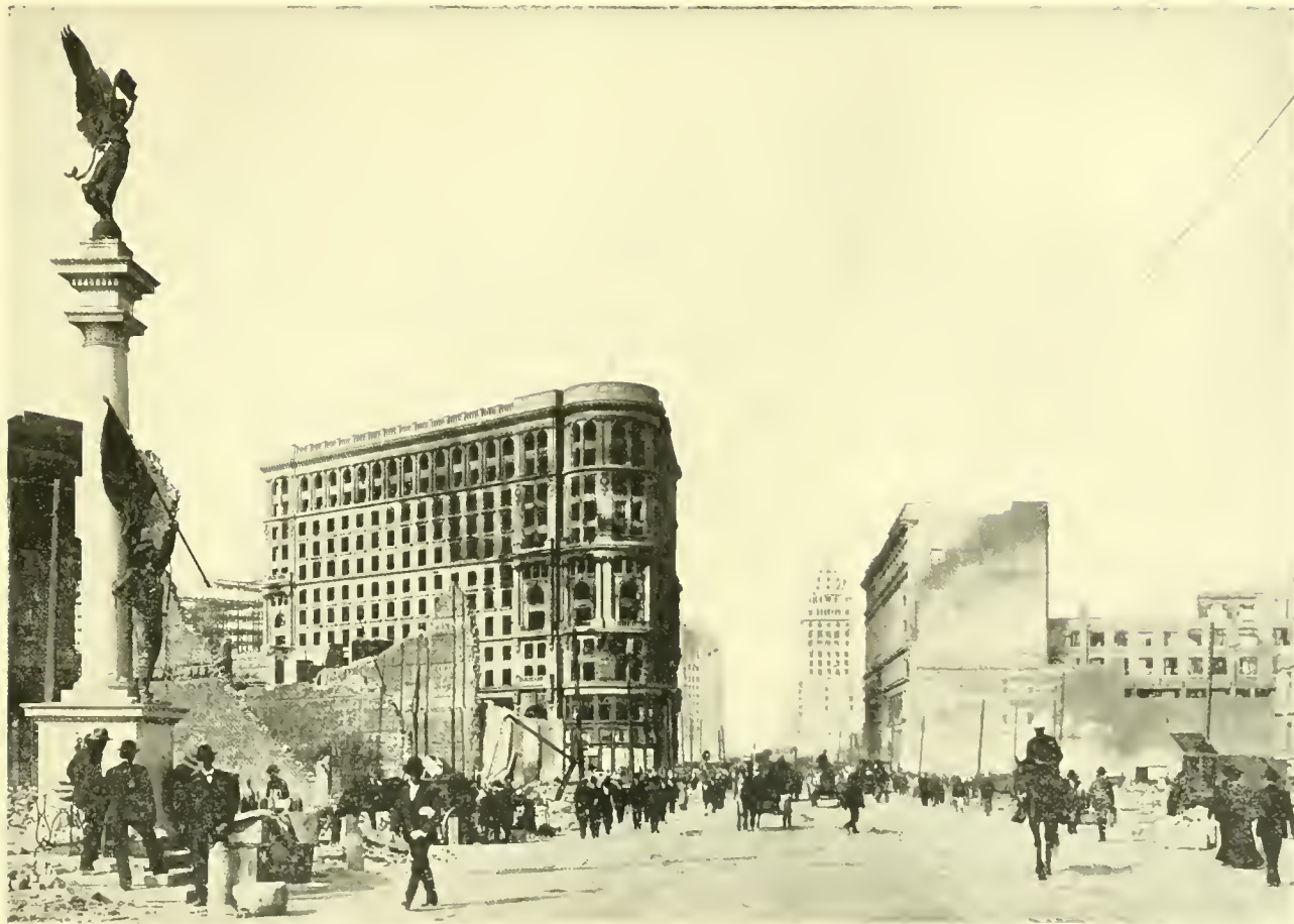
The James Flood Building after the Fire. Building was gutted by the Fire, but apparently not otherwise damaged. The City Treasurer now has his office here together with Western National Bank.
