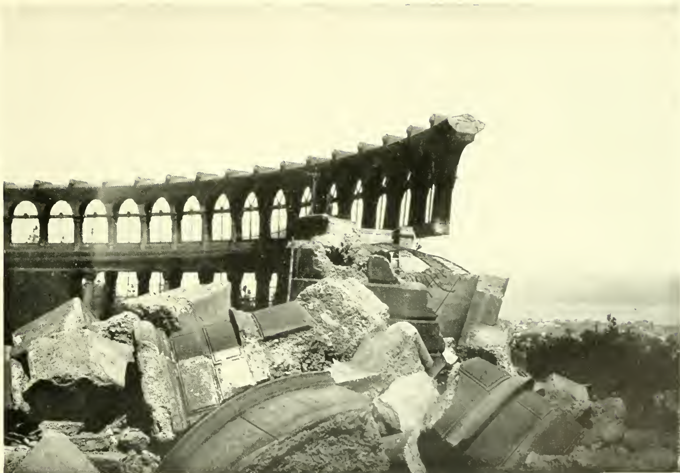
Observatory, Strawberry Hill, Golden Gate Park, San Francisco, Damaged by Earthquake.
