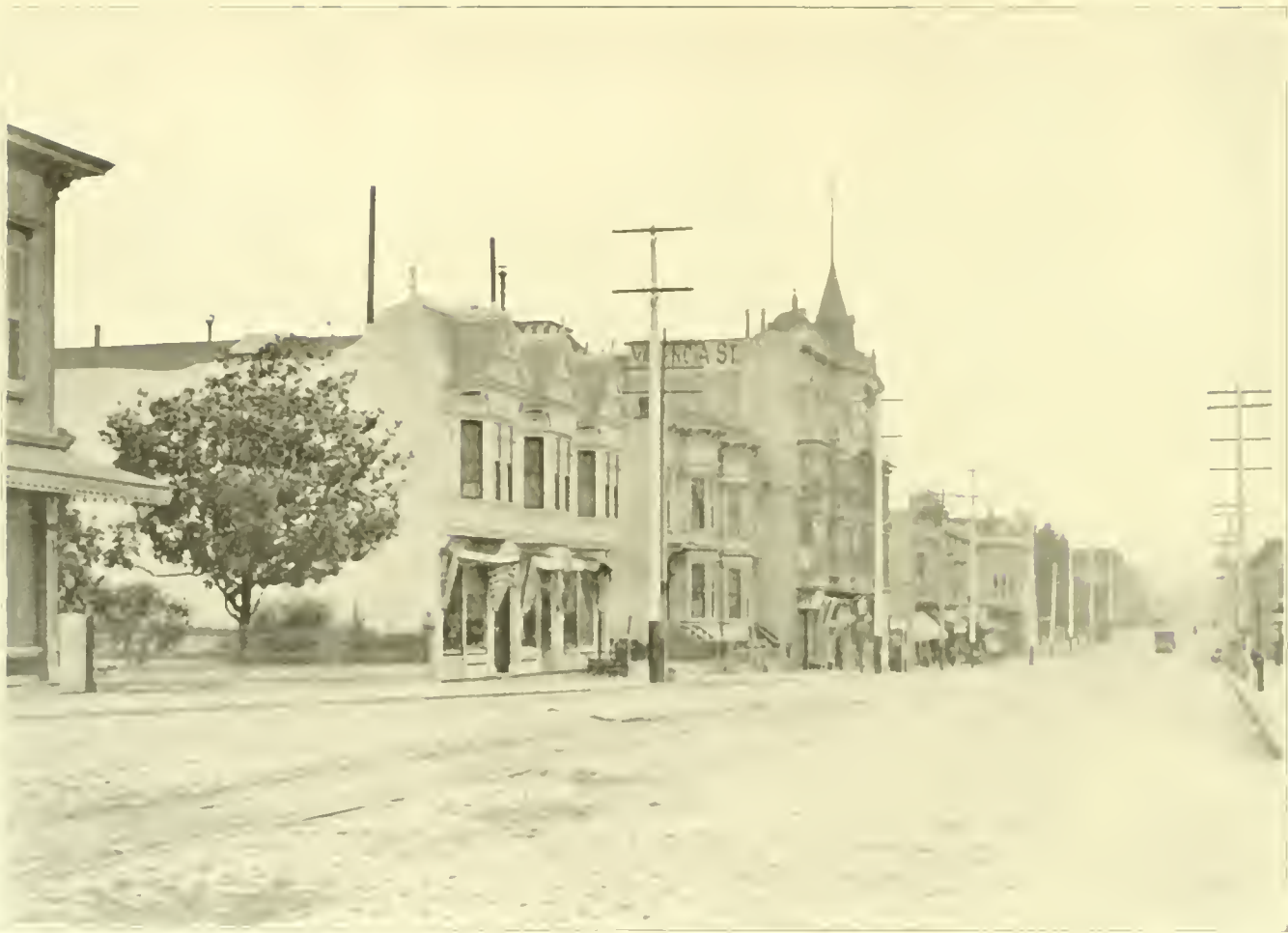
Valencia Street Hotel before the Earthquake.
