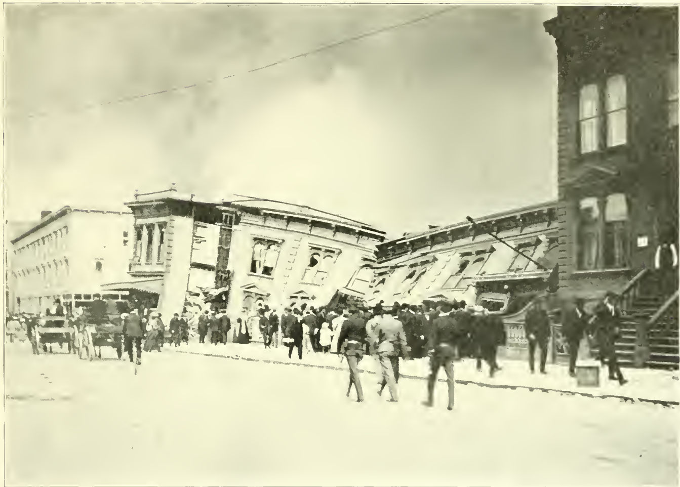
Cottages on Golden Gate Avenue, near Hyde Street, Wrecked by Earthquake.
