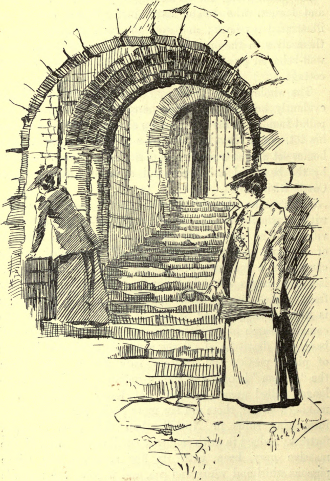
Staircase, Castle Rising.
