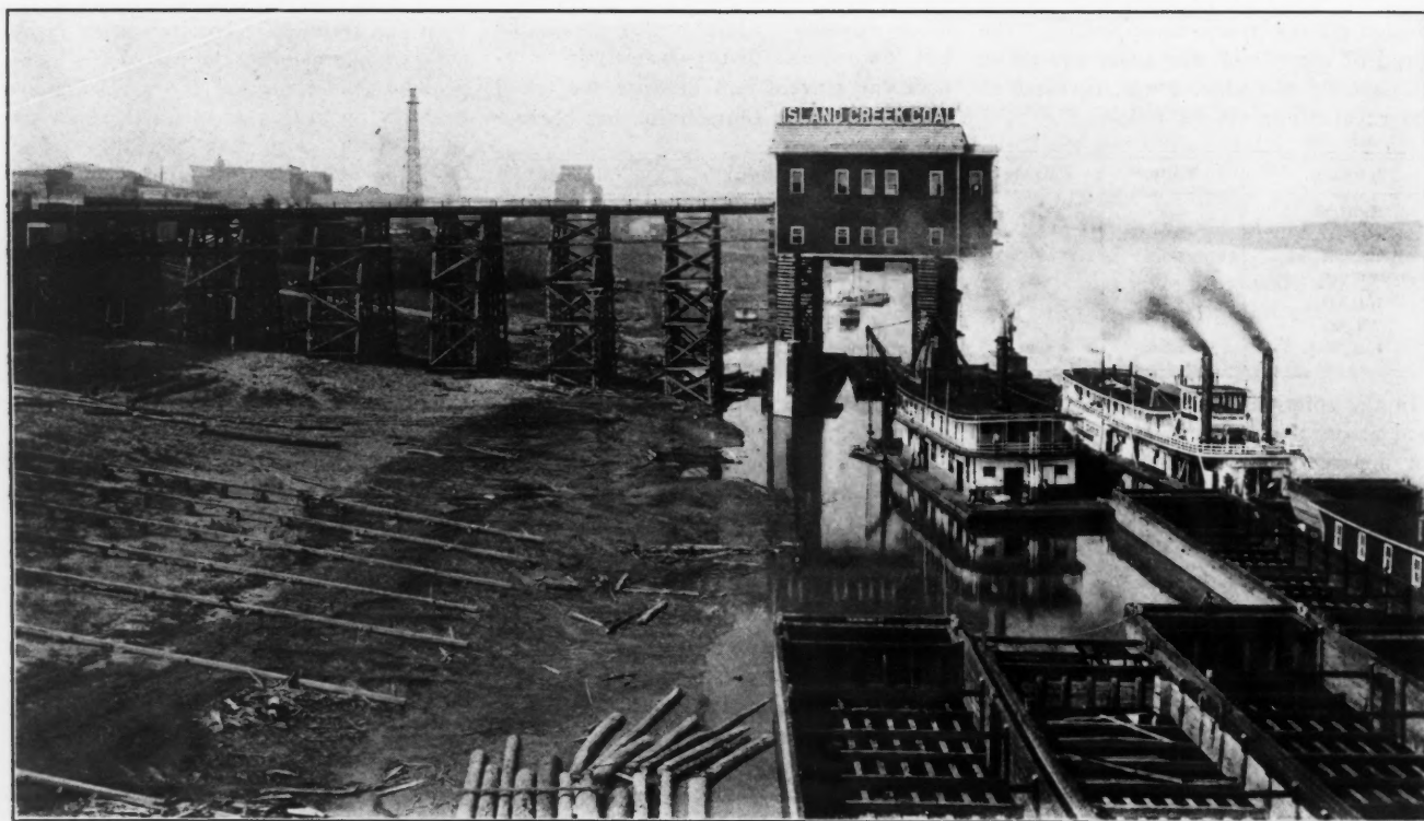
FIG. 7. LOADING PIER AT HUNTINGTON
