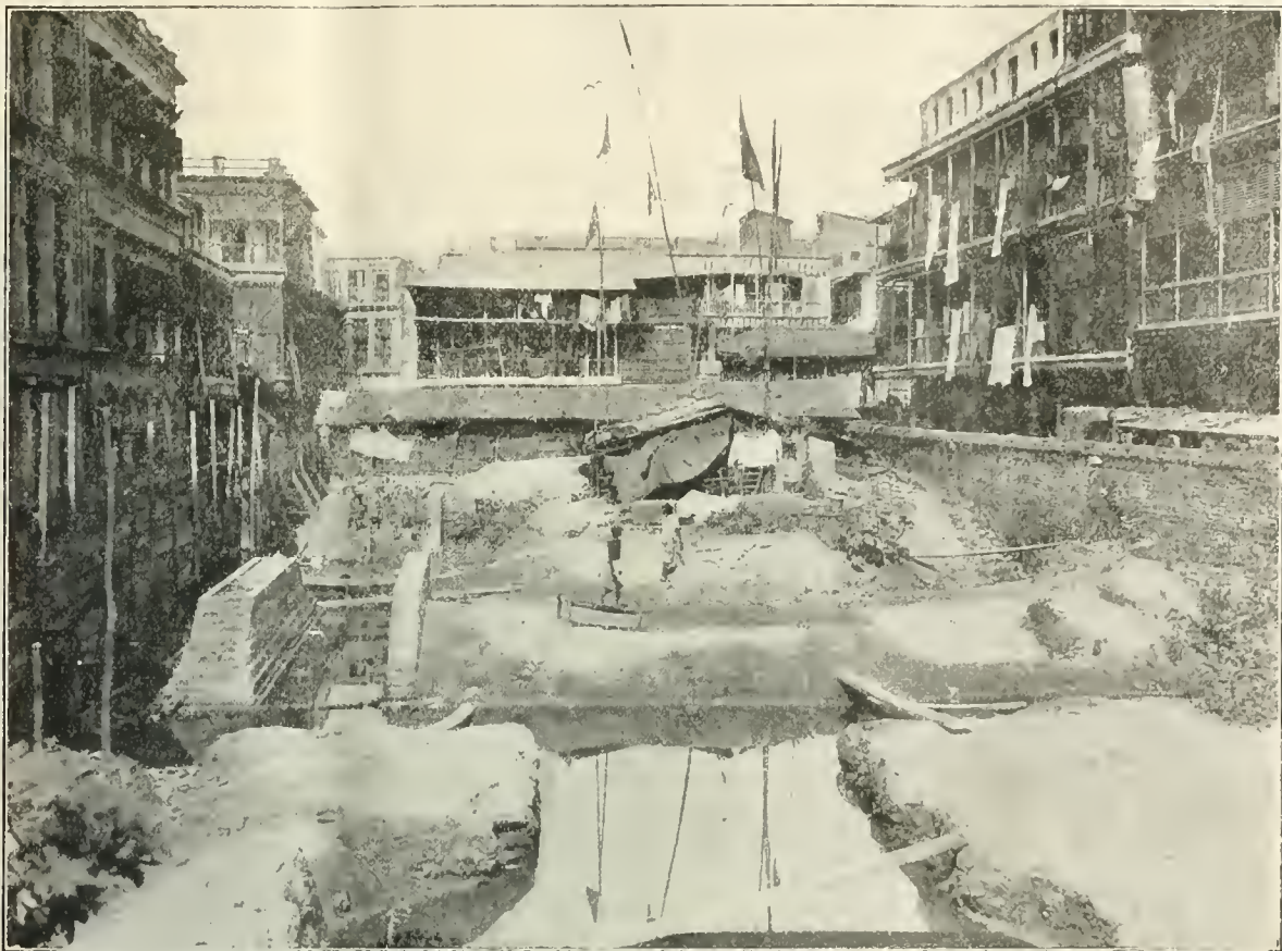
AN EXAMPLE OF INADEQUATE BY-LAWS, CALCUTTA.
