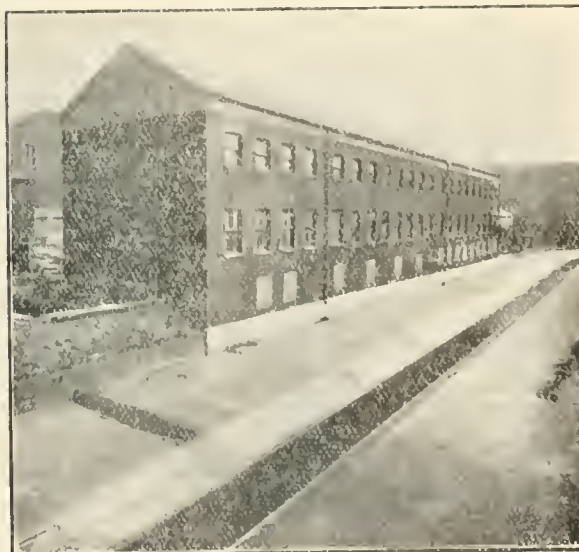
VIEW OF RIVER AFTER IMPROVEMENT (FIG. X).
