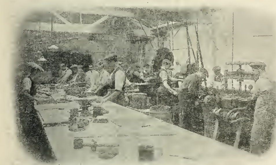
FORMING "DEXINE" ARTICLES FOR MOULDING DEPARTMENT.
