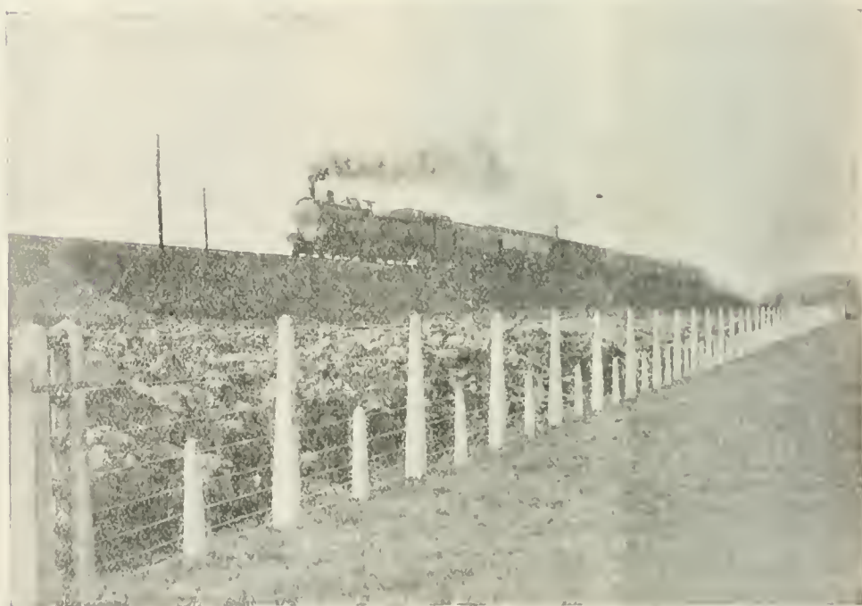
REINFORCED-CONCRETE FENCE POSTS AT CHINGFORD (METROPOLITAN WATER BOARD) AND ON THE L. & N.W. RAILWAY.
