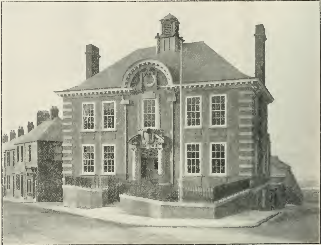
NEWBURN-ON-TYNE COUNCIL OFFICES.
