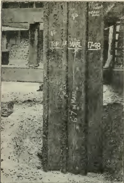
TEST PILES AT NEWPORT, MON.
