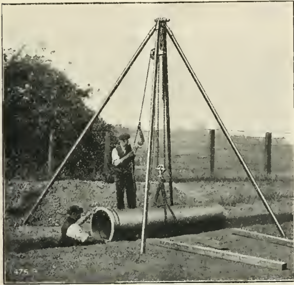
TUBULAR SHEAR-LEGS—PIPE LAYING.
