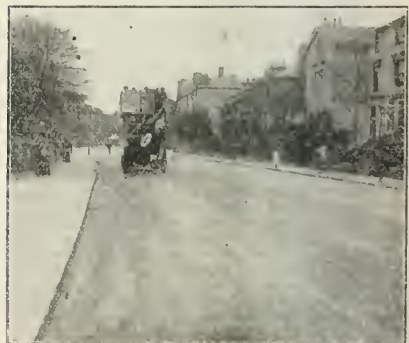
COMPLETED ROAD OPEN TO TRAFFIC AFTER APPLICATION OF GRANITE CHIPPINGS.
