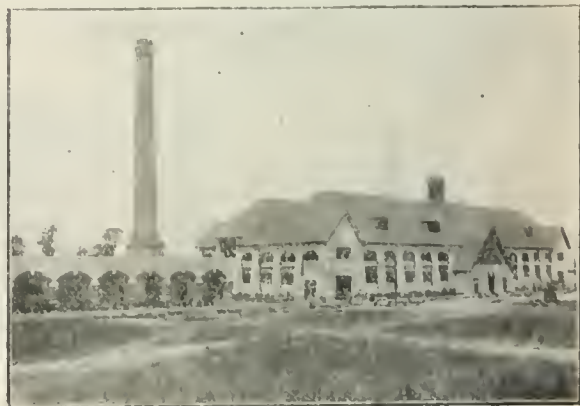
SOUTHEND DESTRUCTOR AND SEWAGE PUMPING STATION.
