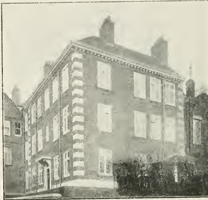
HARROW-ON-THE-HILL PUBLIC OFFICES: BACK ELEVATION.
