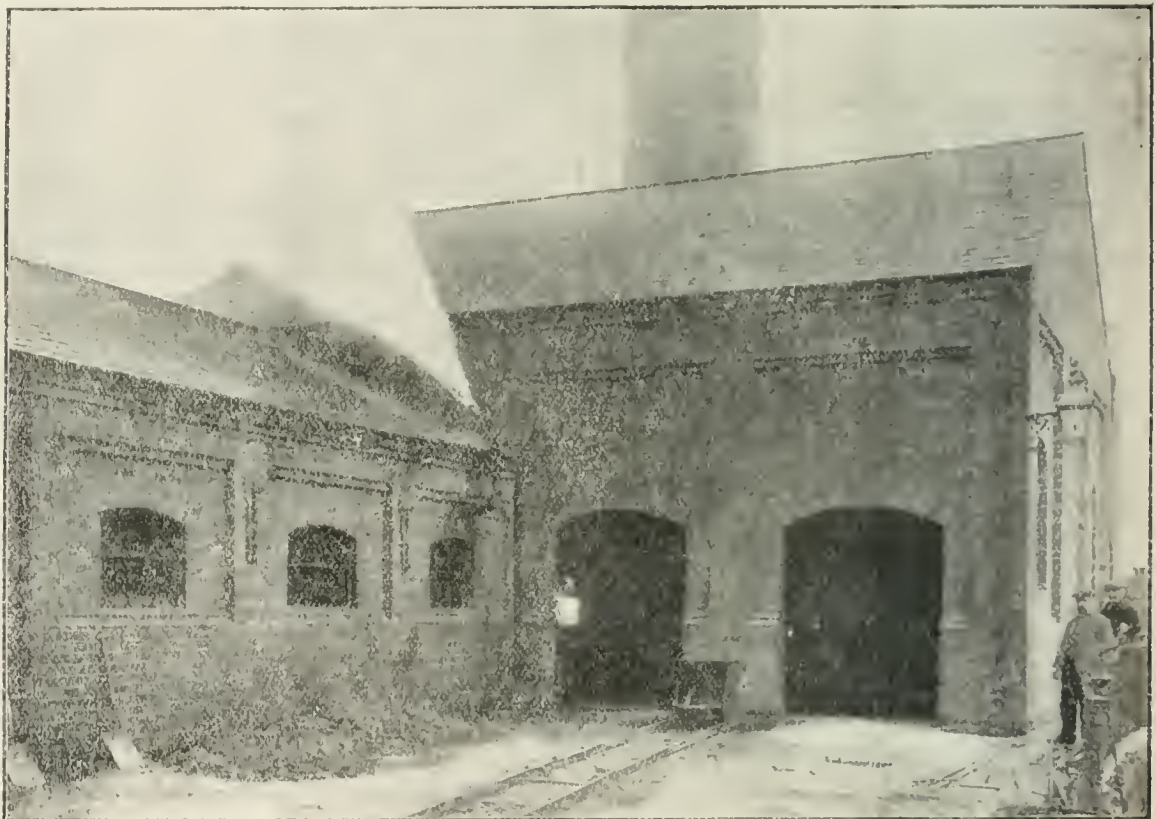
DONCASTER REFUSE DESTRUCTOR. GENERAL VIEW OF DESTRUCTOR BUILDING AND ENGINE-HOUSE.
