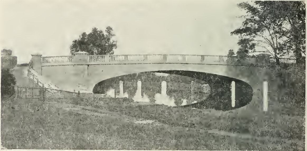
WOOD BRIDGE, GUILDFORD.
