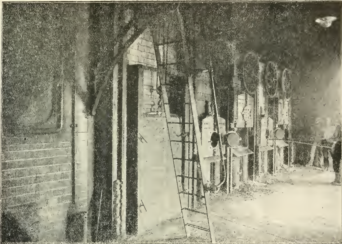
DONCASTER REFUSE DESTROYER. FURNACE FRONT.
