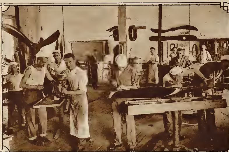
Aviation mechanics receiving instruction in tipping and balancing propellers. U. S. Naval Air Station, Pensacola, Fla
