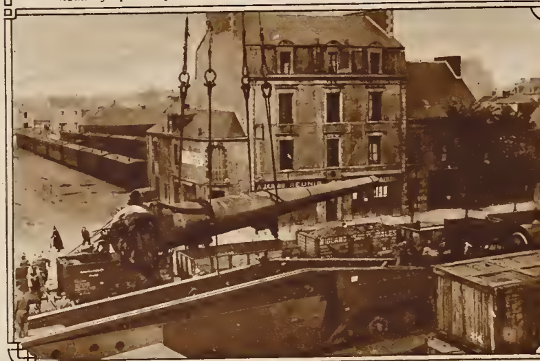
3—Swinging a 14-inch, 50 caliber rifle for United States Naval Railway Battery into position to be placed on girder and taken to the shops, St. Nazaire, France. August 1, 1918. 4—United States Naval Railway Battery leaving yards for the front. St. Nazaire, France. August 1, 1918.
