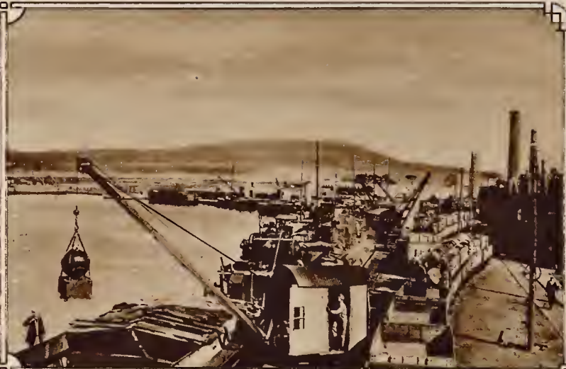
The loading basin for Naval Base No. 18 on the Caledonian Canal at Inverness, Scotland. The picture shows how the lighters were loaded to transfer the mines to the mine layers.
