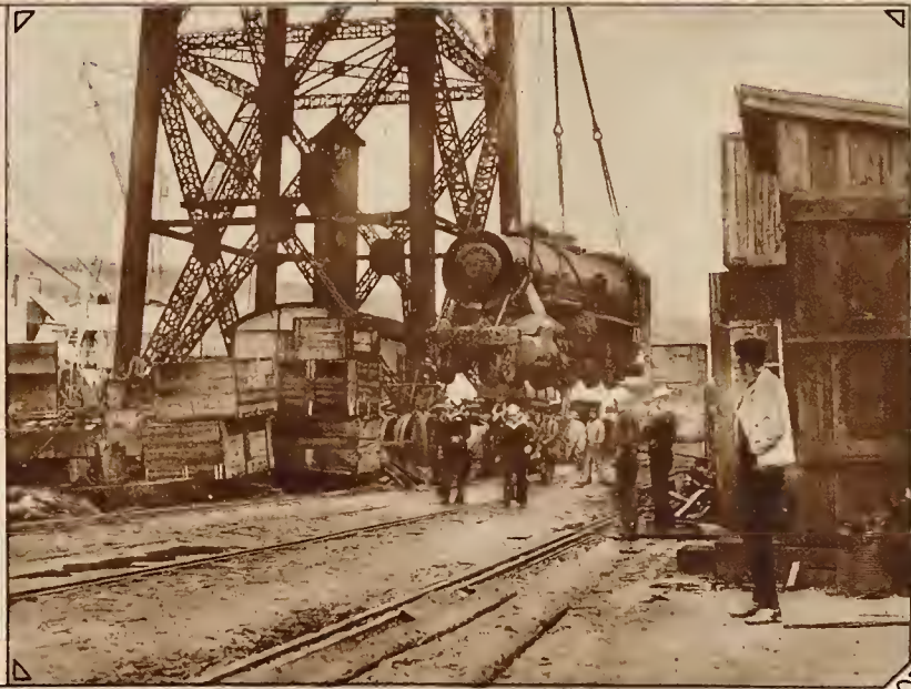
Unloading Baldwin locomotives from steamer to rails in fifteen seconds. U. S. S. "Firmore," Brest.
