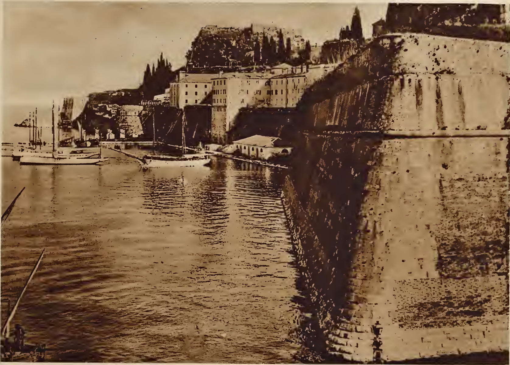
THE ISLAND OF CORFU. In the Spring of 1918, Admiral Sims sent Captain Richard H. Leigh to Southern Italy to locate and construct a subchaser base in that neighborhood. It was decided that the Bay of Govino, in the Island of Corfu, would best meet the requirements. "The immediate connection which was thus established between New London and this ancient city of classical Greece, fairly illustrates how widely the Great War had extended the horizon of the American people," says Rear Admiral Sims. "There was a certain appropriateness in the fact that the American college boys who commanded these little ships—not much larger than the vessel in which Ulysses had sailed these same waters three thousand years before—should have made their base on the same island which had served as a naval station for Athens in the Peloponnesian War, and which, several centuries afterward, had been used for the same purpose by Augustus in the struggle with Antony. And probably the sight of the Achilleion, the Kaiser's palace, which was not far from this new American base, was not without its influence in constantly reminding our young men of the meaning of this unexpected association of Yankee-land with the ancient world."
