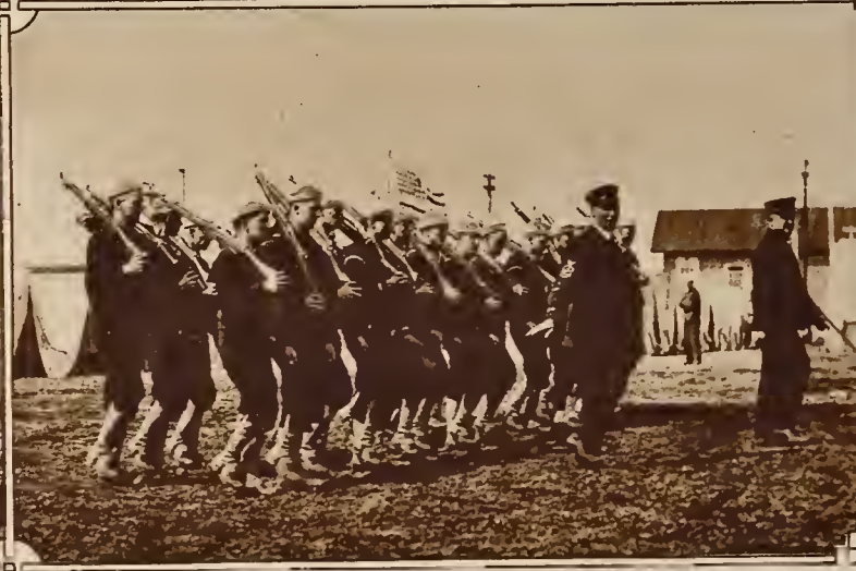
Drilling at League Island.
