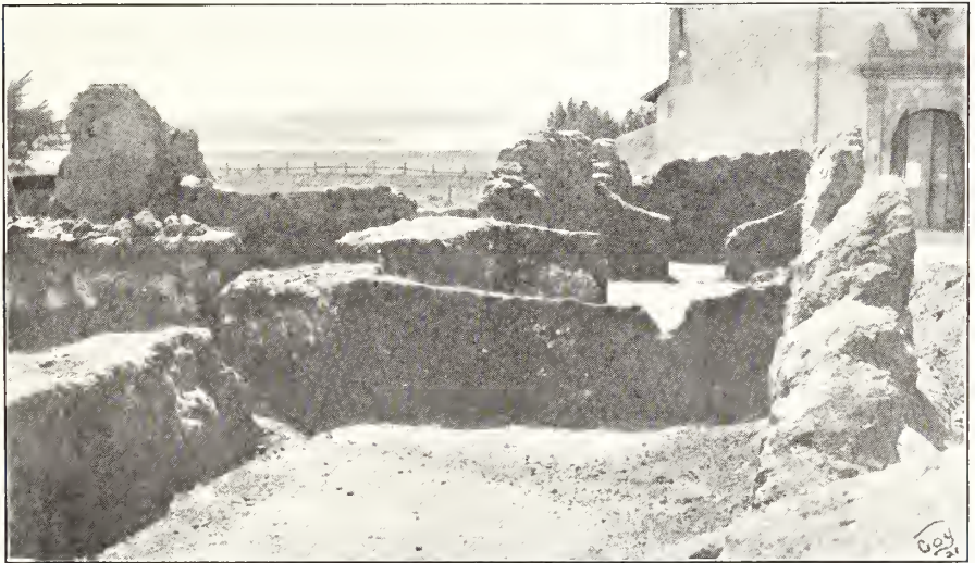
PLATE 37. Same Mound After Excavation, April, 1921. Coy, photo.
