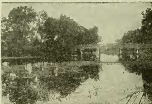
The Old North Bridge where Concord Fight Took Place
