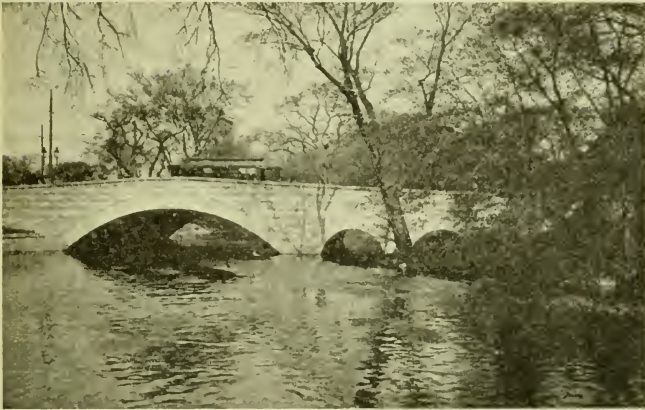
Approaching Boston, We Cross Mattapan Bridge
