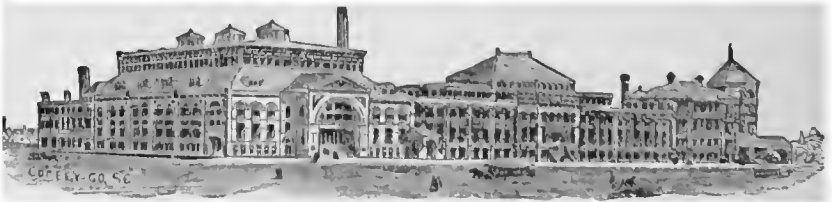
MECHANICS' FAIR BUILDING, BOSTON.
