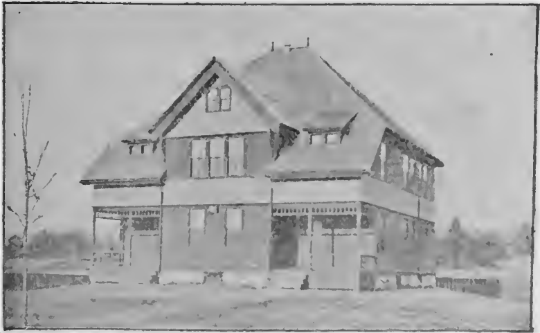
HIGH SCHOOL BUILDING, WILMINGTON.
