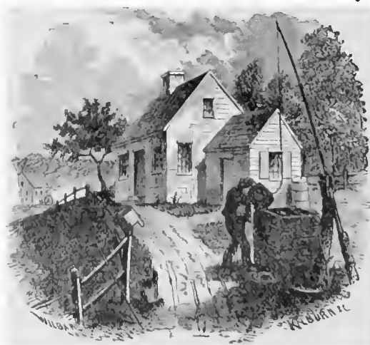
THE "OLD OAKEN BUCKET," SCITUATE.
