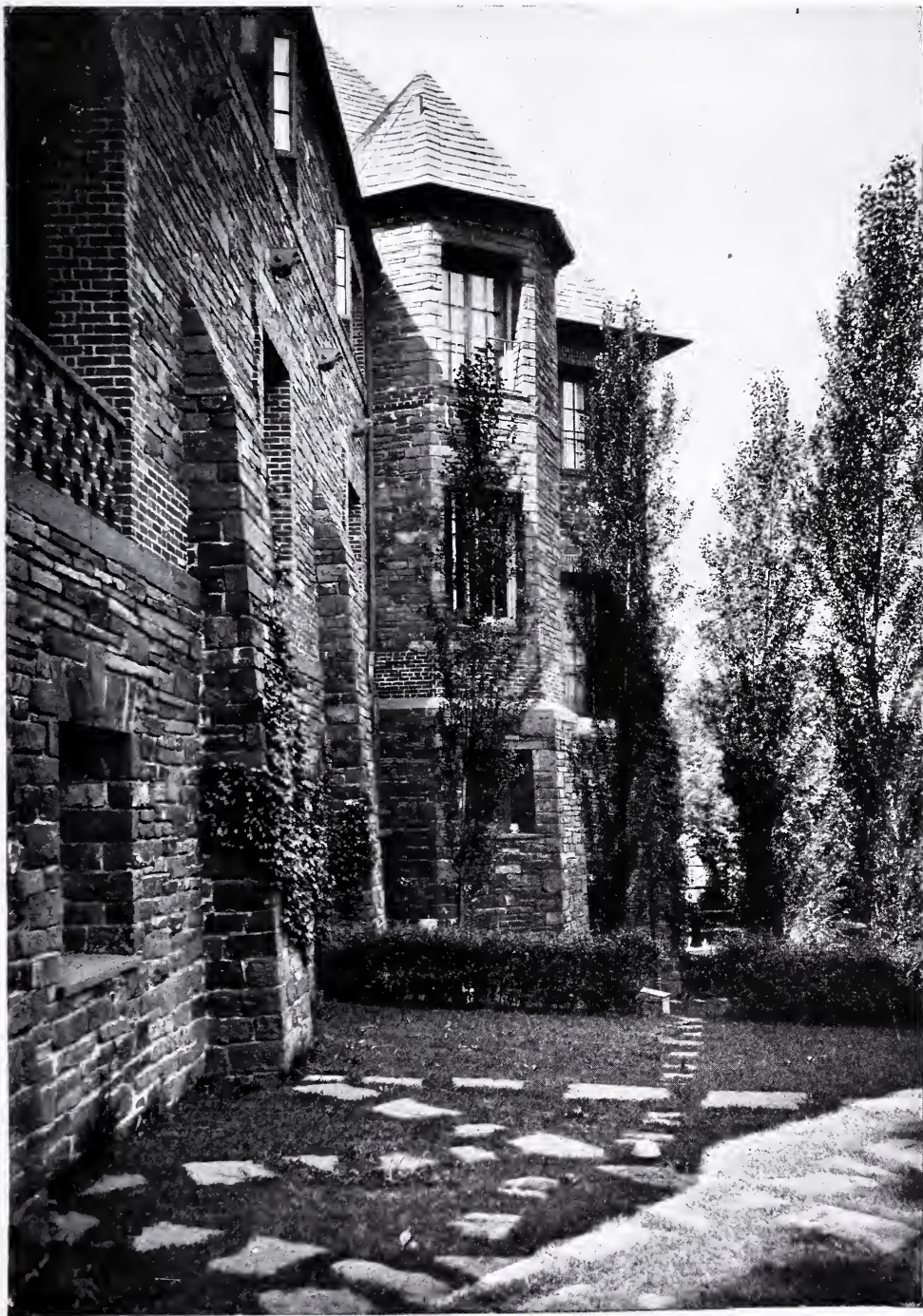
THE SERVICE WING (POINT OF VIEW 18 ON PLAN)— RESIDENCE OF GEORGE HOWE, ESQ., CHESTNUT HILL, PHILADELPHIA. MELLOR, MEIGS & HOWE, ARCHITECTS.
