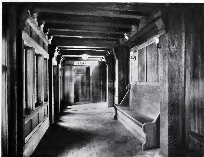
FOYER—WINEMA THEATRE, SCOTIA, HUMBOLDT COUNTY, CAL. Alfred Henry Jacobs, Architect.
