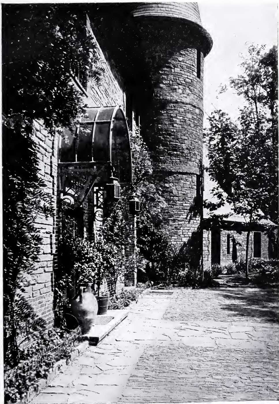
THE ENTRANCE AND TOWER FROM THE GATE OF THE UPPER TERRACE (POINT OF VIEW 5 ON PLAN)—RESIDENCE OF GEORGE HOWE, ESQ., CHESTNUT HILL, PHILADELPHIA. MELLOR, MEIGS & HOWE, ARCHITECTS.
