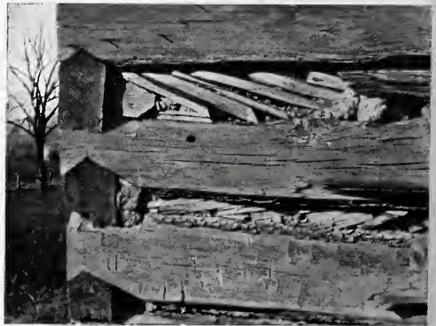
ANGLE VIEW OF EARLY LOG HOUSE, SHOWING "CHINKING."
