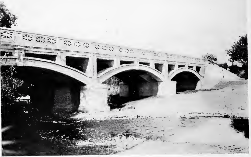
BRIDGE OVER THE INABON RIVER, ON THE ROAD BETWEEN PONCE AND SANTA ISABEL, P. R.
