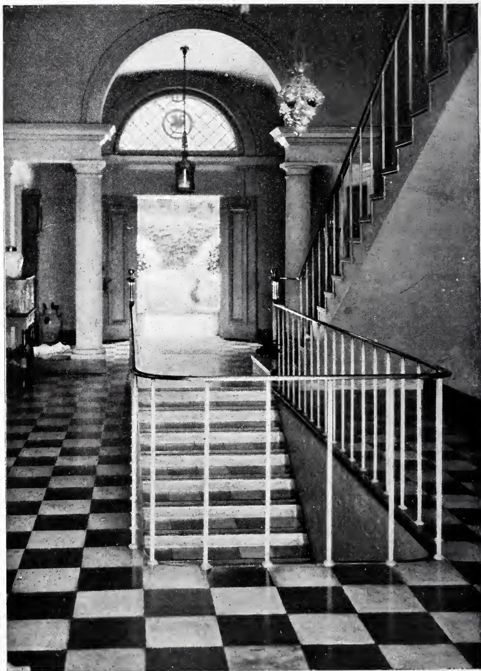
THE STAIR HALL LOOKING TOWARD THE ENTRANCE (POINT OF VIEW 8 ON PLAN)—RESIDENCE OF GEORGE HOWE, ESQ., CHESTNUT HILL, PHILADELPHIA. MELLOR, MEIGS & HOWE, ARCHITECTS.
