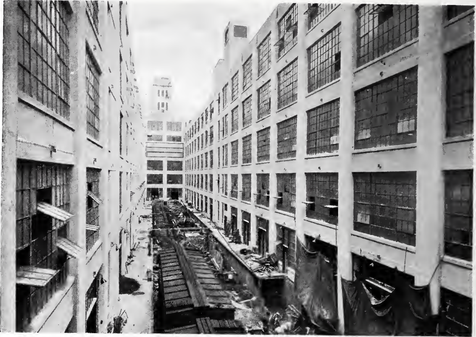
AMERICAN CHICLE COMPANY'S FACTORY, LONG ISLAND CITY, N. Y. Ballinger & Perrot (now The Ballinger Company), Architects and Engineers.
