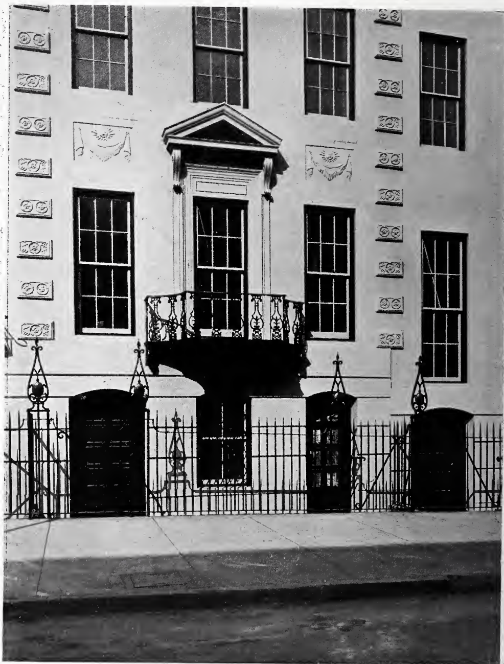
DETAIL OF ONE OF THE FORTY-EIGHTH STREET HOUSES—TURTLE BAY GARDENS, NEW YORK CITY. EDWARD C. DEAN AND WILLIAM LAWRENCE BOTTOMLEY, ASSOCIATE ARCHITECTS.
