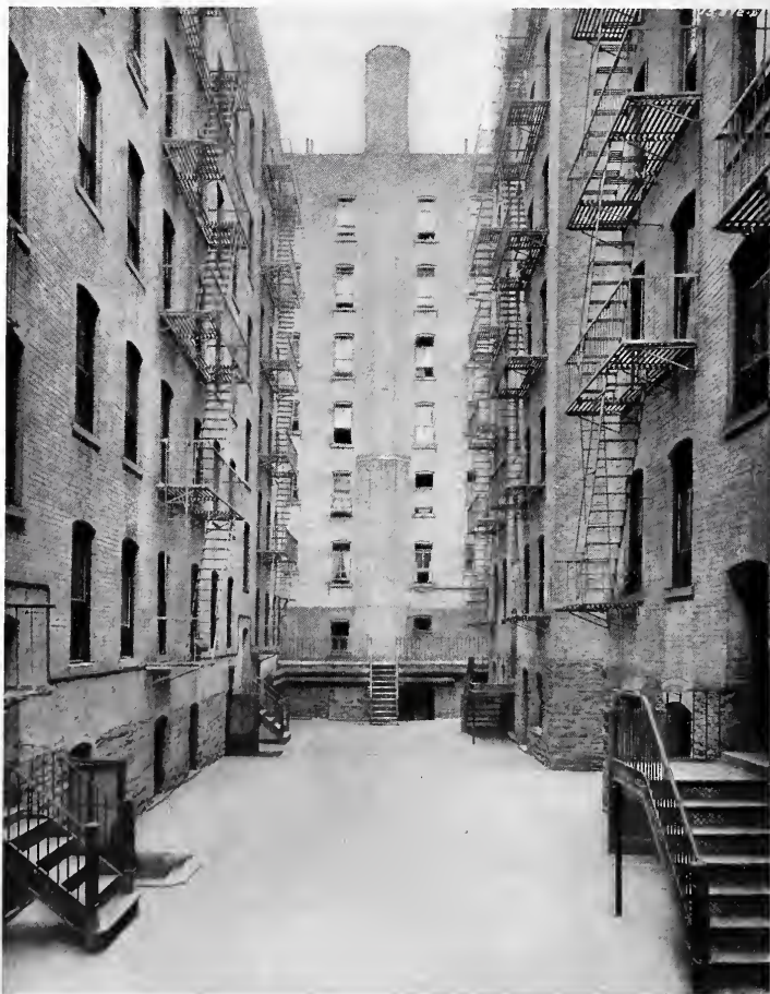
REAR YARDS OF BLOCK DEVELOPMENT AT 511 EAST SEVENTY-EIGHTH STREET, MANHATTAN.
