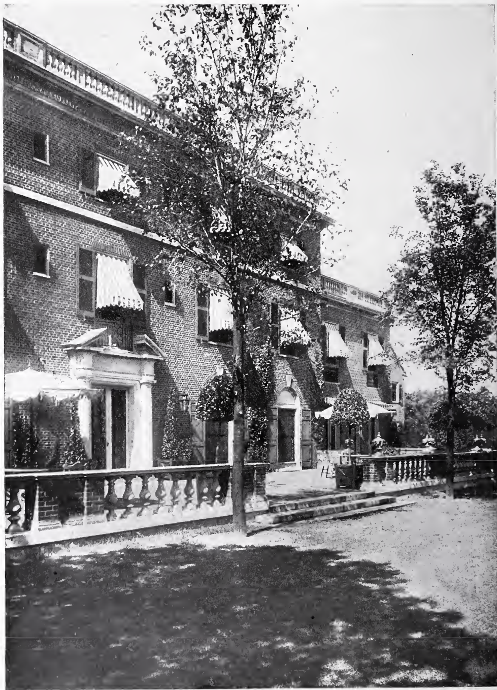
VIEW FROM WEST TERRACE—RESIDENCE OF GUERNSEY CURRAN, ESQ., OYSTER BAY, L. I. GUY LOWELL, ARCHITECT.
