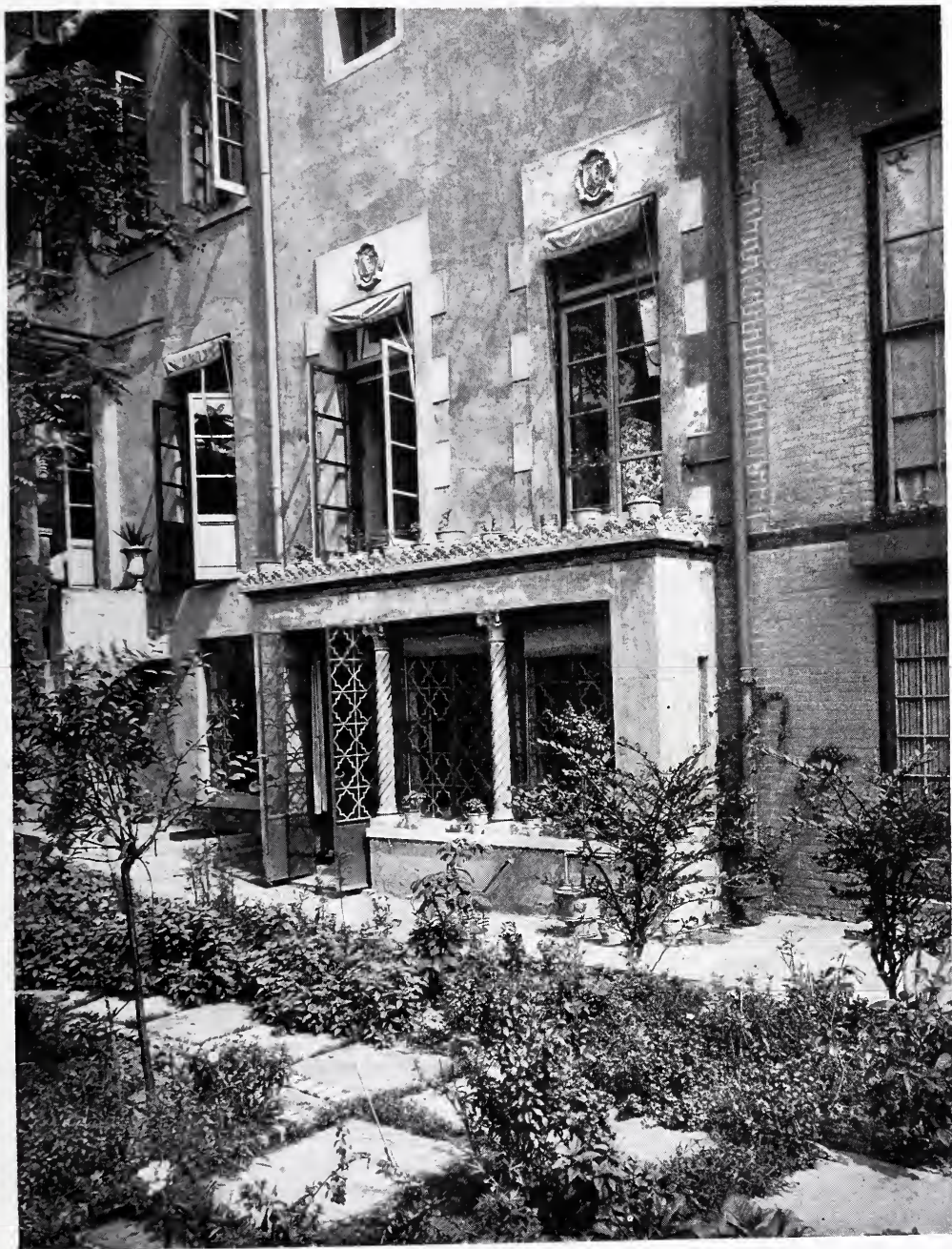
SPANISH DETAILS OF THE GARDEN FAÇADE OF THE FORTY-NINTH STREET HOMES— TURTLE BAY GARDENS, NEW YORK CITY. EDWARD C. DEAN AND WILLIAM LAWRENCE BOTTOMLEY, ASSOCIATE ARCHITECTS.
