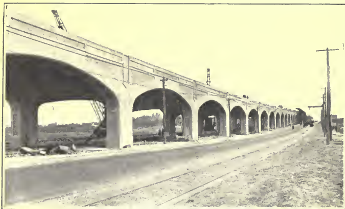
ELEVATED RAILROAD, CONCRETE MASONRY VIADUCT
