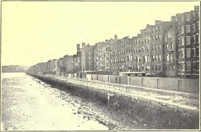
CHARLES RIVER BASIN, BOSTON, BEFORE IMPROVEMENT, SHOWING WATER AT LEVEL OF LOW TIDE
