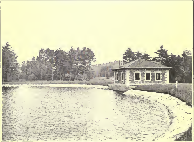
SCREEN CHAMBER, WESTON RESERVOIR
