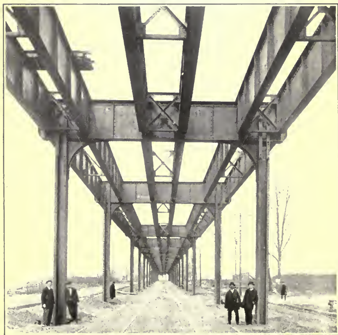
ELEVATED RAILROAD, STEEL STRUCTURE
