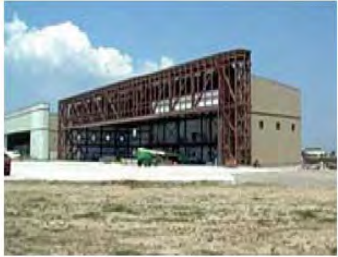
Figure 50 – Aircraft Maintenance Hangar
