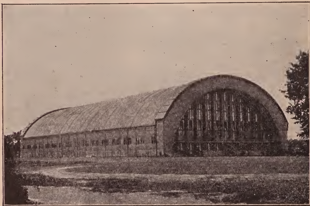
THE ARMORY, UNIVERSITY OF ILLINOIS, URBANA
