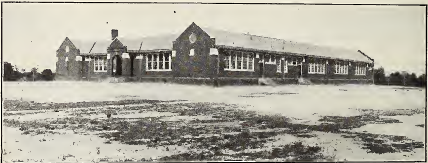
Why should the grounds around North Carolina school buildings be neglected like this? No trees; no shrubs; nothing green except a patch of grass and weeds to break the sea of sand. A few dollars in plants would work wonders here.
