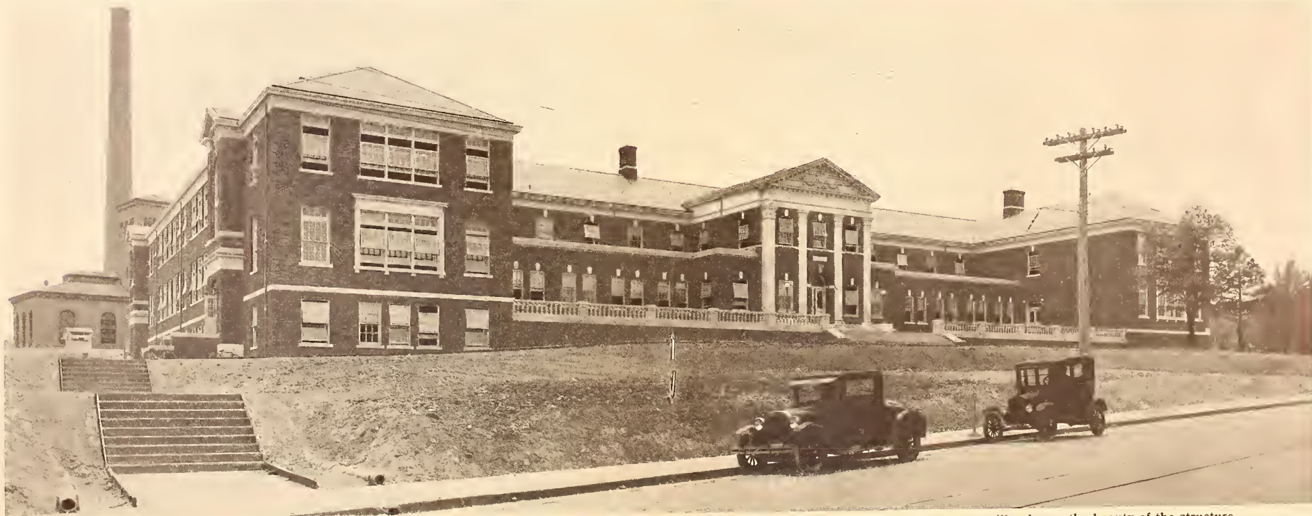
The new Training School connected with the North Carolina College for Women, at Greensboro. Here, again, correct landscape treatment will enhance the beauty of the structure
