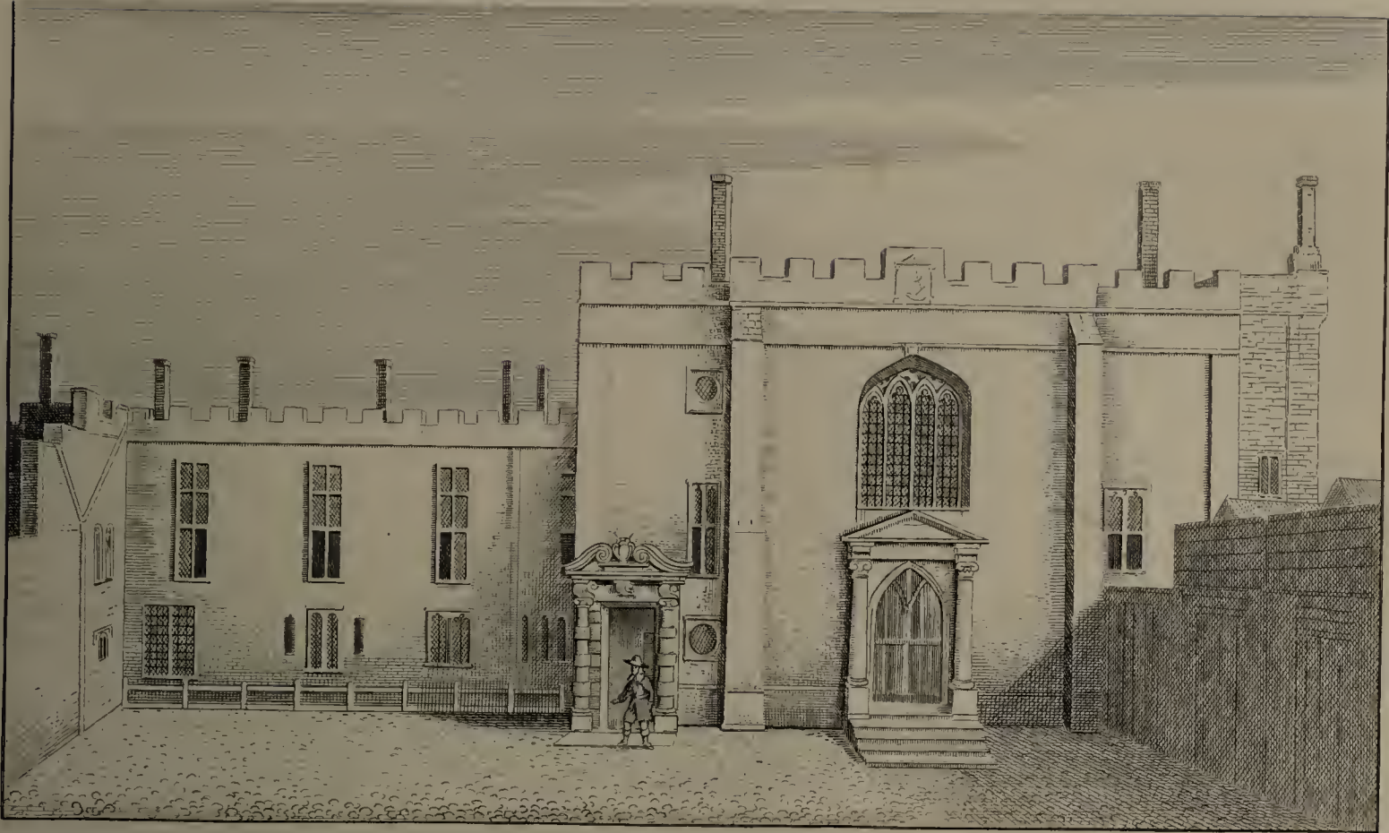
Remains of the Western Front of the Chapel of the House of Hospitallers of St. John of Jerusalem.
