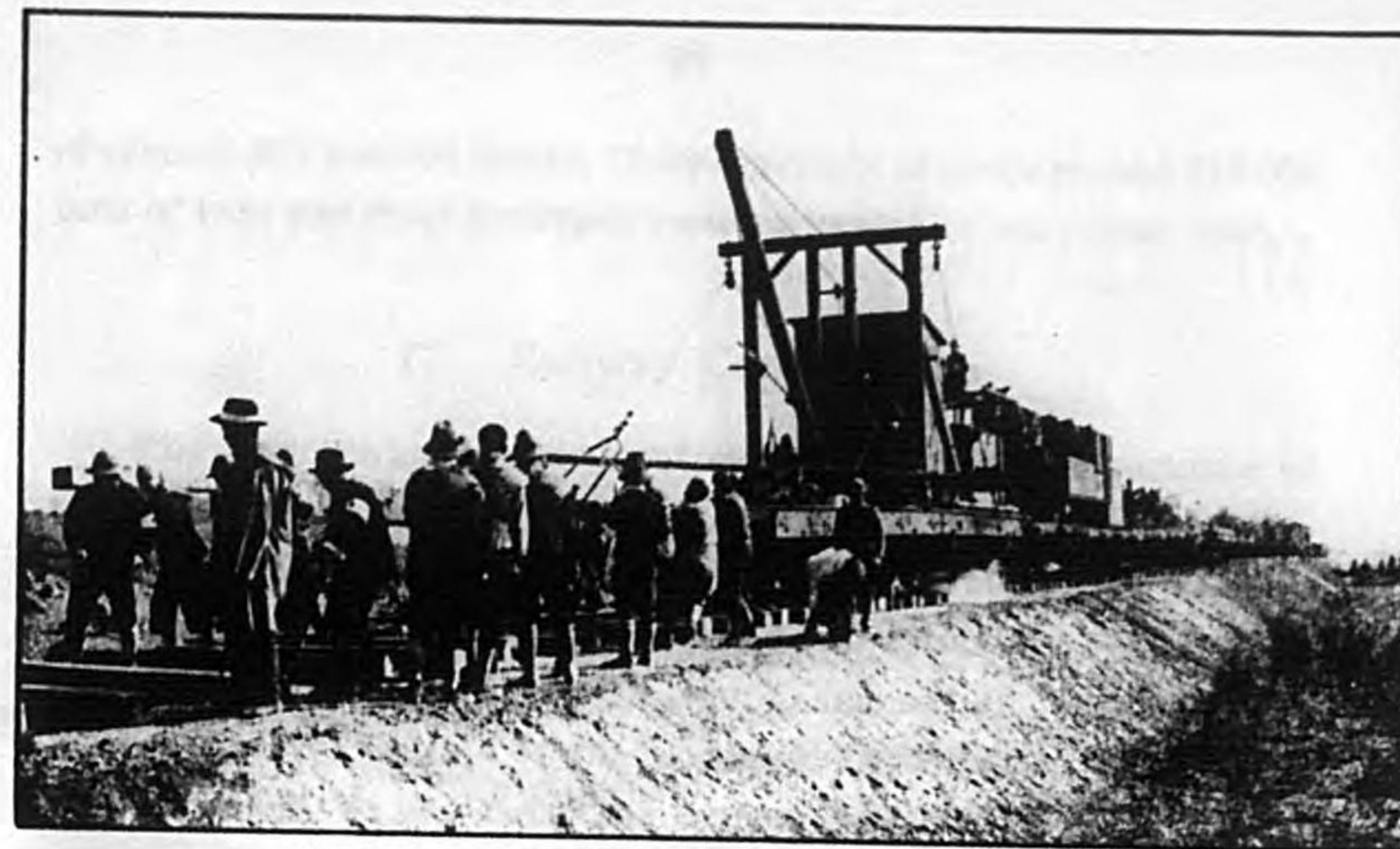
A Scene of the Railway Construction Work
