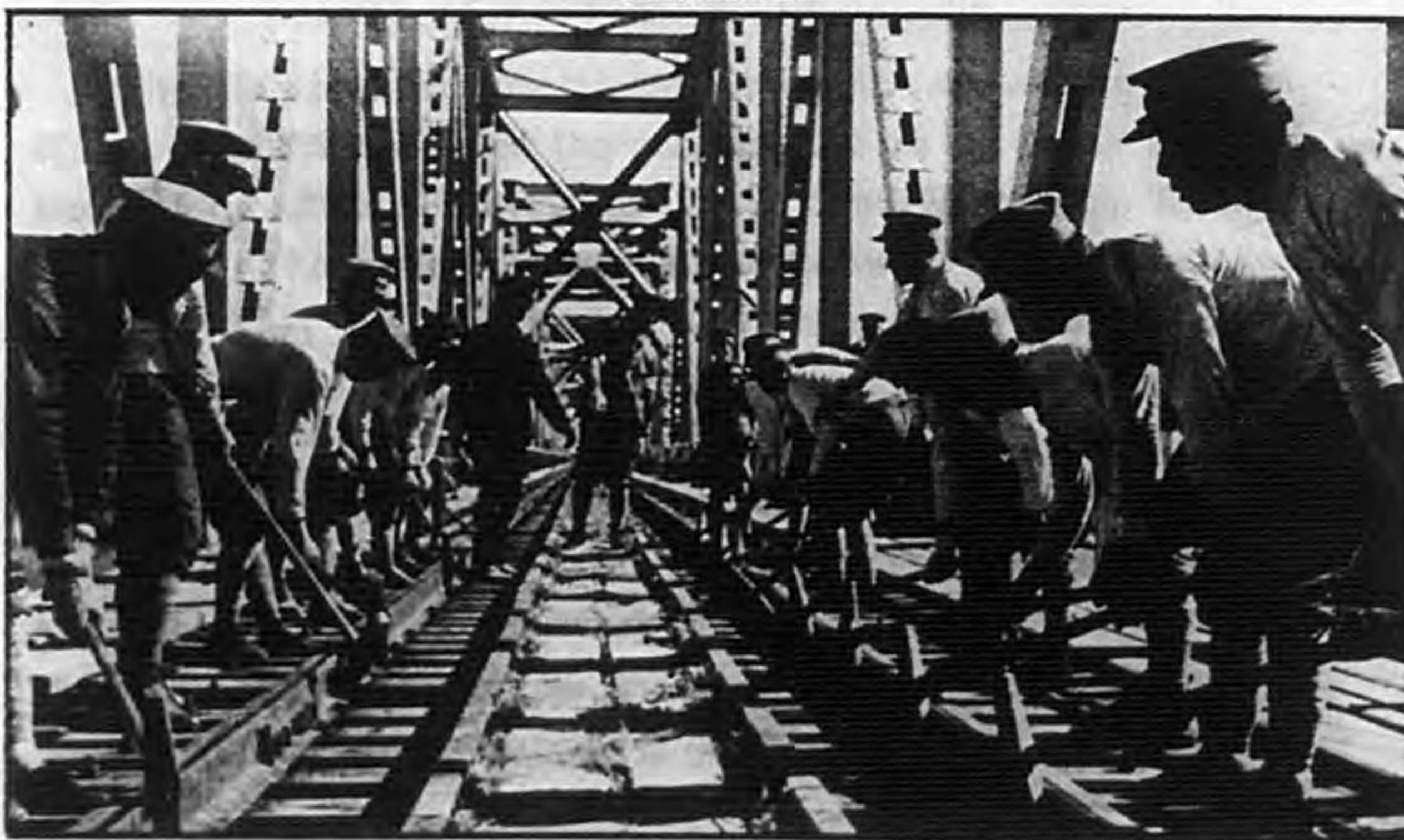
Changing the Gauge of the Hsinking-Harbin Line
