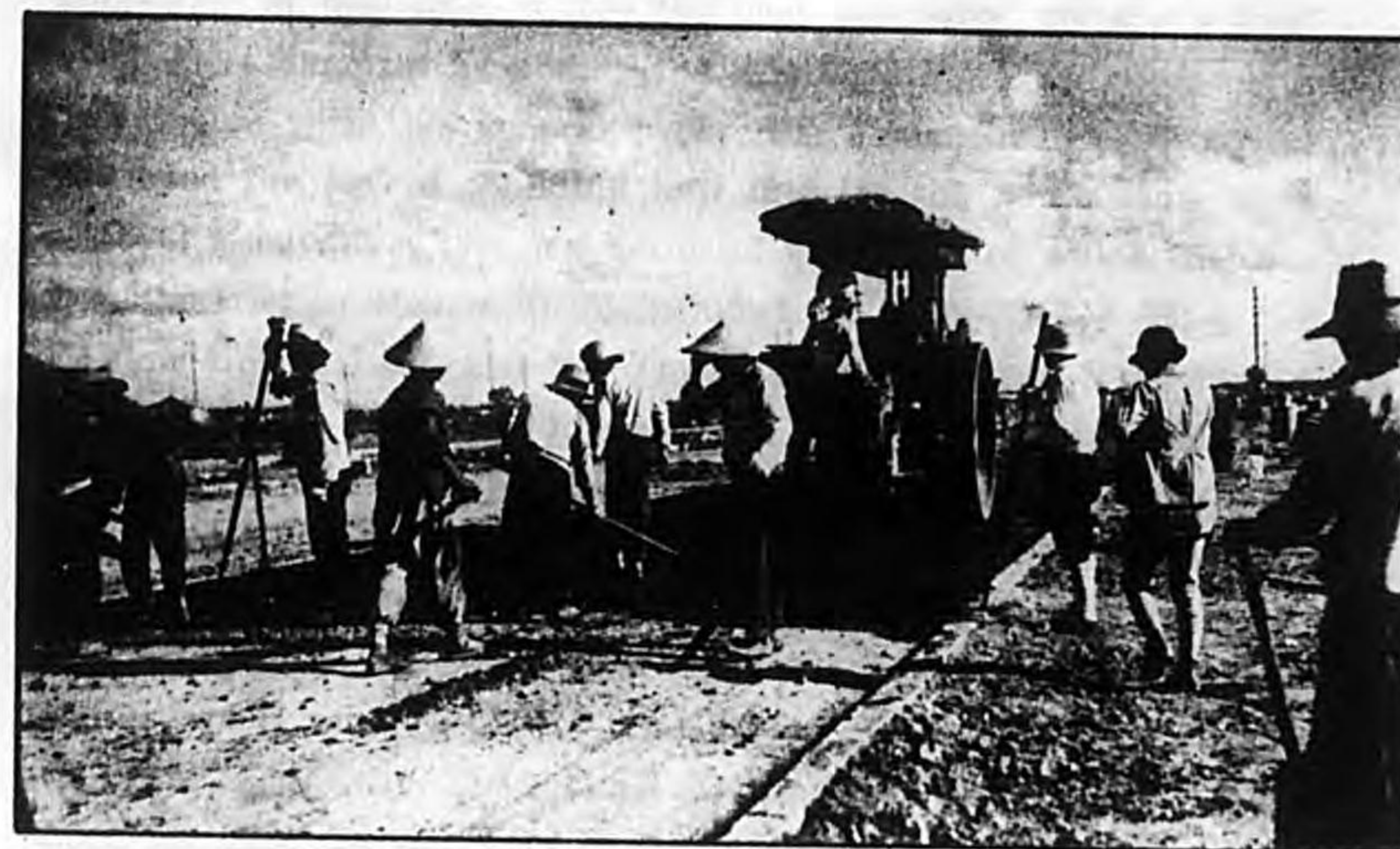
A Scene of the Highway Construction Work
