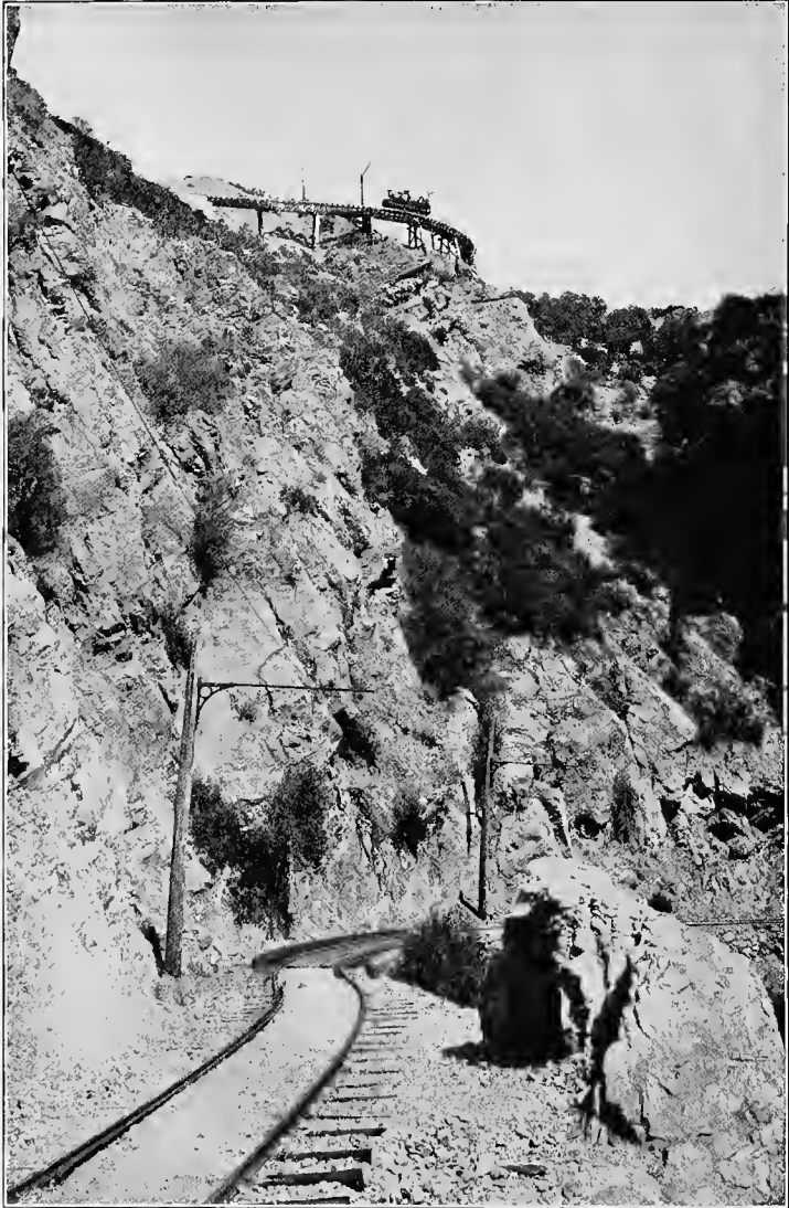
GARDEN OF THE GODS SHOWING "GRAND CIRCULAR BRIDGE"
