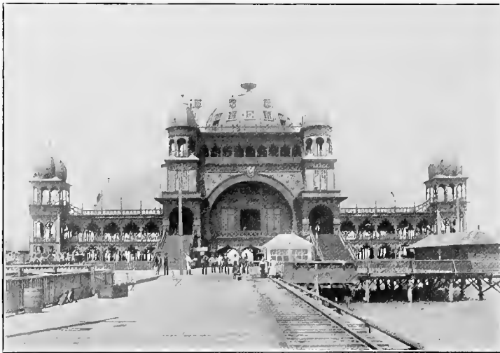
CENTER OF SALT AIR PAVILION, BUILT ON PILING ONE-HALF MILE INTO GREAT SALT LAKE
