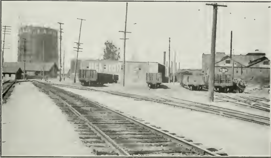
FIG. 164. PACIFIC ELECTRIC TEAM YARD AND TRANSFER YARD
