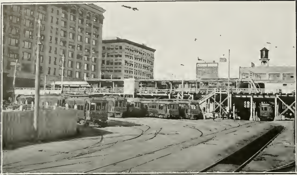
FIG. 88. PACIFIC ELECTRIC YARD AT MAIN STREET STATION
