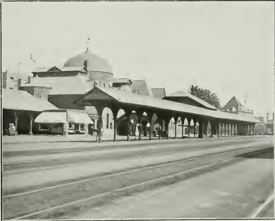
FIG. 85. SANTA FE STATION—REAR VIEW
