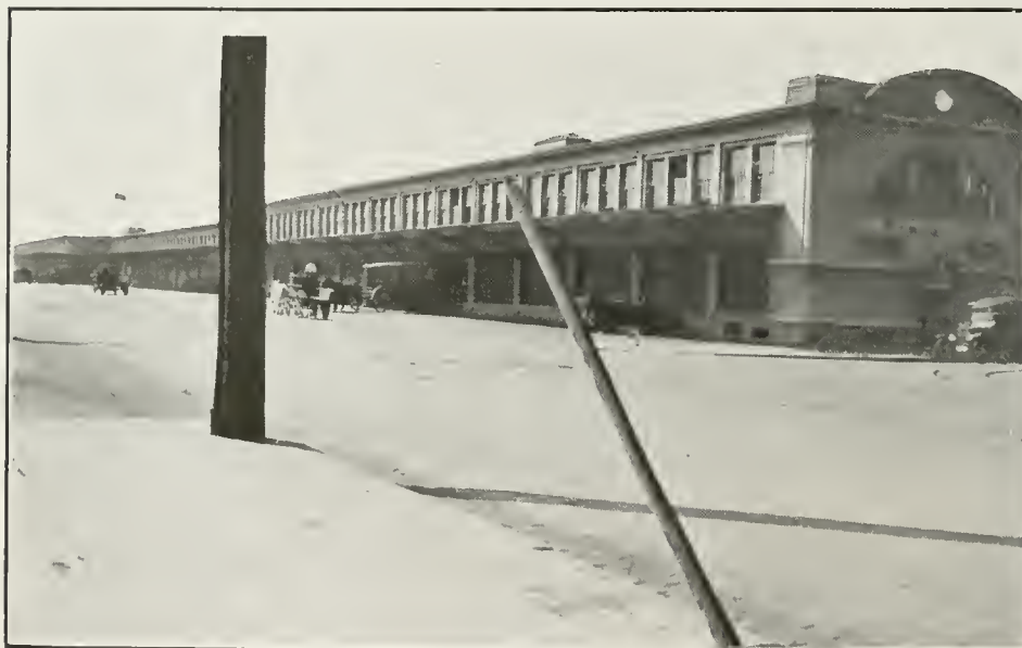
FIG. 150. SANTA FE INBOUND FREIGHT SHED
