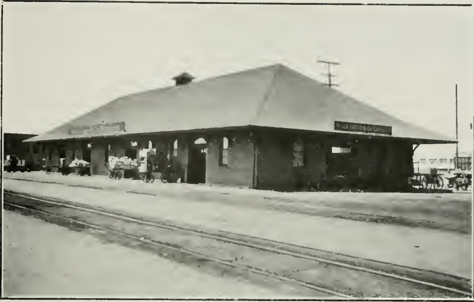
FIG. 97. WELLS FARGO EXPRESS BUILDING—SANTA FE DEPOT
