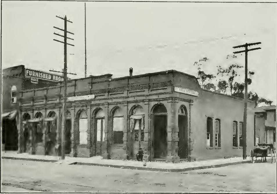
FIG. 83. SOUTHERN PACIFIC RIVER STATION
