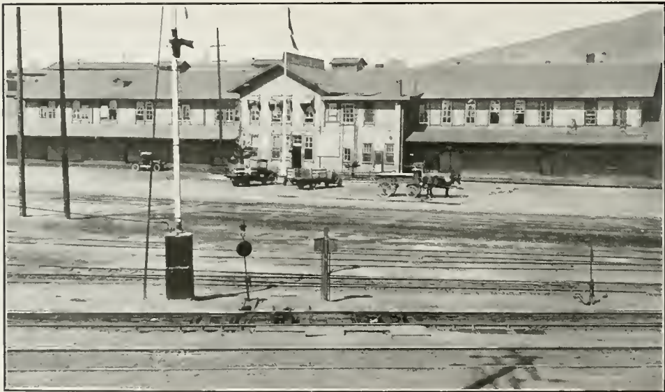
FIG. 147. SOUTHERN PACIFIC FREIGHT DEPOT
