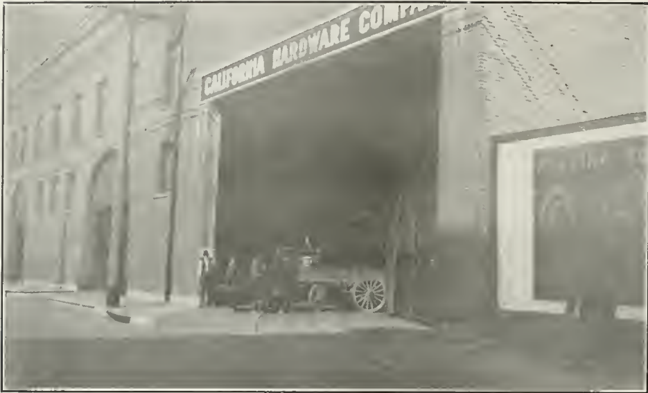
FIG. 171. WAREHOUSE WITH SPUR TRACK INSIDE
