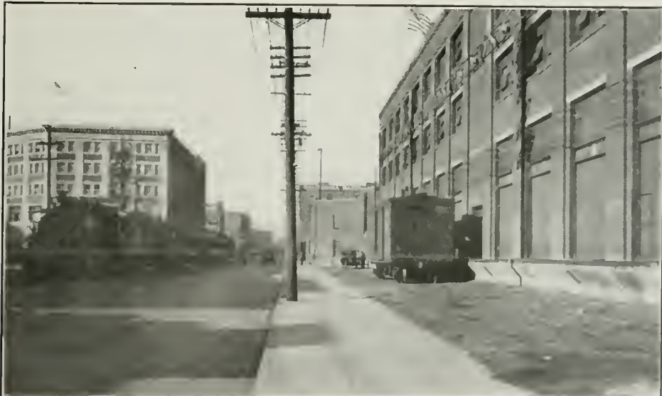
FIG. 170. SPUR TRACK PLACED BEHIND SIDEWALK
