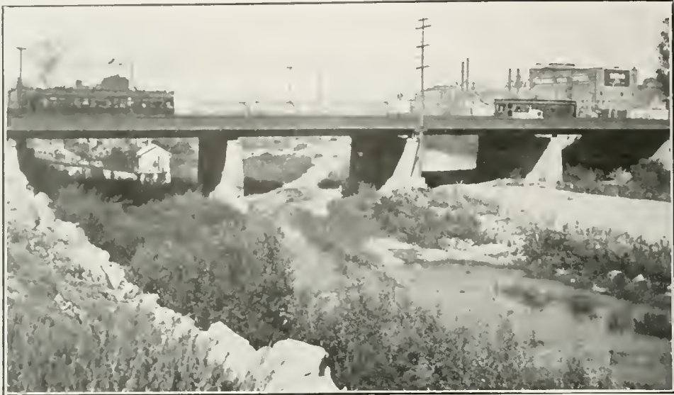
FIG. 42. ALISO STREET BRIDGE ACROSS THE LOS ANGELES RIVER
