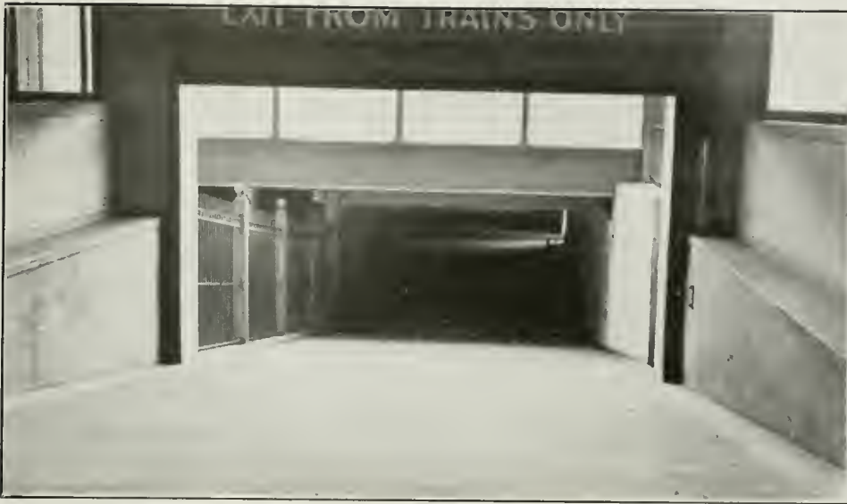
FIG. 81. EXIT SUBWAY AT SOUTHERN PACIFIC STATION
