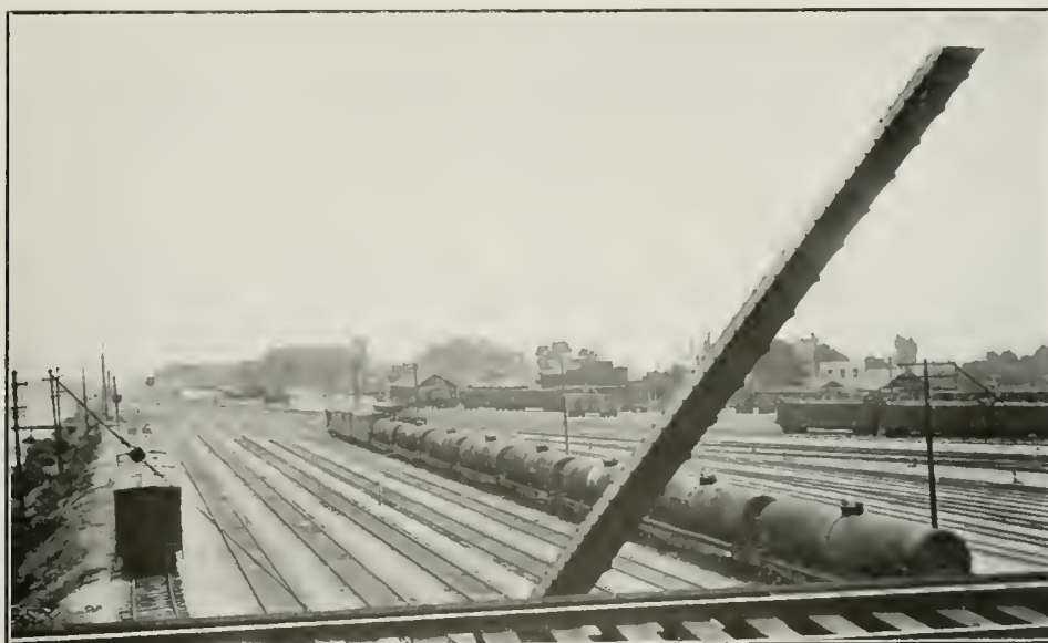
FIG. 142. SOUTHERN END OF SANTA FE FREIGHT YARD
