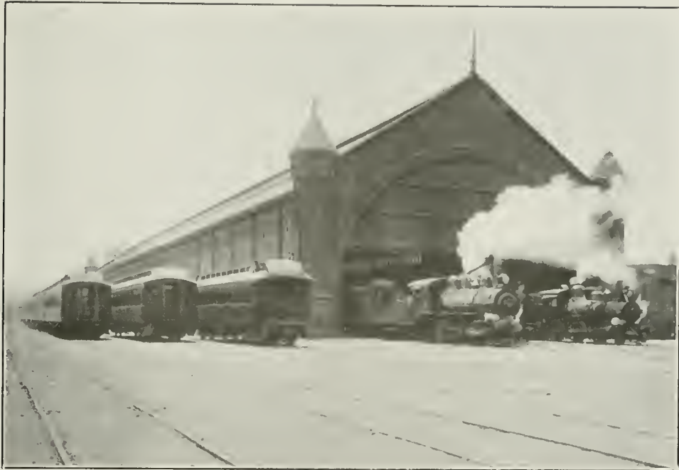
FIG. 9. TRAIN SHED—OLD SOUTHERN PACIFIC ARCADE STATION
