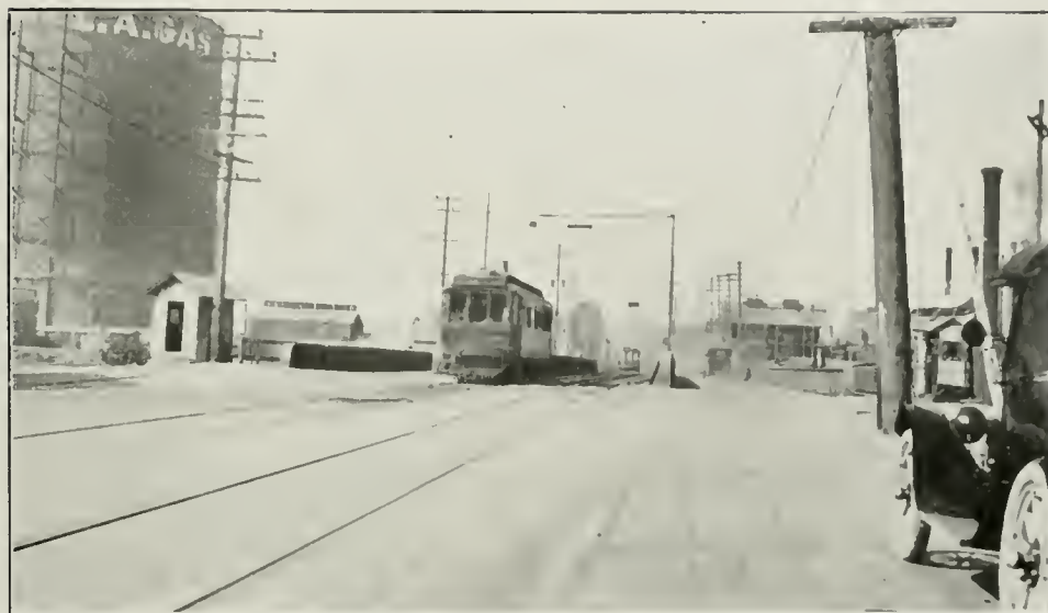
FIG. 33. VIEW LOOKING ALONG ALISO STREET BRIDGE ACROSS THE LOS ANGELES RIVER
