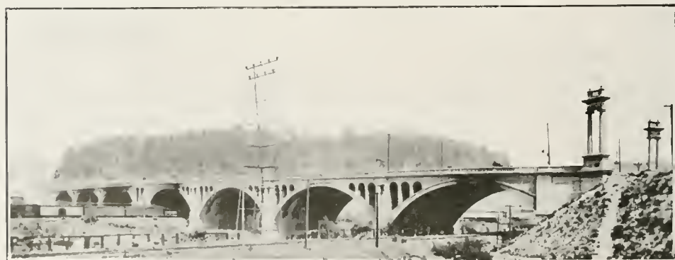
FIG. 31. NORTH BROADWAY BRIDGE
