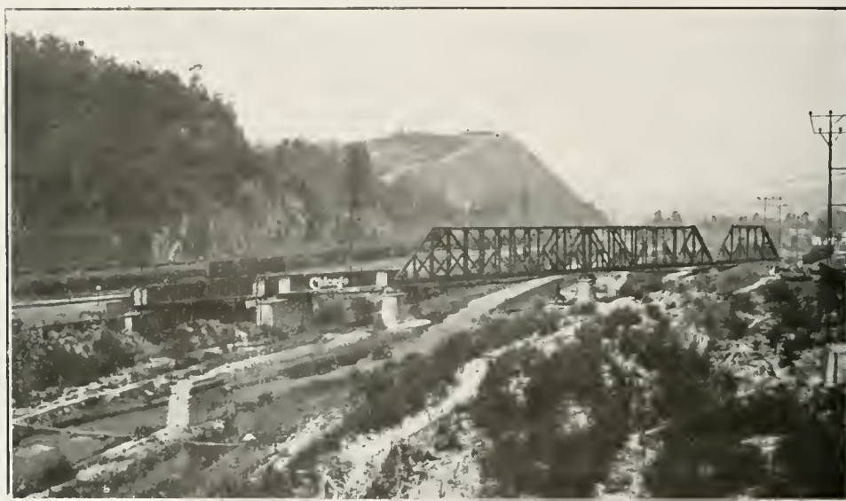
FIG. 30. SANTA FE BRIDGE ACROSS THE LOS ANGELES RIVER
