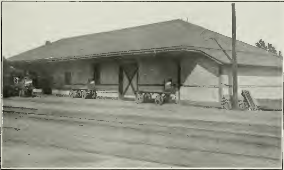
FIG. 98. AMERICAN EXPRESS COMPANY—SALT LAKE STATION
