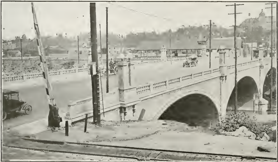
FIG. 55. ANOTHER VIEW OF SEVENTH STREET BRIDGE ACROSS LOS ANGELES RIVER
