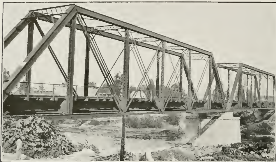
FIG. 61. SANTA FE BRIDGE ACROSS LOS ANGELES RIVER SOUTH OF BUTTE STREET This is a single track, steel structure, built in 1897, and carries the Santa Fe's main line to San Diego and San Bernardino, via Fullerton.
