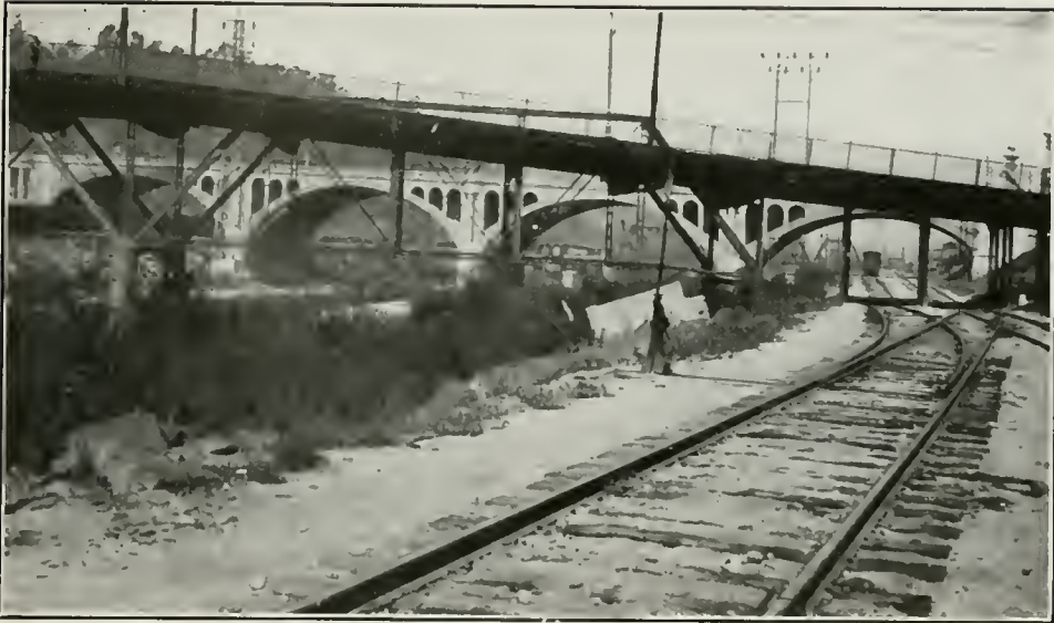
FIG. 33. NORTH END OF NORTH SPRING STREET BRIDGE
