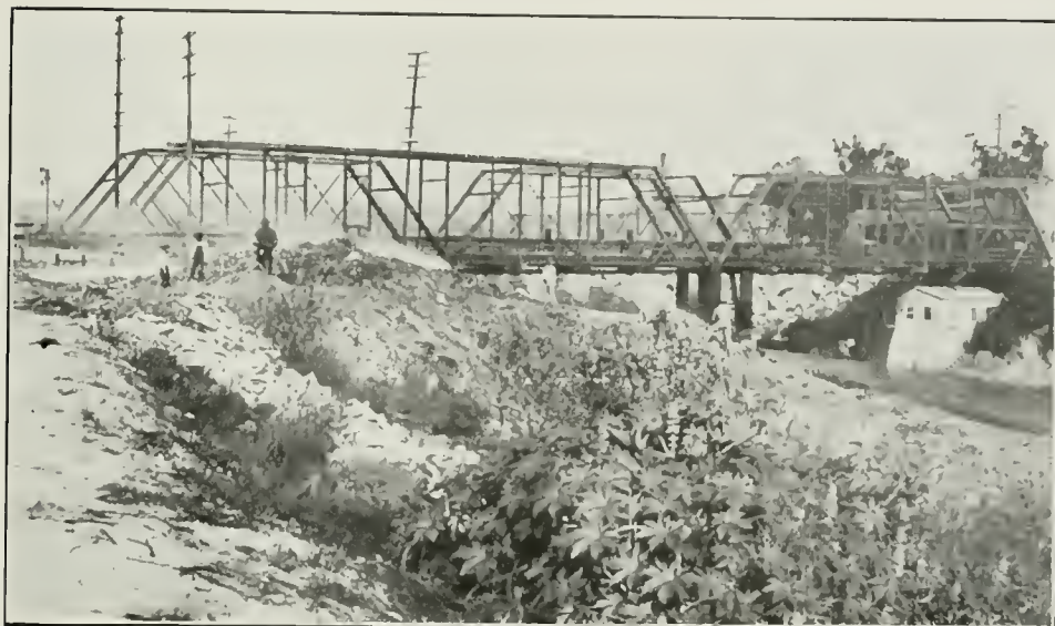
FIG. 39. BRIDGES ACROSS LOS ANGELES RIVER AT MACY STREET
