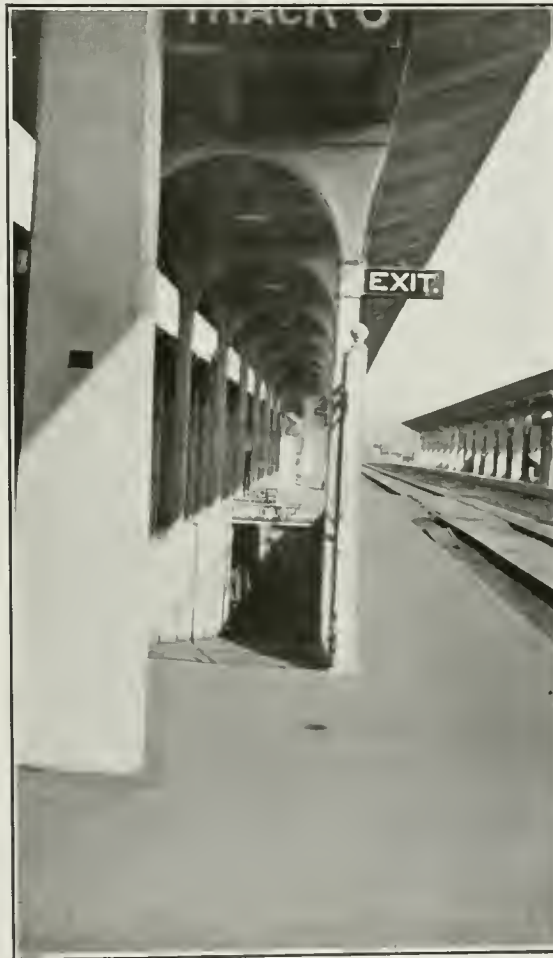
FIG. 79. PLATFORMS AND SIDE SUBWAYS AT SOUTHERN PACIFIC STATION
