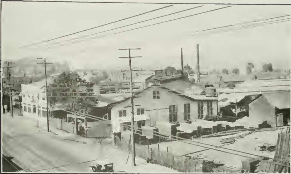
FIG. 196. IMPROVEMENTS UPON THE PROPERTY OF THE OIL WELL SUPPLY COMPANY
