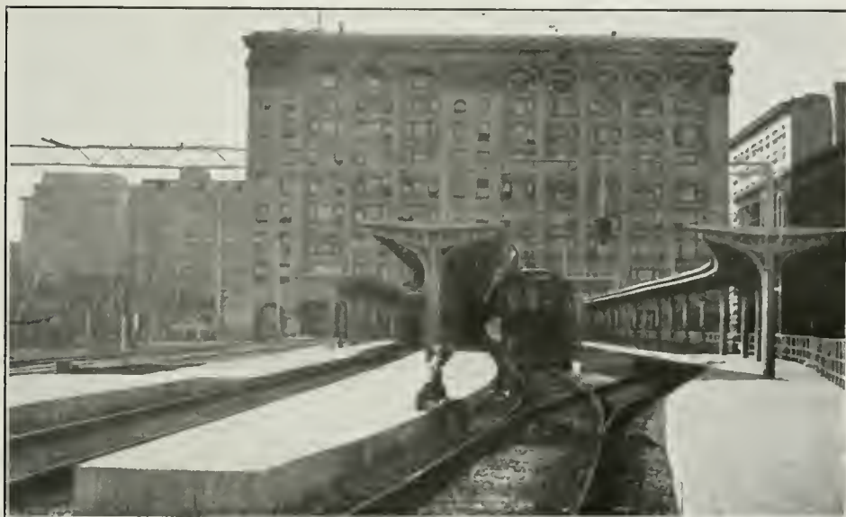
FIG. 87. PACIFIC ELECTRIC BUILDING—REAR VIEW
