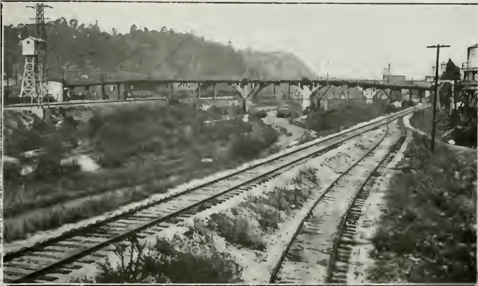
FIG. 32. NORTH SPRING STREET BRIDGE CROSSING THE TRACKS OF THE SANTA FE, THE LOS ANGELES RIVER AND THE TRACKS OF THE SALT LAKE
