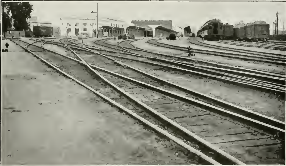
FIG. 82. SOUTHERN PACIFIC STATION YARD—SOUTH END
