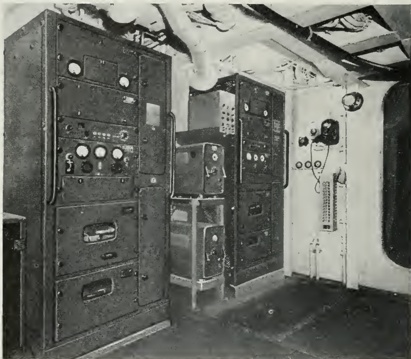
Fig. 37—Radars Mark 3 & 4—main units on Battleship New Jersey (Navy Photo 181809)
