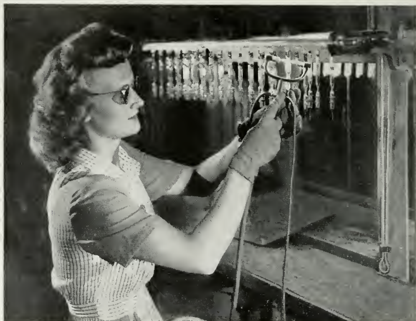
Fig. 35—Pump Station for the 724B Vacuum Tube
