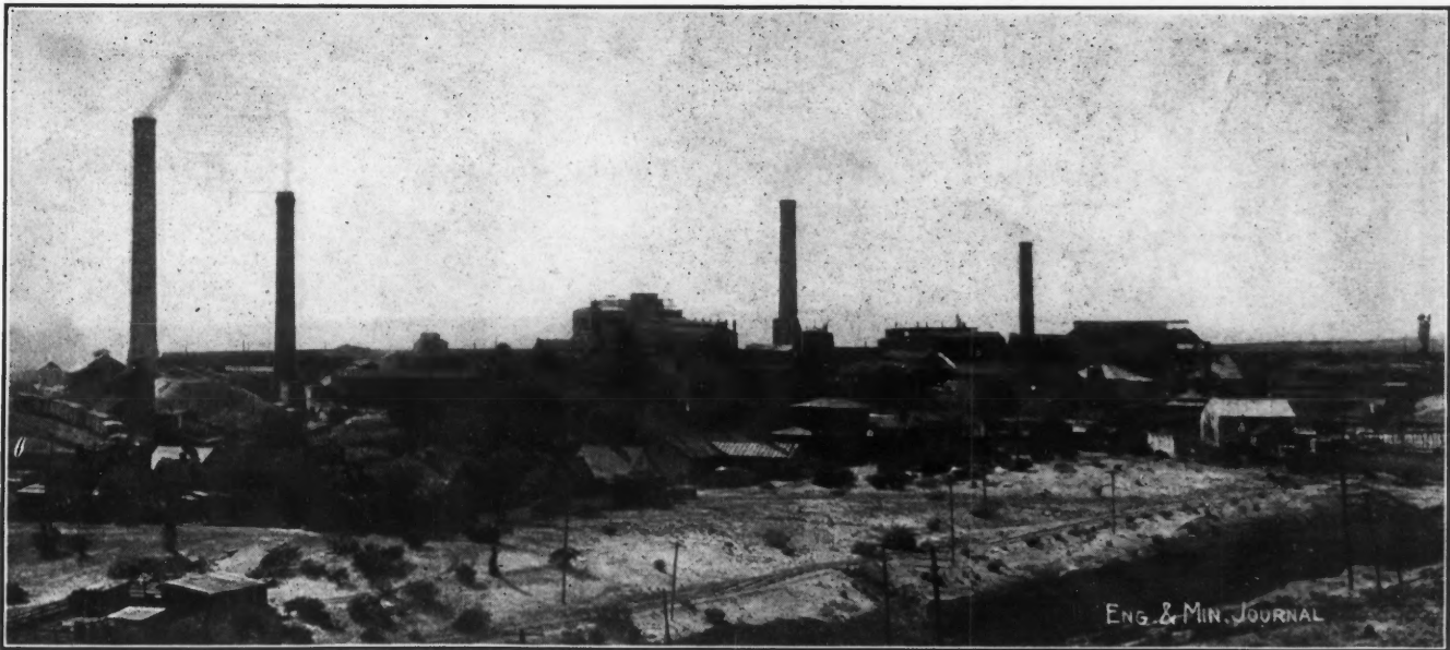
GENERAL VIEW OF EL PASO SMELTING WORKS, EL PASO, TEXAS
