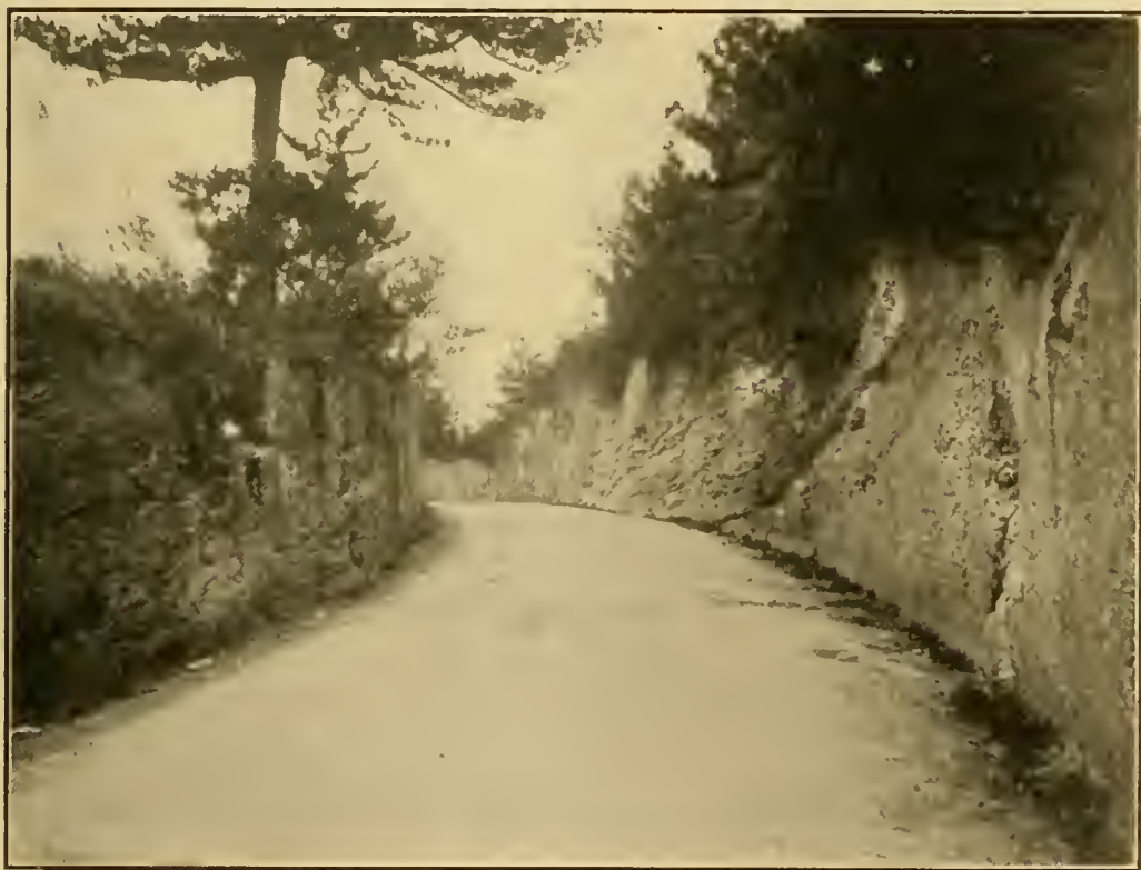
Figure 12.—Road Cutting near Hamilton.
