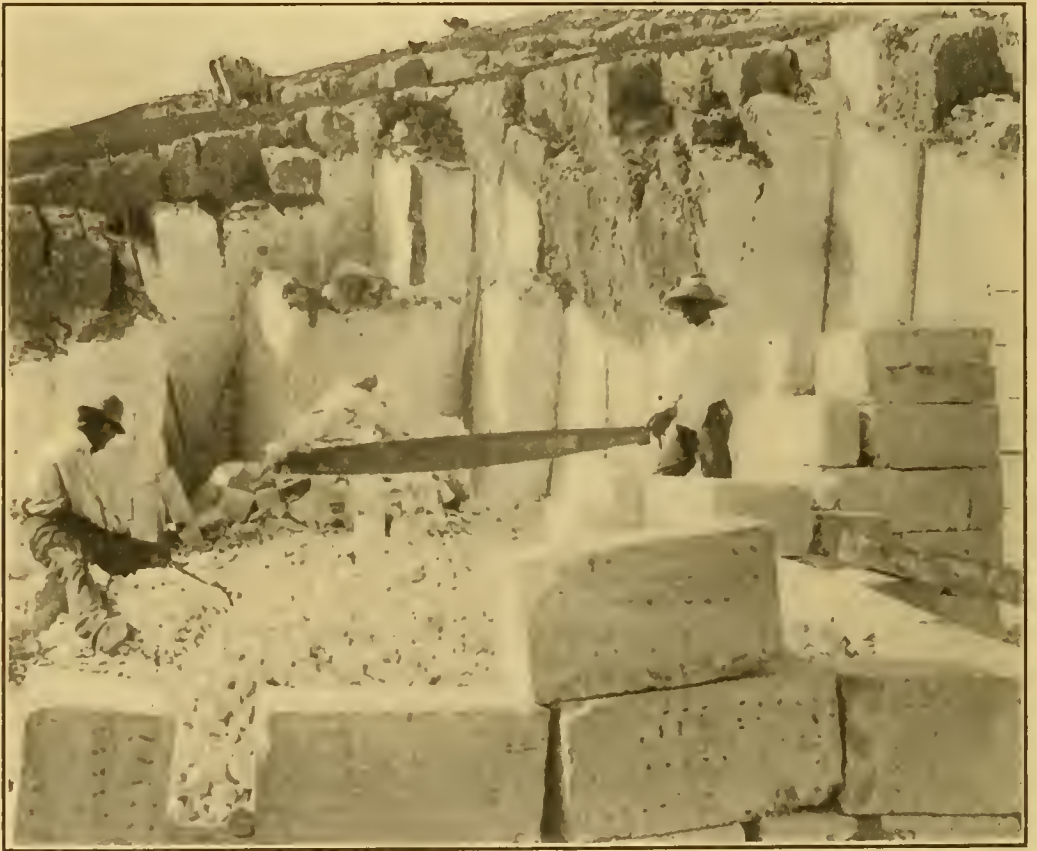
Figure 11.—Quarrying Limestone with chisels and saws.
