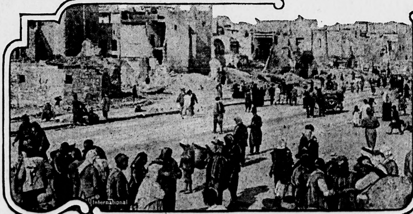
Allenby street, Beirut, Syria, showing houses destroyed. This street is one of the most interesting thoroughfares in the world, being a product of the war and of German "efficiency." Needing a good highway from the waterfront to their barracks, the Germans destroyed the major part of the residential district in building it. When the British finally occupied the port their first act was to name this roadway "Allenby street" in honor of their famous commander.
