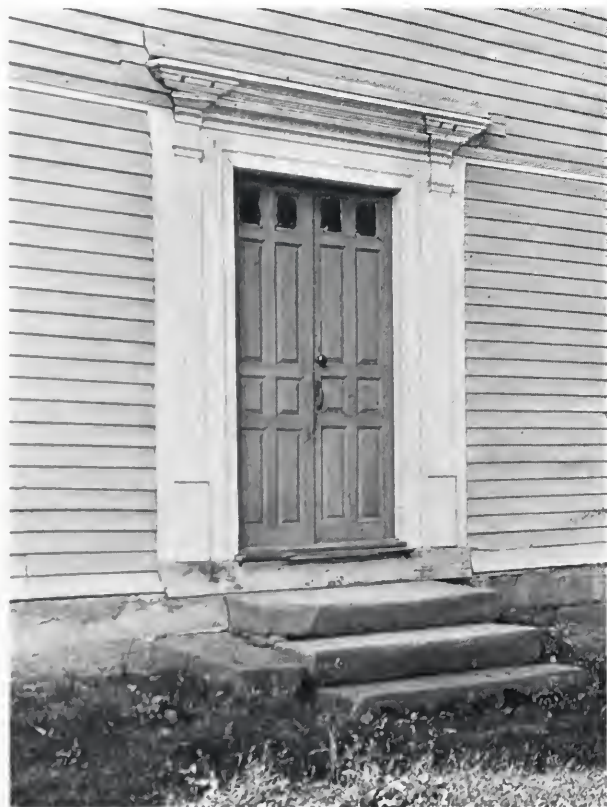
DETAIL OF DOORWAY FARMHOUSE, ROCKY HILL, CONNECTICUT
