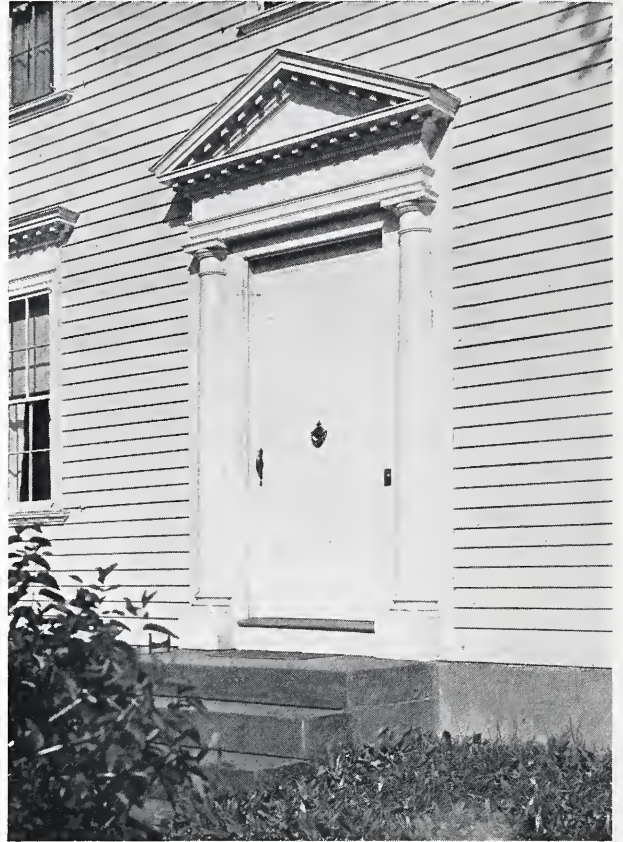
DETAIL OF DOORWAY HOUSE AT WINDSOR, CONNECTICUT
