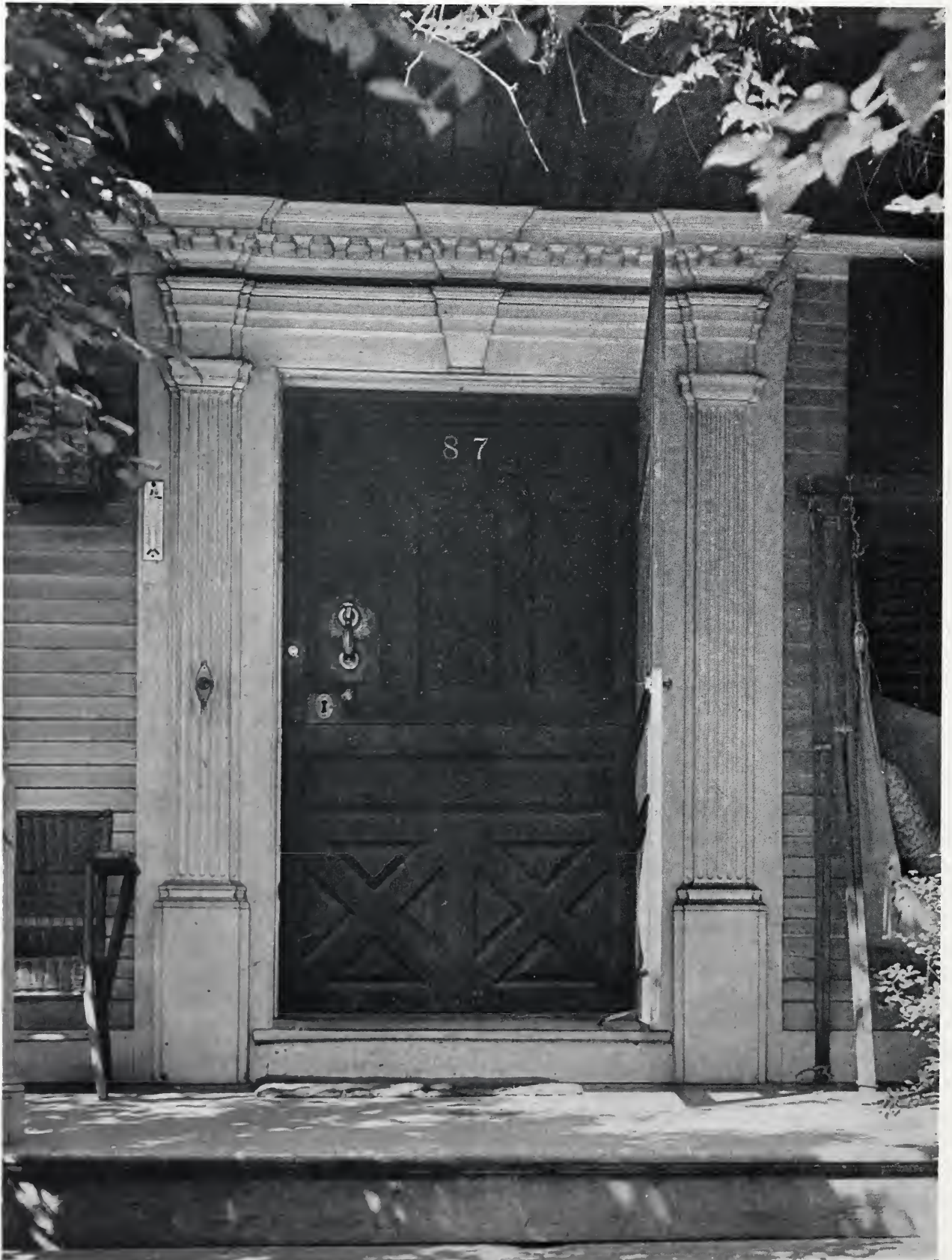
DETAIL OF DOORWAY SILAS DEANE HOUSE, WETHERSFIELD, CONNECTICUT
