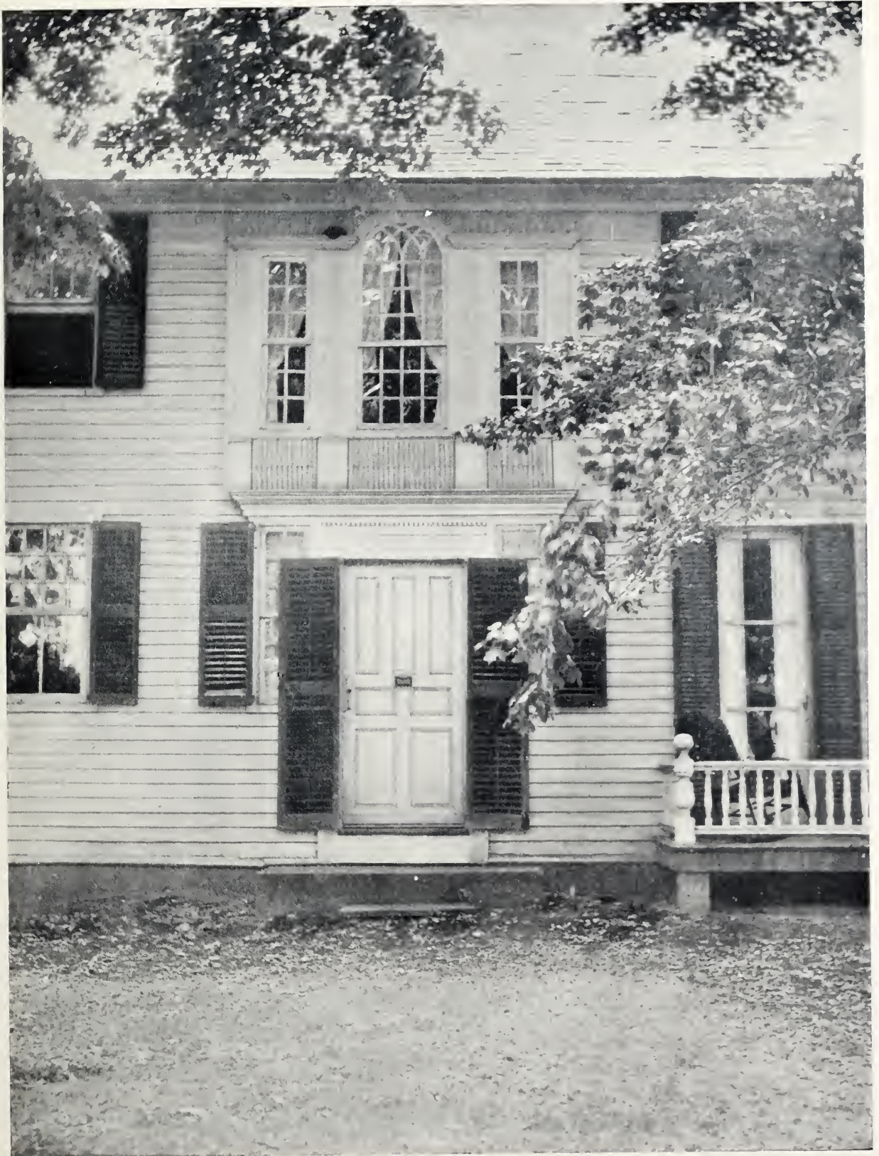
THE ABIJAH CATLIN HOMESTEAD, HARWINTON, CONNECTICUT Built in 1795. It has all the motives which are distinctly of Connecticut origin
