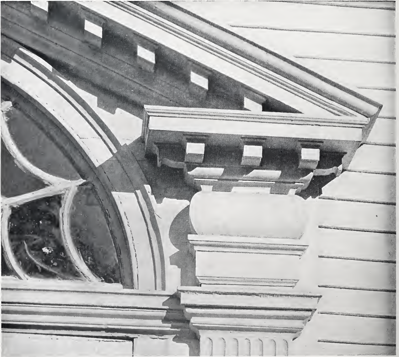
Detail of Main Doorway
