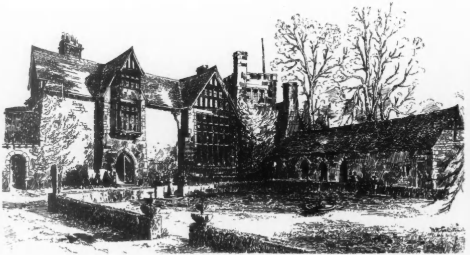
1488. Little Missenden Abbey, Bucks, View from Courtyard , W. HOWARD SETH-SMITH, F.R.I.B.A., Architect.
