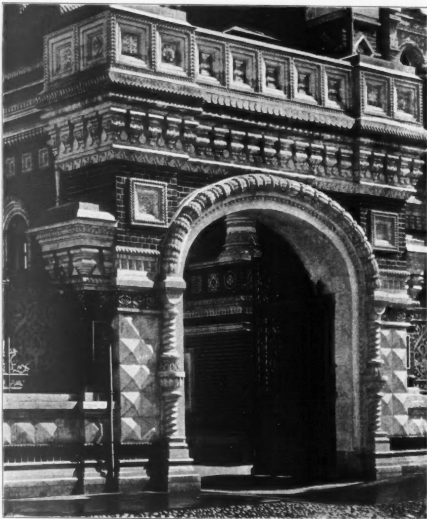
Palais Igumnoff, Moskau, THE LATE N. I. POSDEFF, Architect.
