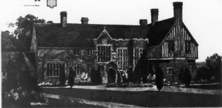
1506. House at Oxted, Entrance Front , R. A. BRIGGS, F.R.I.B.A., Architect.
