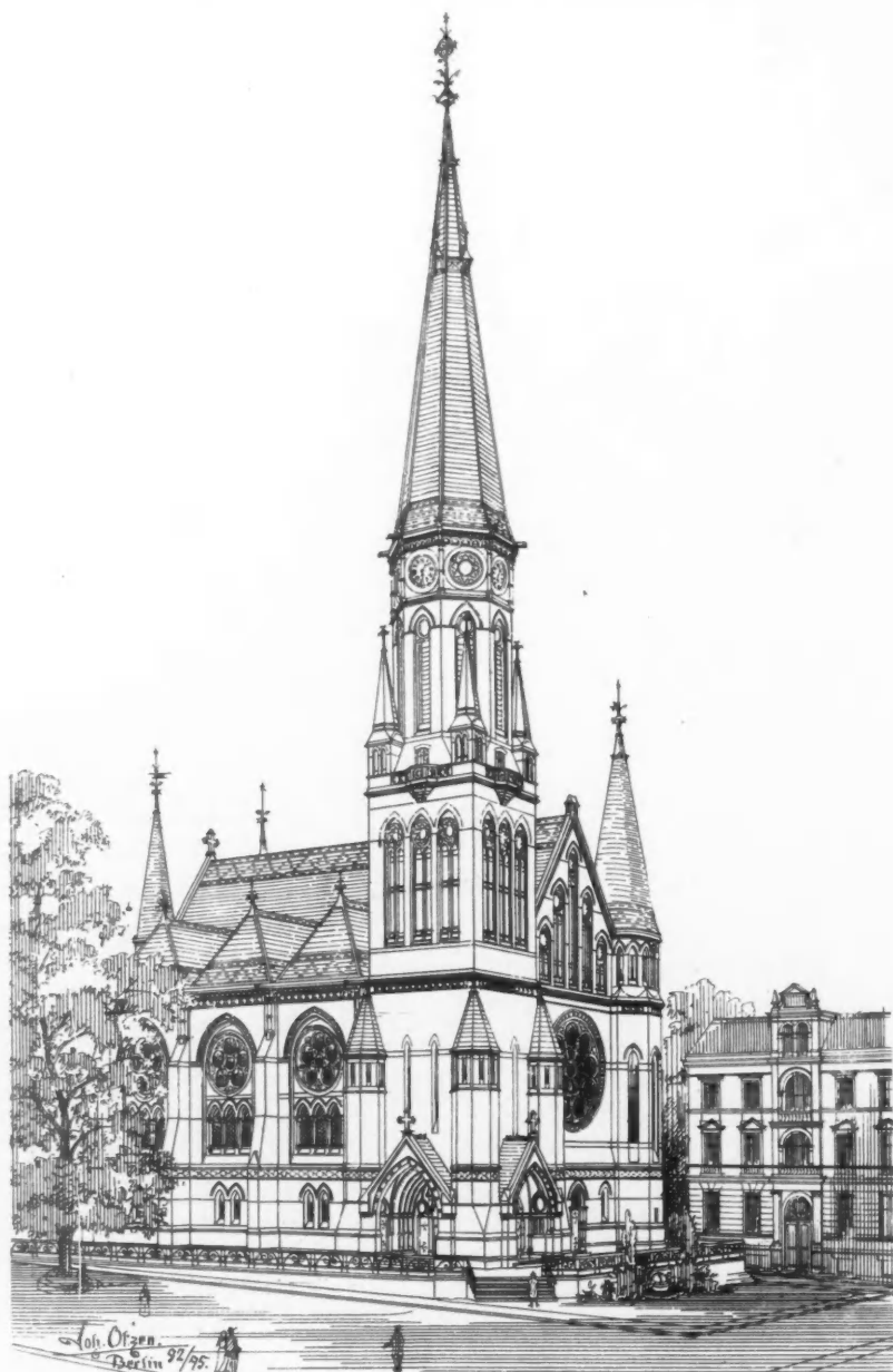
Church at Apolda, PROFESSOR JOHANNES OTZEN, Architect, Berlin. (For Plan, see p. 64.)
