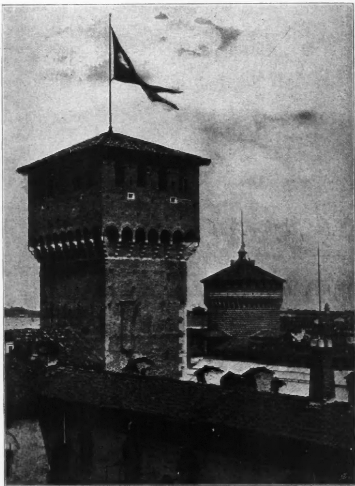
Restoration of the Round Tower, erected at Milan, A.D. 1456, pulled down to ridge of adjoining Roofs in the year 1848, and rebuilt 1893-94, to contain Water Supply for the Town of Milan, LUCA BELTRAMI, Architect.
