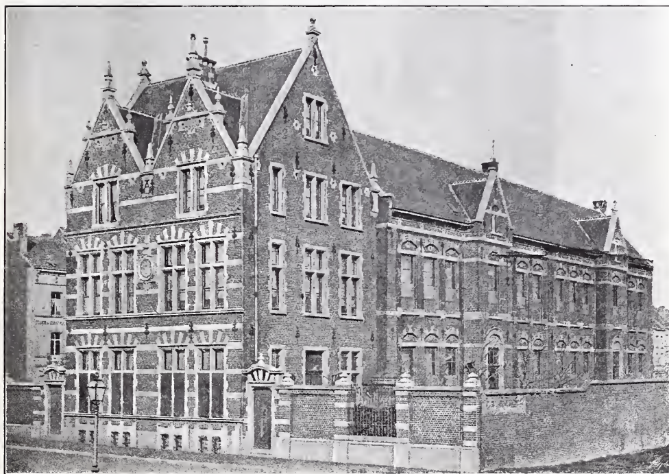
Schools, Avenue de Birmingham, Anderlecht, near Brussels, J. J. VAN YSENDYCK, Hon. Corresponding Member R.I.B.A. Architect, Brussels. (For plan see p. 145.)
