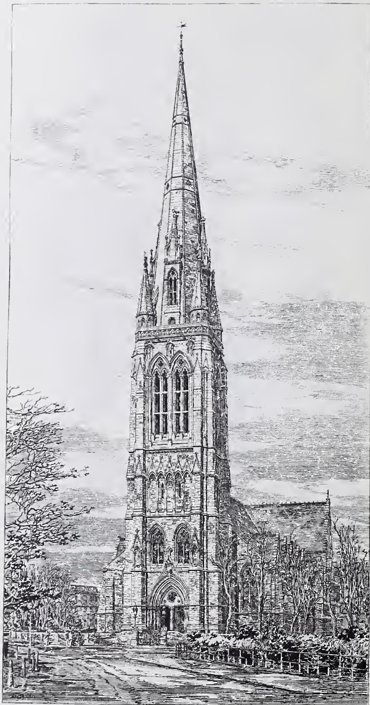
1821. St. Mary's, Stoke Newington, Tower and Spire , J. OLDRID SCOTT, F.R.I.B.A., Architect.
