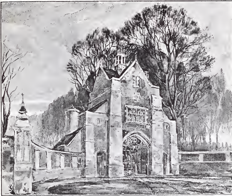
Entrance Lodge at Welbeck Abbey, for his Grace the Duke of Portland, H. WILSON, Architect.
