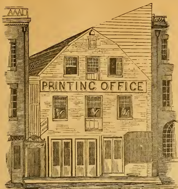
THE OLD GABLE HALL.
