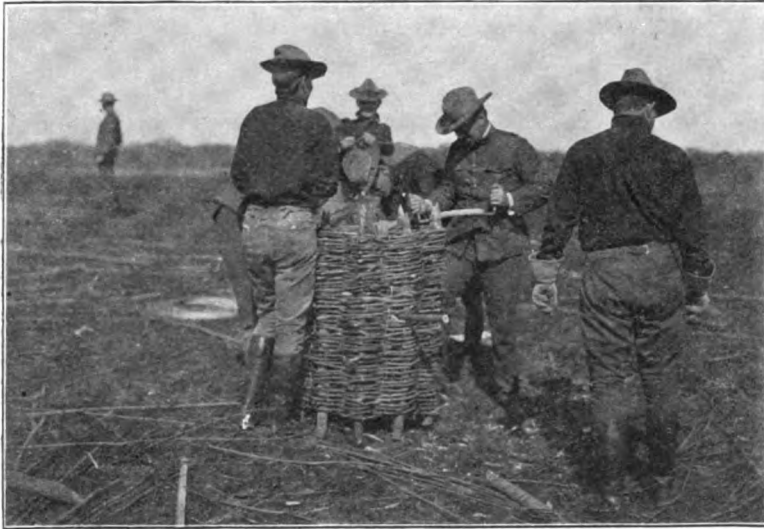
CONSTRUCTING GABION.
