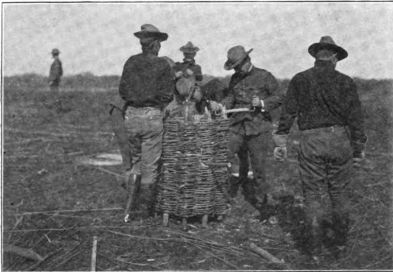
CONSTRUCTING GABION.
