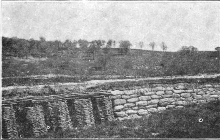
GABION AND SAND BAG REVETMENT.
