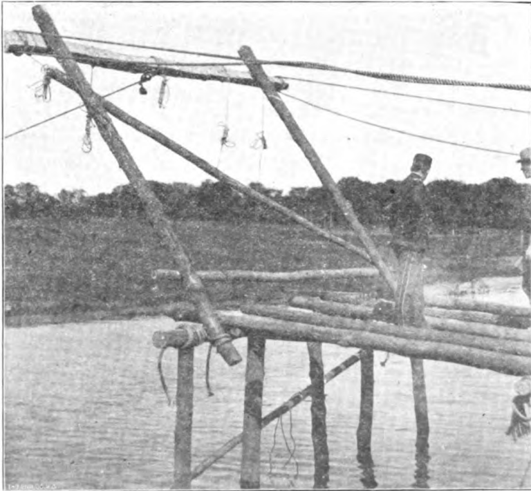
REES' PILE BRIDGE. FIRST POSITION NEW BAY.
