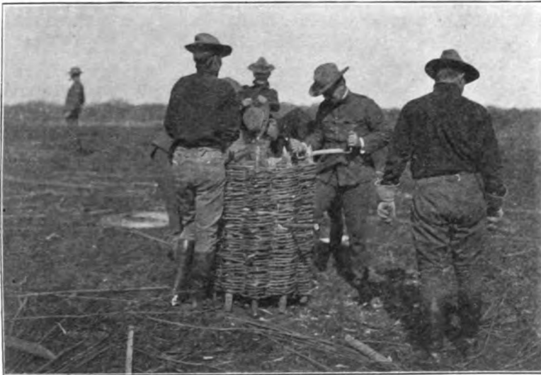
CONSTRUCTING GABION.
