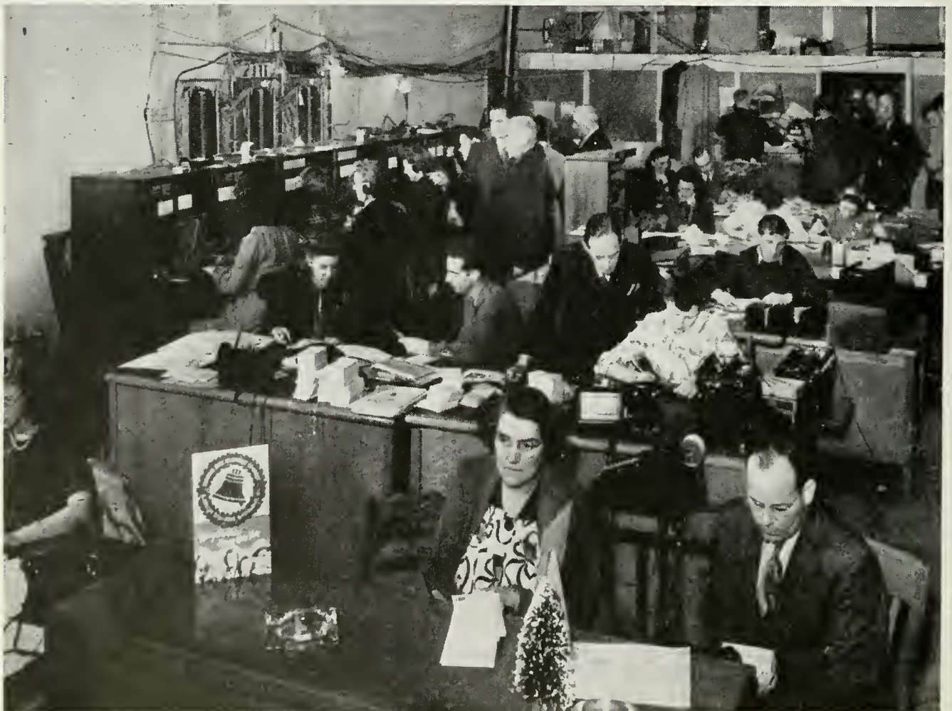
Eight positions of PBX switchboard turn the telephone business office, a block from the destroyed central office, into a temporary operating room
