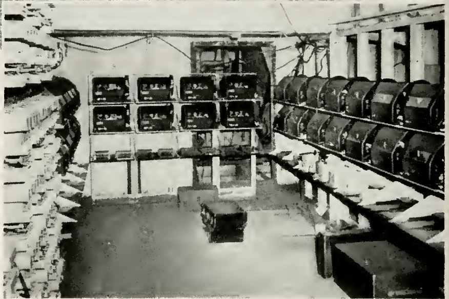
"Sigcircus" afloat: the Signal Corps' complete "Seaborne Communications Center" used in the Pacific. Right: Teletypewriter equipment installed in one of the barges
