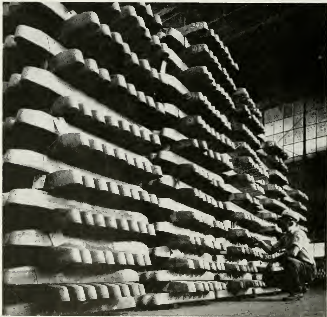
Reclaimed, refined, and molded into wire bars, copper by the ton at Nassau awaits shipment to Western Electric, where it will be drawn into copper wire
