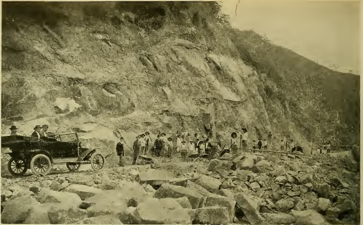
Carretera del Norte—Northern Wagon Road
