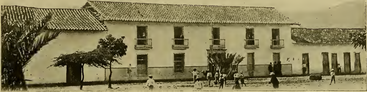
Casa de Gobierno—Government Building—Zapatoca
