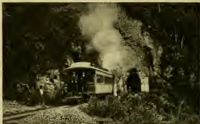
Entrada al túnel, Ferrocarril de Girardot—Entrance to tunnel, Girardot Railroad
