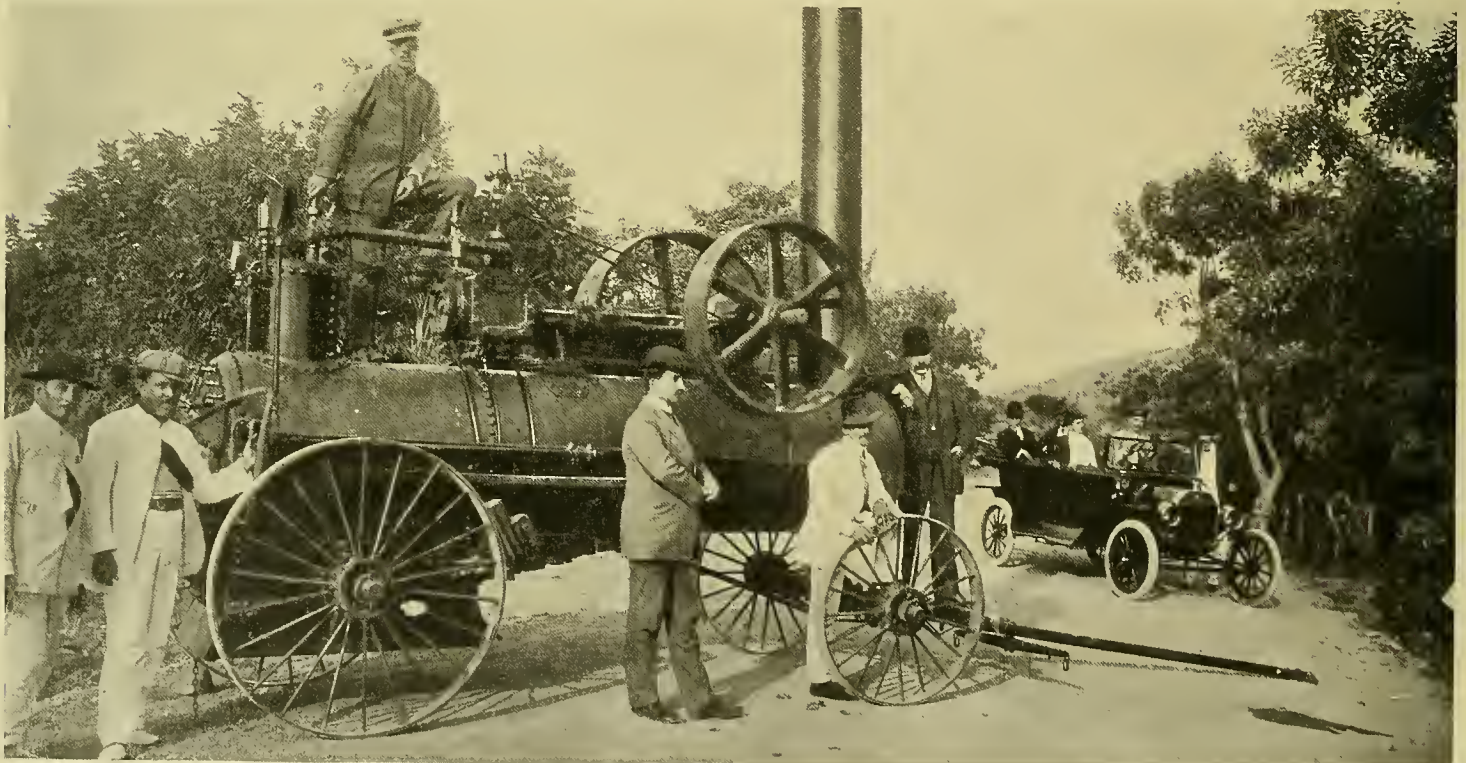
Maquinaria de la Carretera—Wagon-Road Machinery
