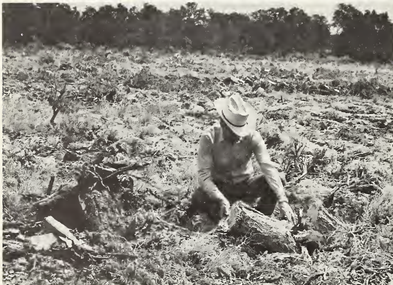
Figure 17.—The 83-ton tree crusher (top) uproots and crushes the trees in one operation. Pieces of trees left on the ground (left) are the right size for fireplaces.
