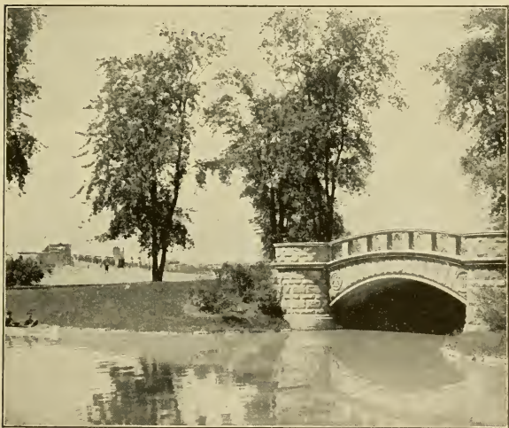
Entrance to Belle Isle from the Bridge.
