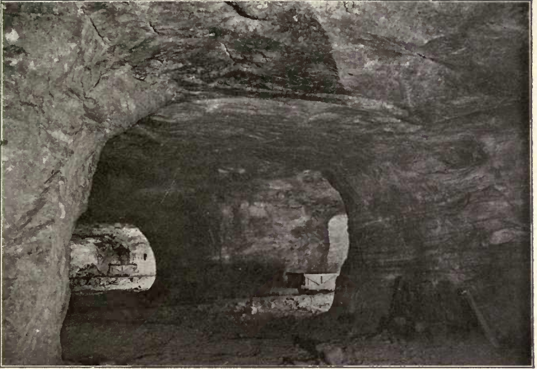
FIG. 1. — Interior view of salt mine, Livonia, N. Y. Both roof and pillar are rock salt.
