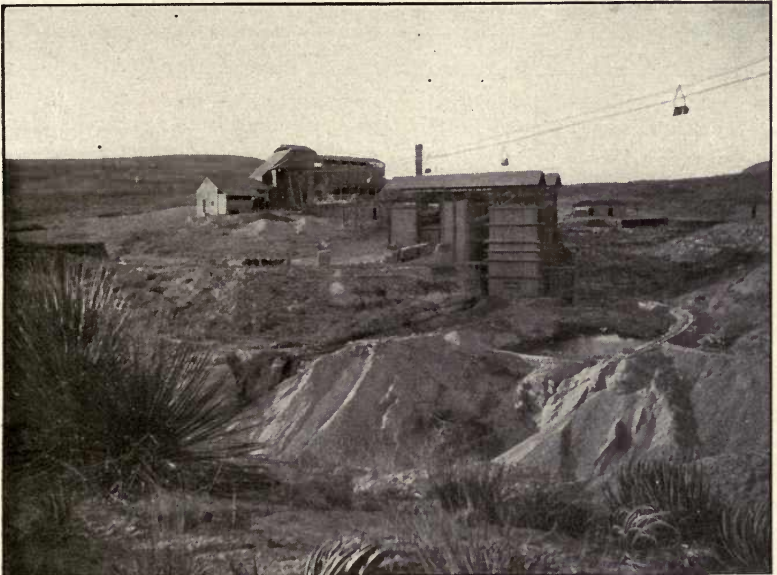
FIG. 2. — Furnace for roasting mercury ore, Terlingua, Tex. ( H. W. Turner, photo. )
