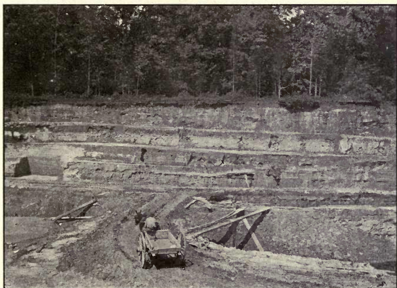
FIG. 2.—Bank of sedimentary clay, Woodbridge, N. J. This section affords at least five kinds of clay. (Photo., H. Ries.)
