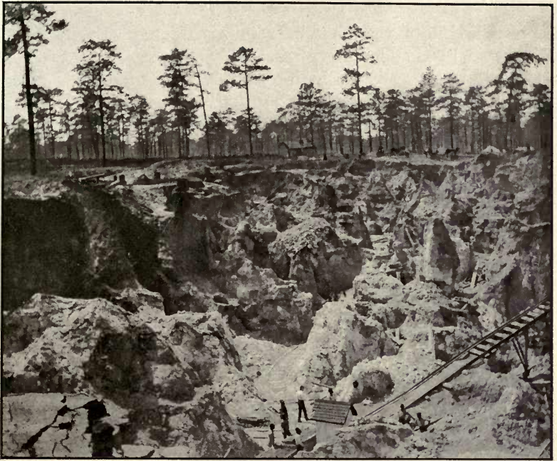
FIG. 1.—Rock phosphate mine near Ocala, Fla. (Photo., A. W. Sheaffer.)
