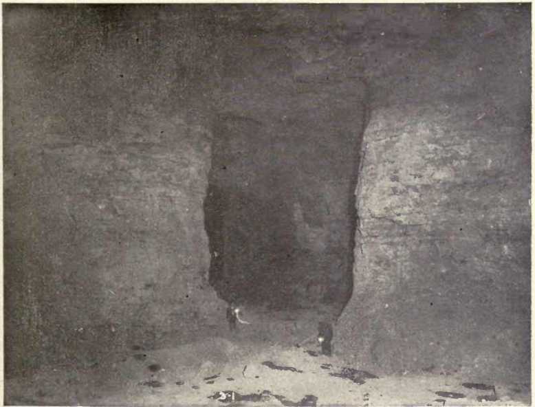
FIG. 2. — Chambers in Disbrow Mine, near Webb City, Mo. These include both sheet ground and the "broken ground" above. (Photo from F. C. Wallower.)
