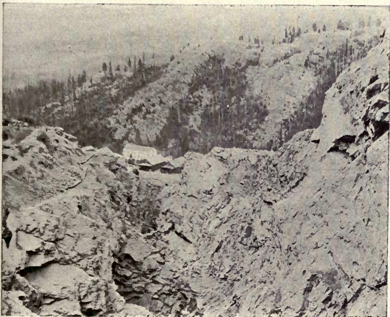
FIG. 2.—Open cut, Mother Lode mine, near Greenwood, Brit. Col. Right wall, limestone; left wall, contact metamorphosed rock. ( H. Ries, photo. )
