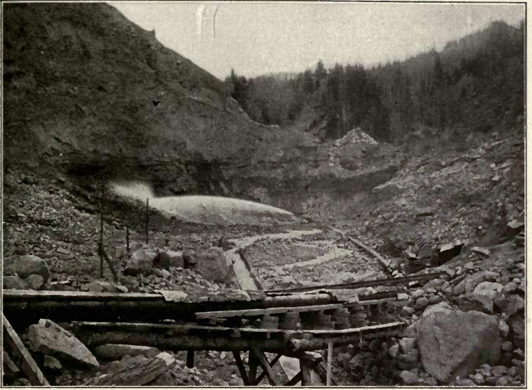
FIG. 1. — Hydraulic mining of auriferous gravel. The sluice box in foreground is for catching the gold.
