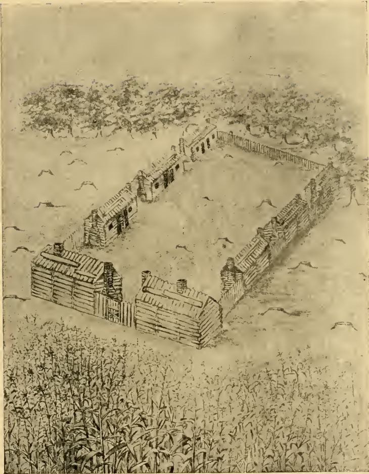
BLOCKHOUSE AND LOG CABINS ON CORN ISLAND, 1778.
