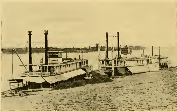
LITTLE ROCK LEVEE.
