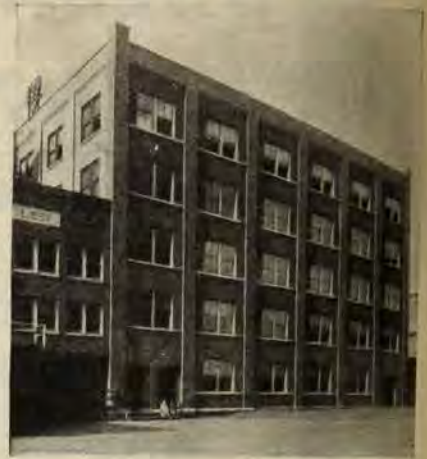
Libby, McNeil & Libby Bldg., Chicago, P. Larnon, Archt. Kahn System Reinforced Concrete
