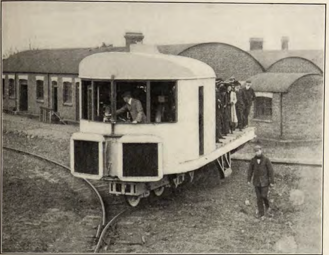
FRONT VIEW OF THE BRENNAN MONO-RAIL CAR
