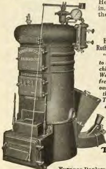
This illustration shows the Underfeed Boiler.
