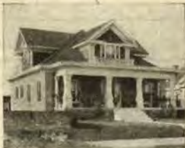
A No. 1-22-W IDEAL Boiler and 422 ft. of 38-in. AMERICAN Radiators, costing the owner $195, were used to Hot-Water heat this cottage.
