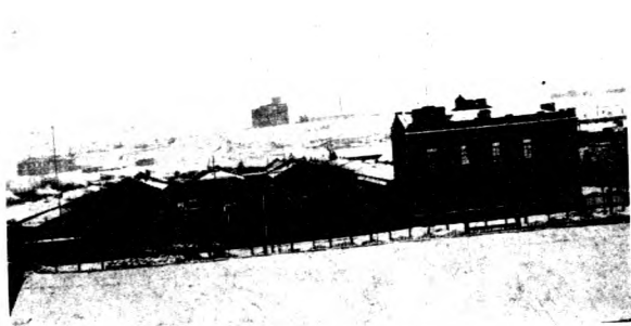
HARBIN HOSPITAL West (administrative) compound containing also general hospital. 哈爾濱醫院 表示靠西辦事大院與總醫院圖
