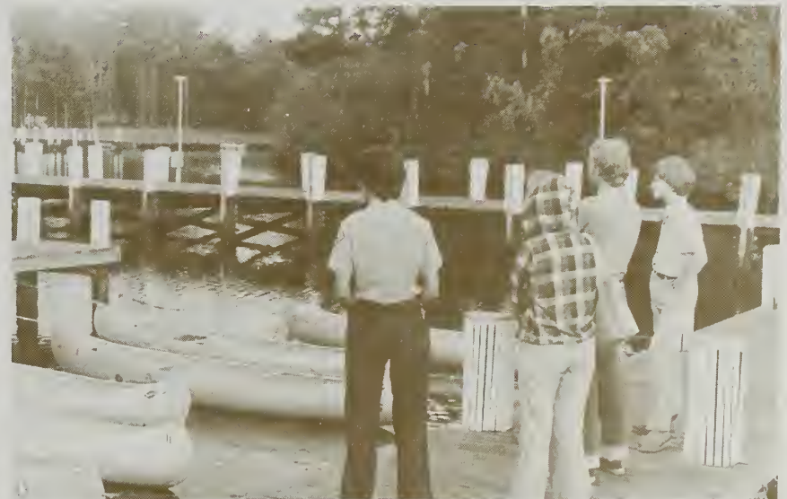
Boat docks in Pocomoke State Park, Shad Landing Area.
